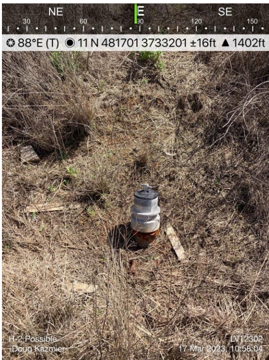
Photo 6: View of modern irrigation riser (View E)
