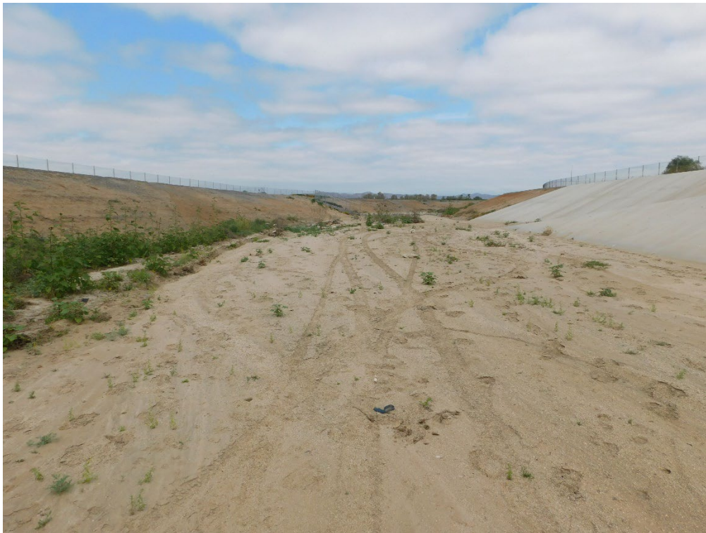
Photograph 8: From the middle of the flood control channel looking southeast.
