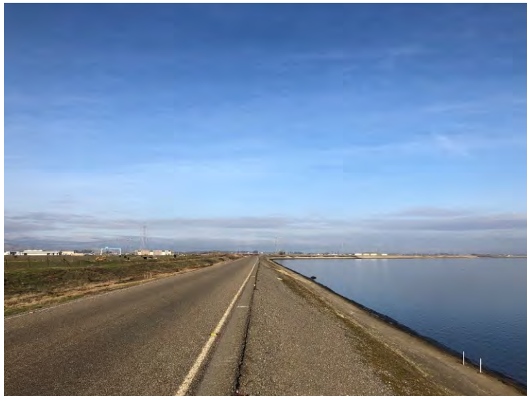
Figure 3. Clifton Court Forebay, looking west towards California Aqueduct intake channel (IMG_3800)
