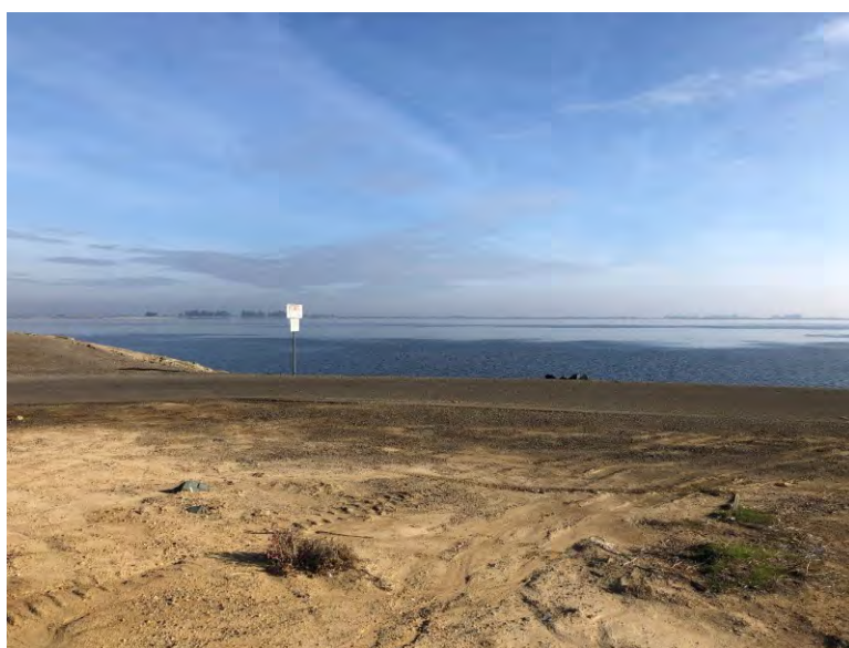
Figure 9. Clifton Court forebay, looking northeast (IMG_3786)
