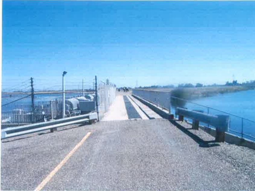
Photograph 7. Bridge, camera facing northeast
