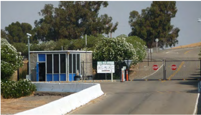
Photograph 20. Banks Plant Building 11. View to northwest.
