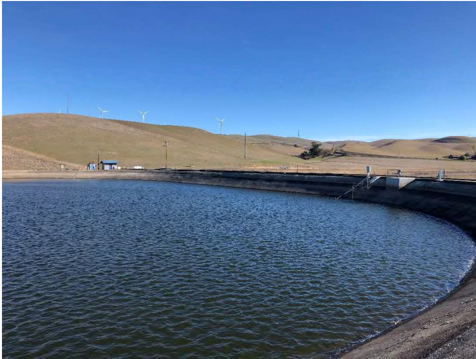
Figure 6. Patterson Reservoir, view looking southeast (IMG_4146)
