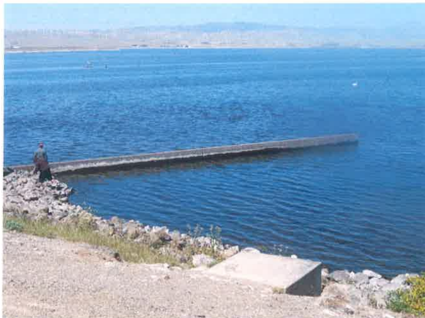
Photograph 6. Concrete wing walls, camera facing southwest
