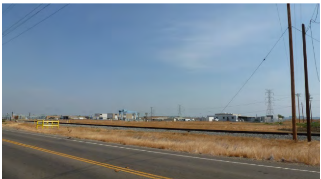
Photograph 8. Overview of Skinner Fish Facility. View to north.
