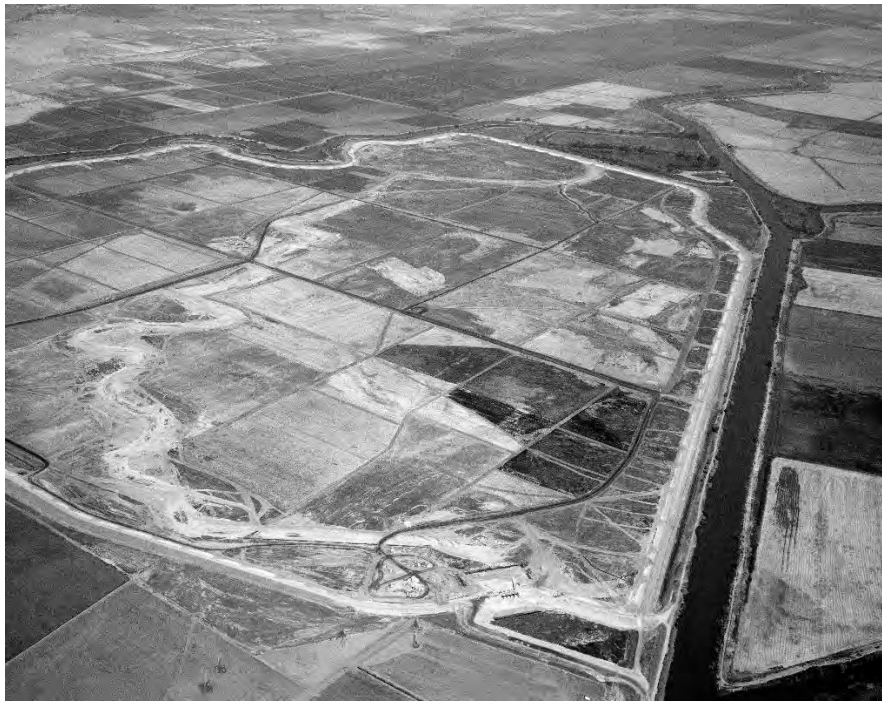
Exhibit C. 1969 aerial view looking northwest over the Clifton Court Forebay construction site showing the land divisions within the Clifton Court Tract before the completion of the project (DWR 1969).
