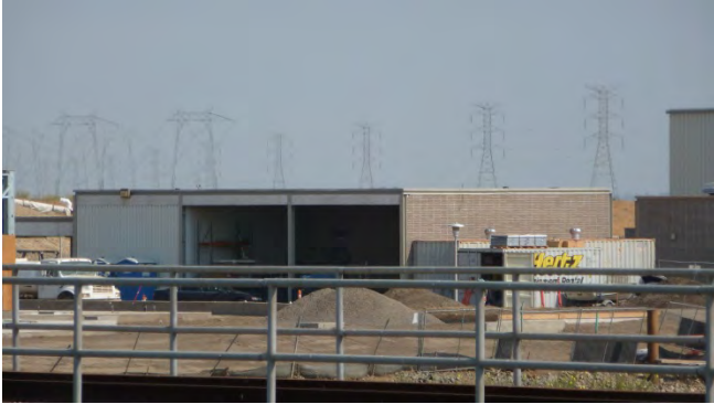
Photograph 12. Skinner Facility Building 3. View to north.
