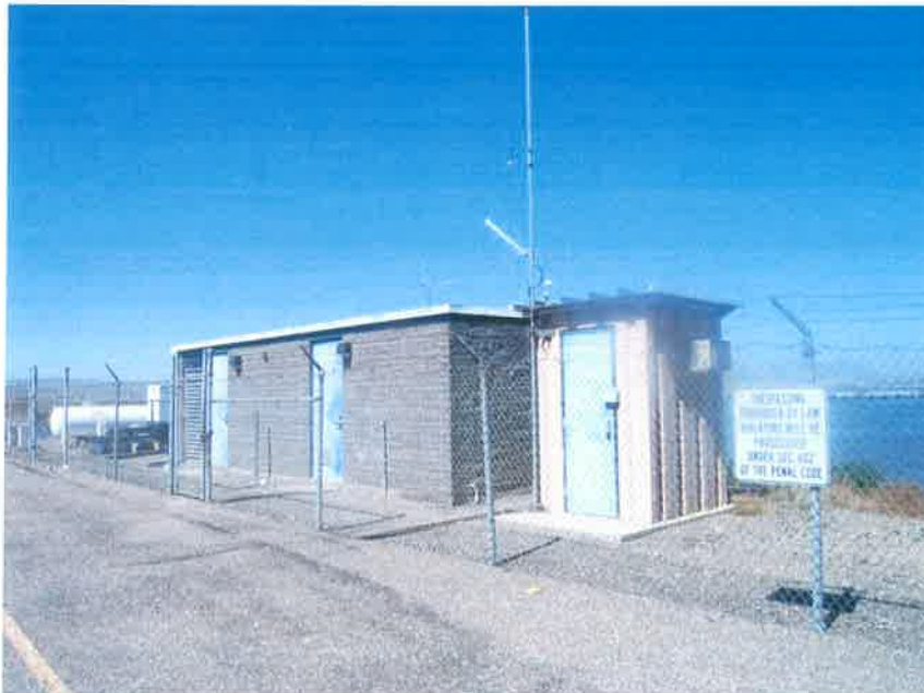
Photograph 8. Buildings, camera facing southwest
