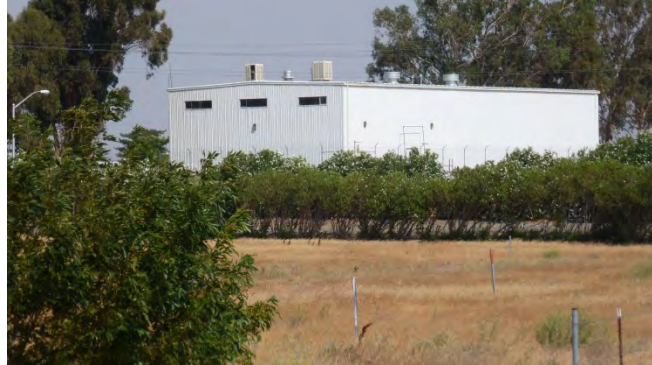
Photograph 19. Banks Plant Building 9. View to north.
