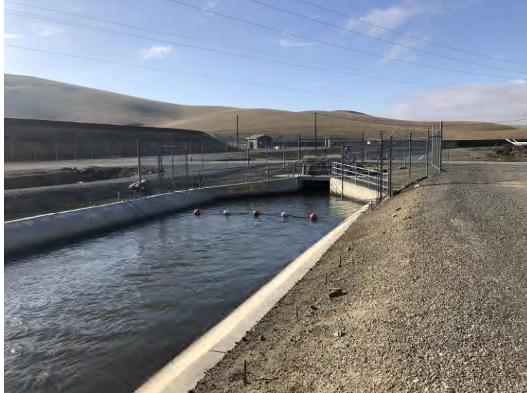
Figure 7. South Bay Aqueduct, Dyer Segment, looking south to check structure (IMG_4889)
