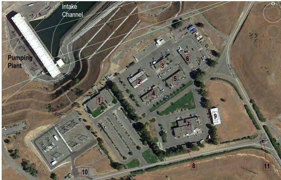
Figure 3. Aerial view of Harvey O. Banks Delta Pumping Plant. Source: Google Earth Pro, 2013.
