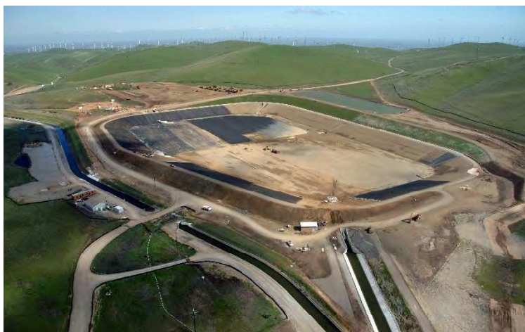
Exhibit D. Dyer Reservoir under construction, 2011 (DWR n.d.)
