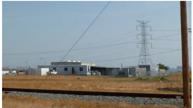
Photograph 15. Skinner Facility buildings with Building 12 at the far right.
