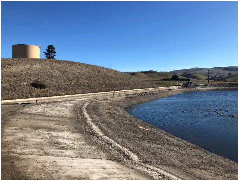
Figure 3. Patterson Reservoir, view looking southeast (IMG_4158)
