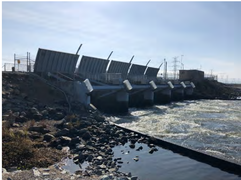
Figure 6. Clifton Court Forebay, gated intake control structure, looking southwest (IMG_3917)
