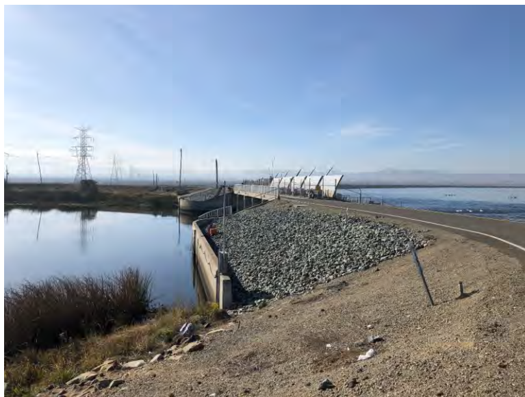
Figure 7. Clifton Court forebay, gated intake control structure, looking northwest (IMG_3924)
