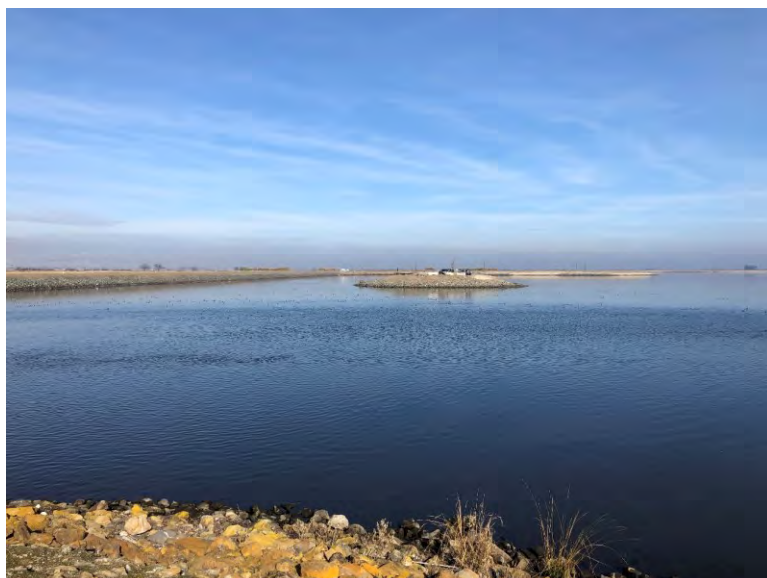
Figure 5. Clifton Court Forebay at California Aqueduct intake, looking north (IMG_3840)
