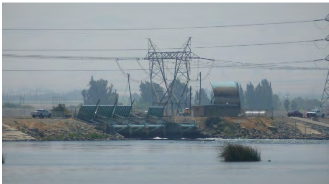
Photograph 6. Inside view of intake gates. View to south.
