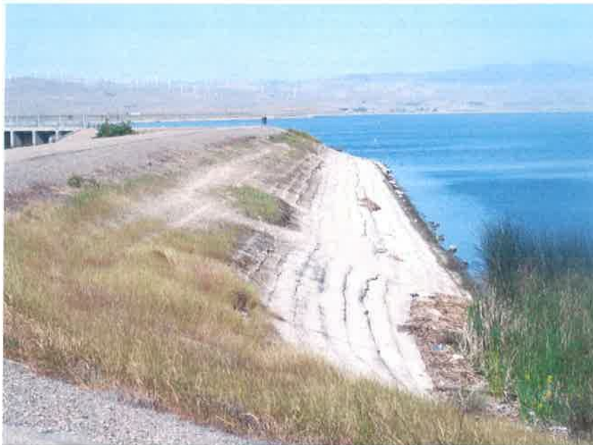
Photograph 2. Treated portion of dam, camera facing west
