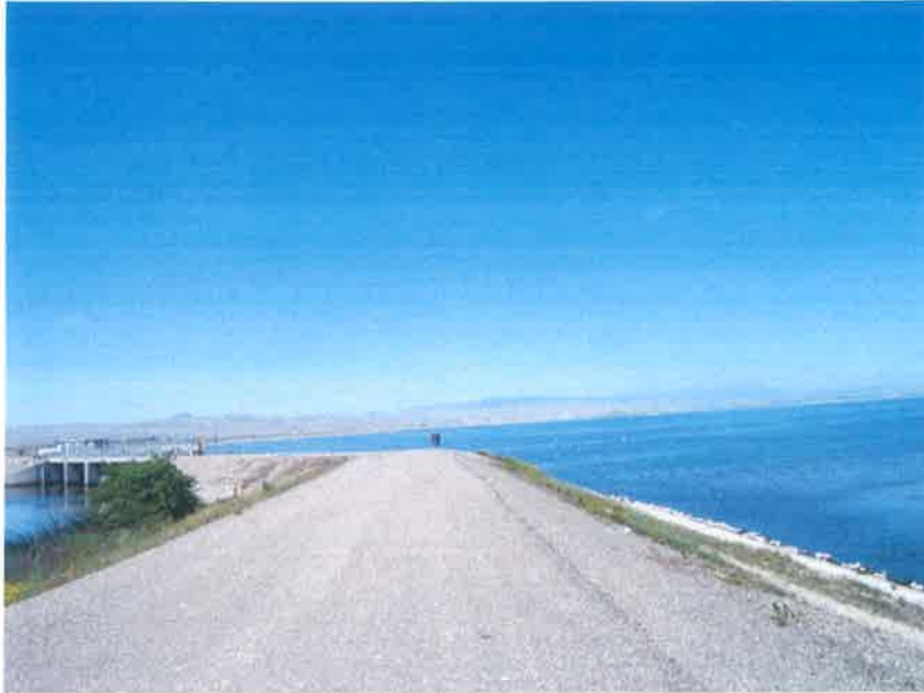
Photograph 3. Gravel levee road, camera facing west
