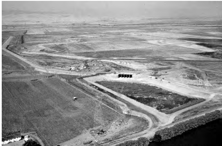
Figure 13. 1969 aerial view looking northwest over the Clifton Court Forebay construction site showing the inlet structure and its five control gates in the foreground (DWR n.d.).
