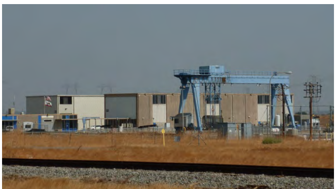
Photograph 10. Skinner Facility Buildings 2, 4, and 1 (L to R). View to north.
