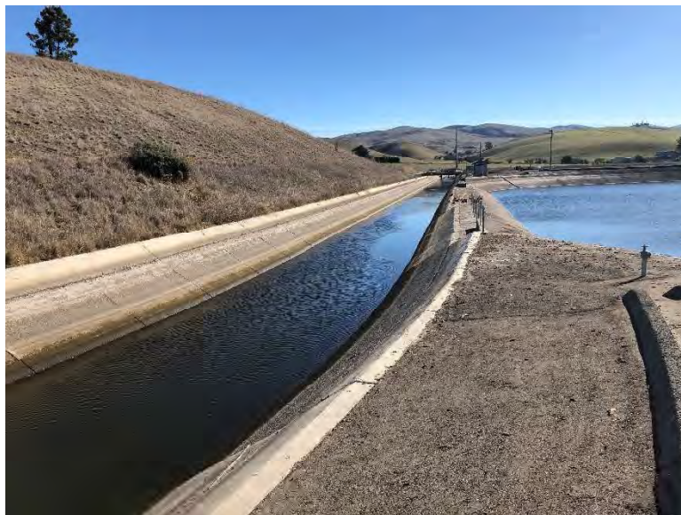
Figure 11. Patterson segment of South Bay Aqueduct, adjacent to Patterson Reservoir, view looking south (IMG_4163)
