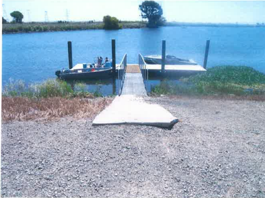
Photograph 9. Boat ramp/dock, camera facing south
