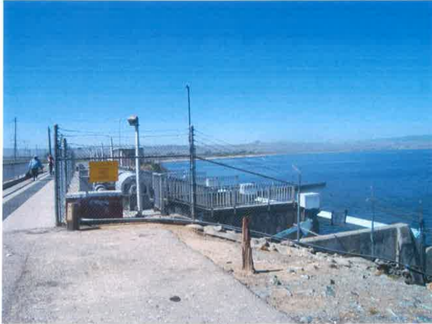
Photograph 5. Radial gates, camera facing southwest
