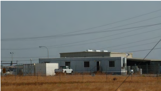
Photograph 14. Skinner Facility Buildings 10 and 11. View to north.
