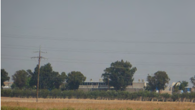
Photograph 18. Banks Plant Building 7. View to north.
