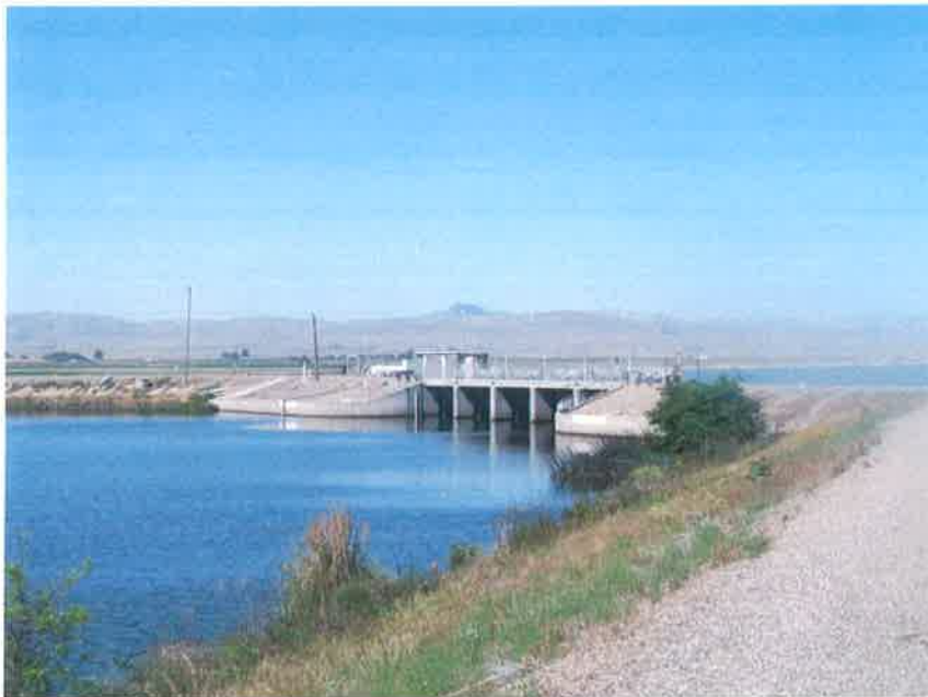
Photograph 4. Radial gates, camera facing southwest
