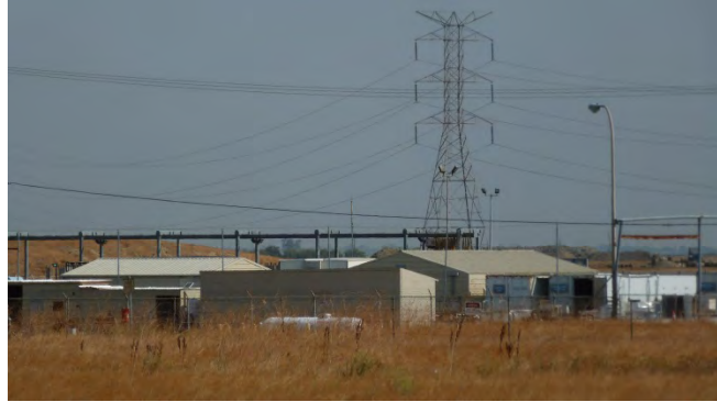
Photograph 13. Skinner Facility Buildings 7, 8, and 9. View to north.
