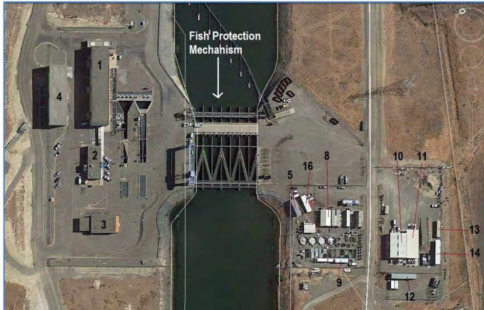
Figure 1. Aerial view of John E. Skinner Delta Fish Protective Facility. Source: Google Earth Pro, 2013.
