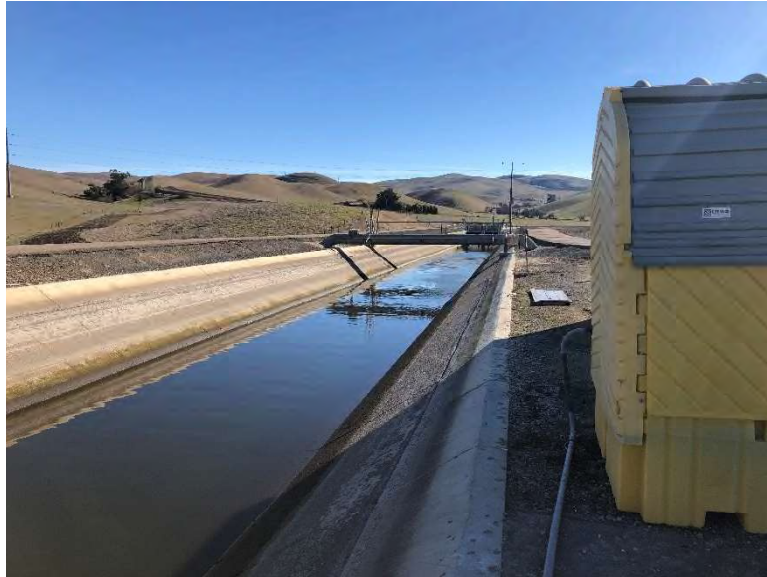
Figure 10. Patterson segment of South Bay Aqueduct, adjacent to Patterson Reservoir, view looking south (IMG_4129)
