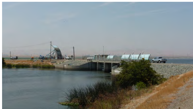
Photograph 4. Outside view of Clifton Court Forebay intake gate. View to west.
