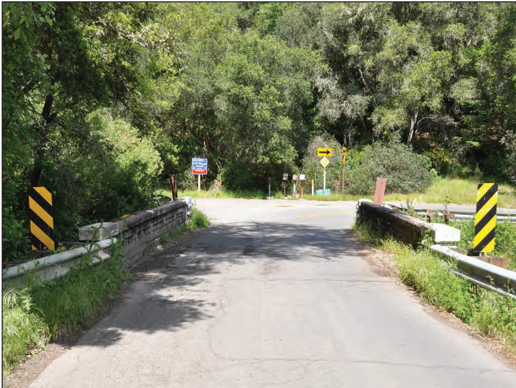
Figure 2. Dry Creek Road Bridge facing east; April 2017
