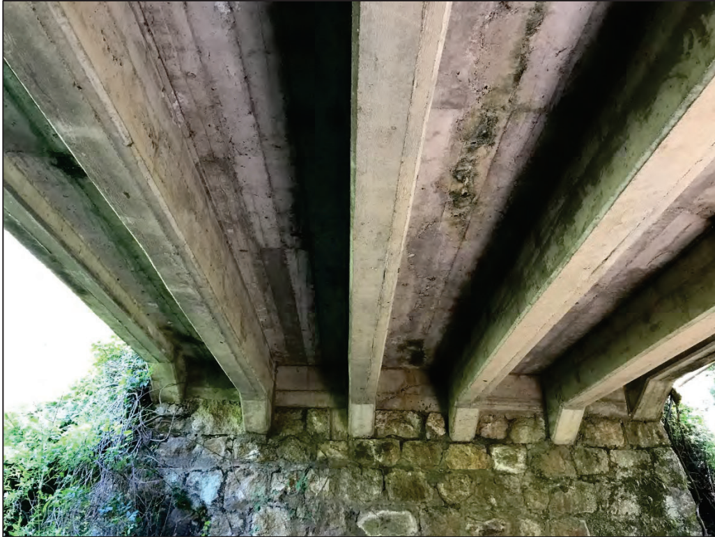
Figure 7. Underneath Dry Creek Bridge facing east; May 2017
