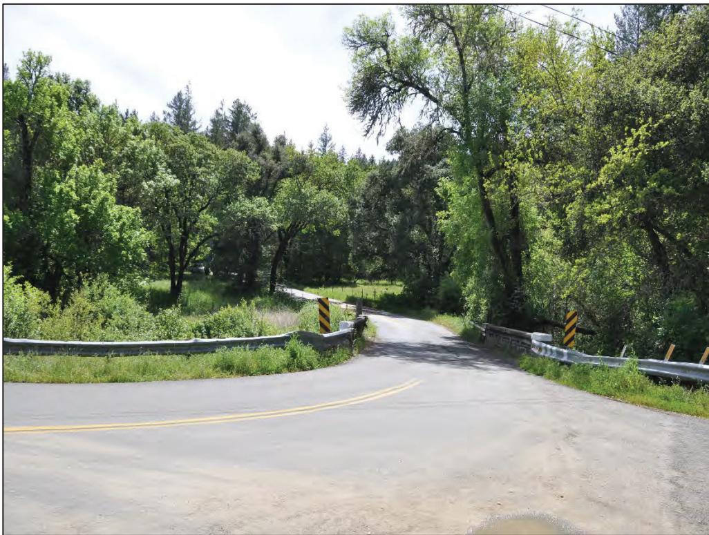
Figure 4. Dry Creek Road Bridge northern approach from the southwest; April 2017
