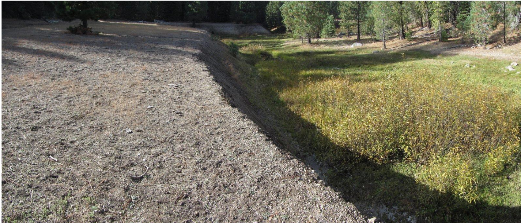
Figure 15. Plot 65, on dry terrace at left, has strongly mottled wetland soils but the 8-foot deep erosion gully to the right has dewatered this terrace and it no longer has wetland hydrology or wetland plants.
