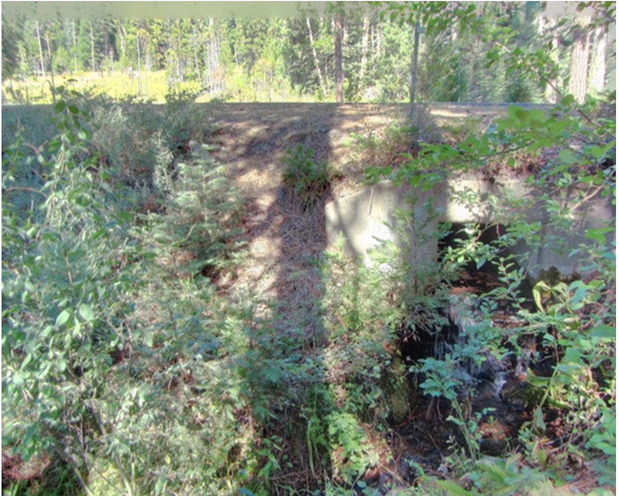
Photo 7: View Looking Upstream at Concrete Culvert Under Highway 36E
