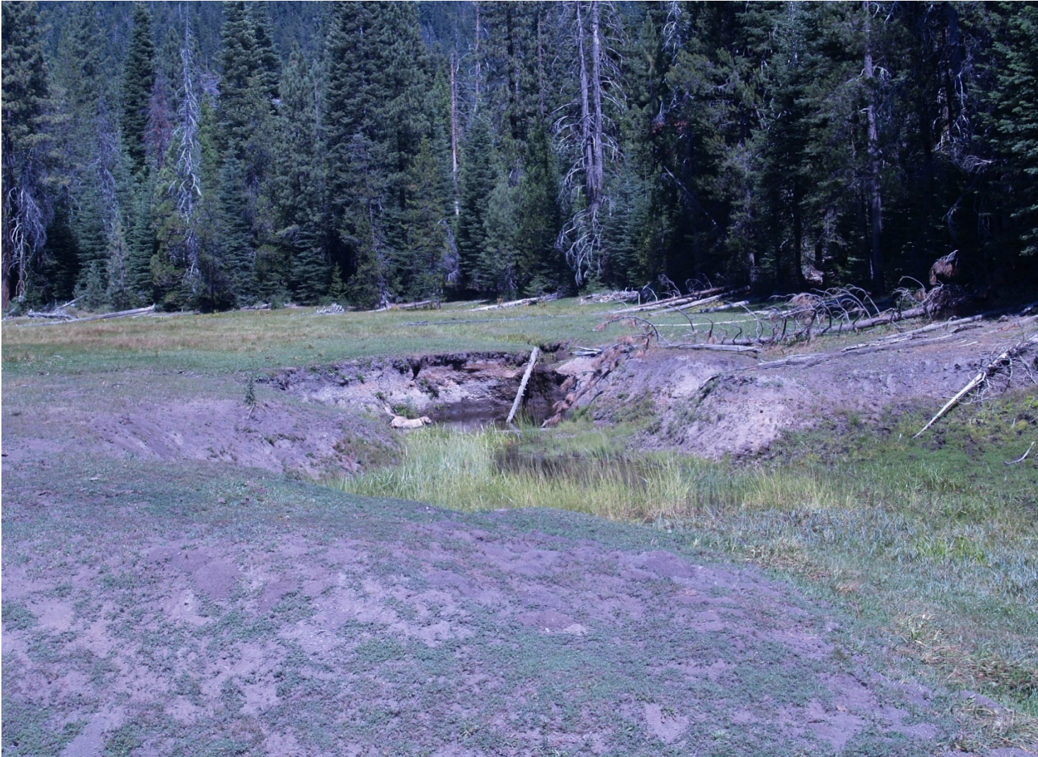
Photo AES 9: Overview of a Head Cut and Surrounding Impacted Area
