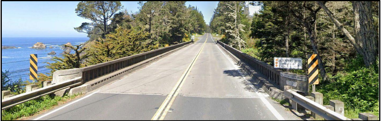
Figure 2. Existing Jack Peters Creek Bridge
