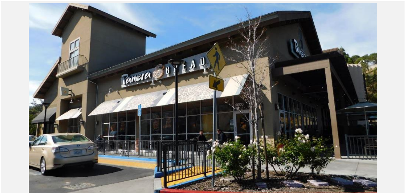
Photograph 21. Panera: South and west elevations, view to northwest (DSCN9562)
