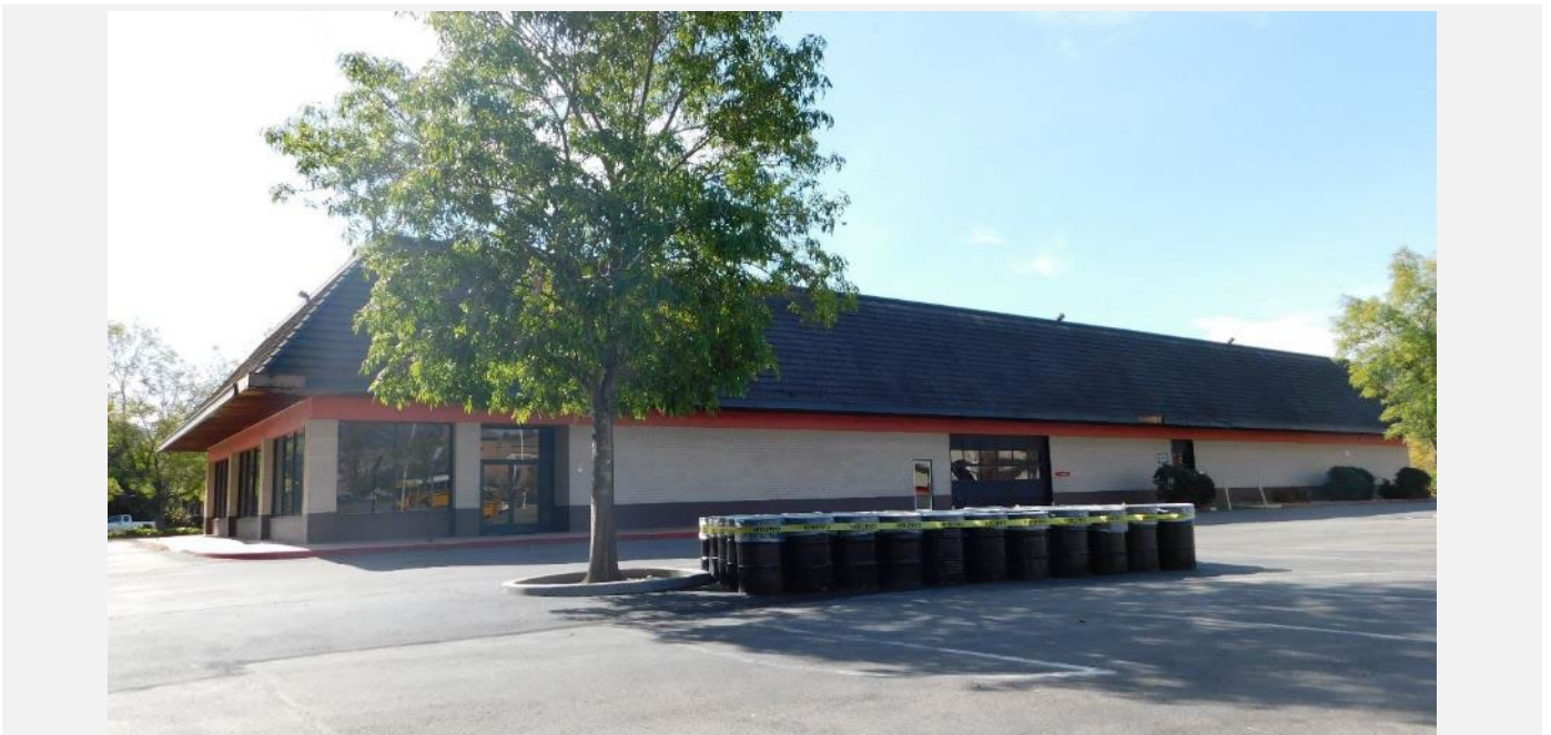
Photograph 14. Sears Automotive Center: East (main) and north elevations, view to southwest (DSCN9481)
