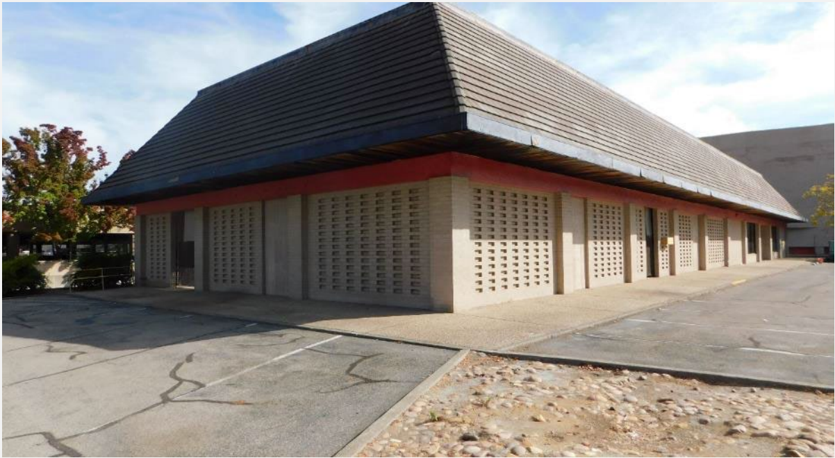
Photograph 15. Sears Seasonal Sales Building: West and south (main) elevations, view to northeast (DSCN9454)
