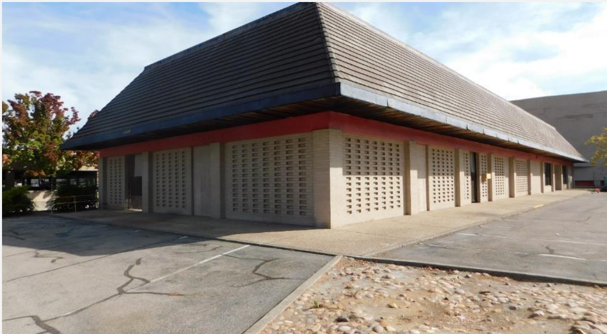
Exhibit 29. Sears Seasonal Sales Building: West and south (main) elevations, view to northeast (DSCN9454)
