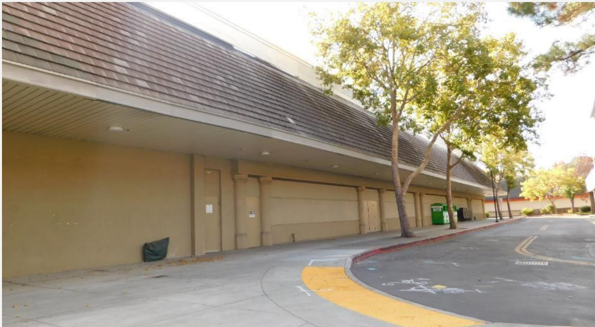
Exhibit 22. Northgate Mall Unit 4: West (main) elevation, view to southeast (DSCN9420)
