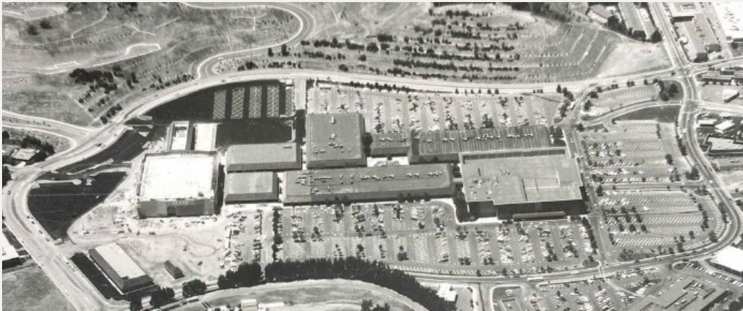
Photograph 31. Detail of a historical aerial photograph in 1972 showing Units 4 and 5 between the nearly completed Sears buildings at the far left and the original 1964 sections of the Northgate Mall at right (Courtesy of the Marin History Museum Brady Collection)
