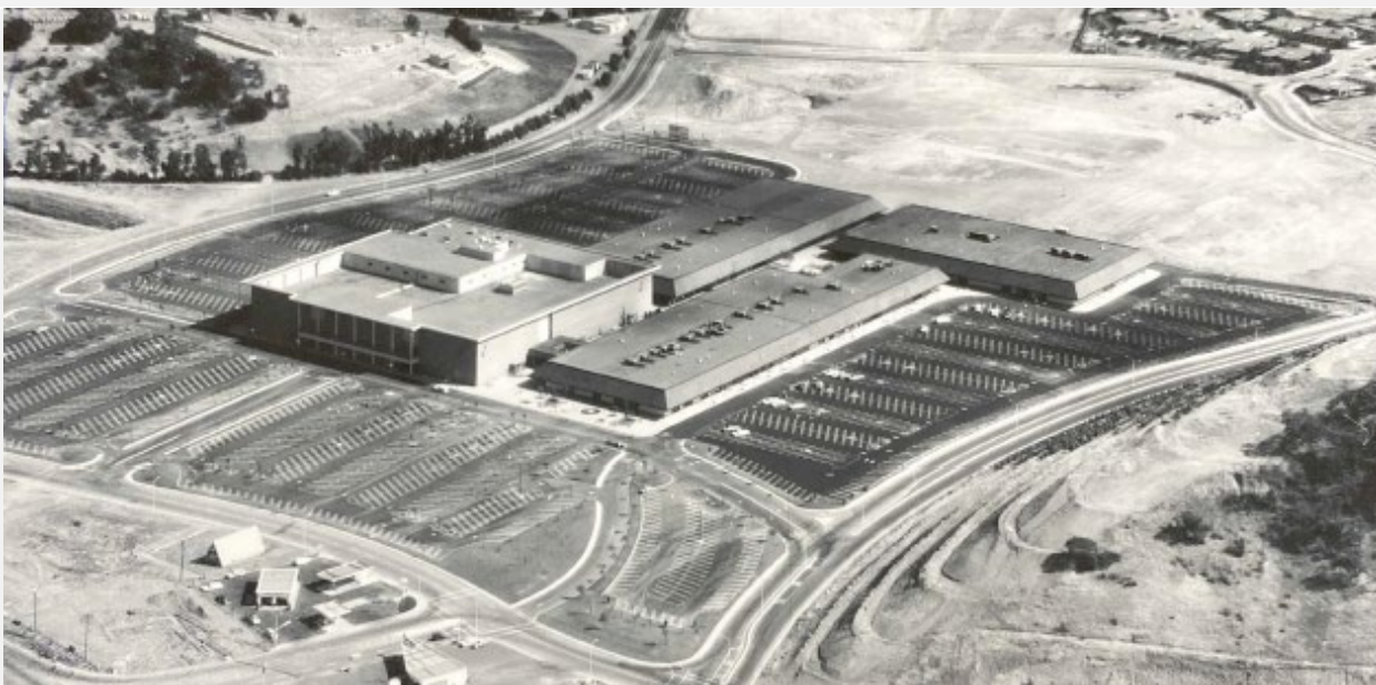
Photograph 26. Detail of a historical aerial photograph looking southwest at the Northgate Mall as it appeared in 1965 with the Emporium building at the left foreground flanked by Northgate Mall Units 1, 2, and 3. (Courtesy of the Marin History Museum Brady Collection)
