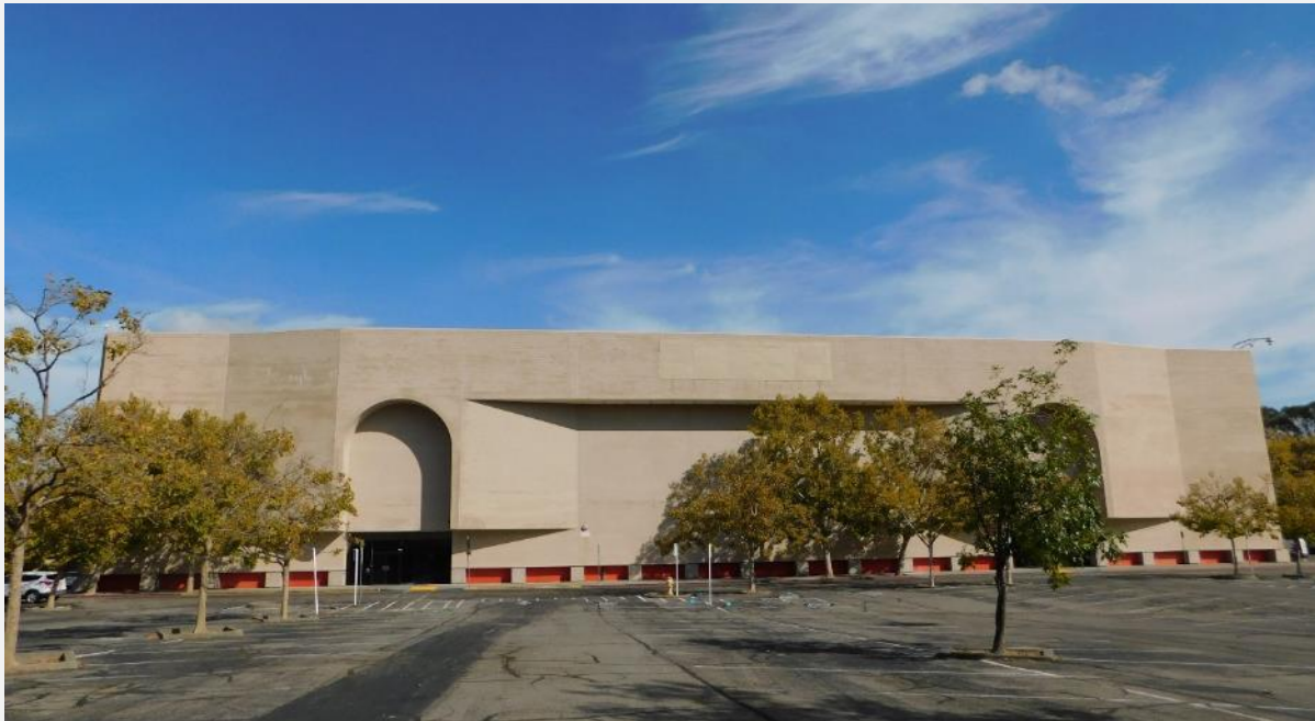
Exhibit 25. Sears: South (main) elevation, view to north (DSCN9464)
