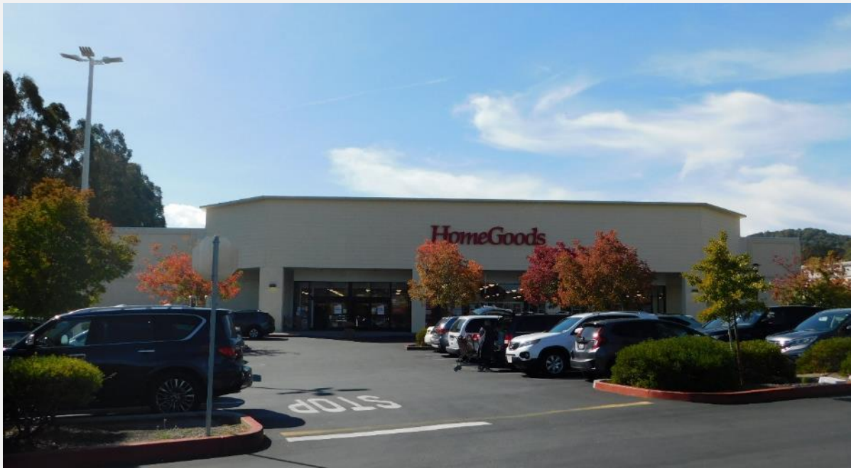
Exhibit 33. Home Goods: West and north elevations, view to southwest (DSCN9533)
