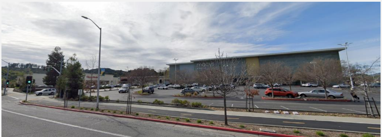
Exhibit 16. Contextual Overview of the Northgate Mall, view looking west from Las Gallinas Avenue (Google Earth 2021)
