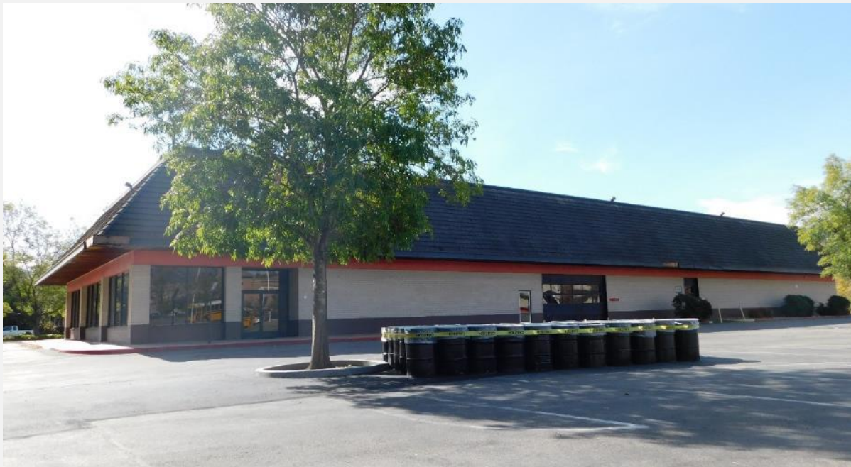
Exhibit 28. Sears Automotive Center: East (main) and north elevations, view to southwest (DSCN9481)
