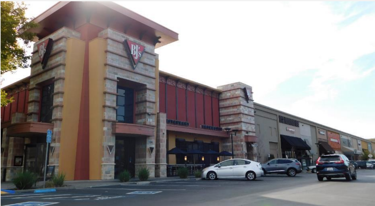
Exhibit 19. Northgate Mall Unit 1: West (main) elevation, view to southeast (DSCN9402)
