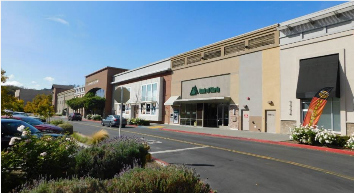
Photograph 6. Northgate Mall Unit 2: east (main) elevation, view to southwest (DSCN9515)
