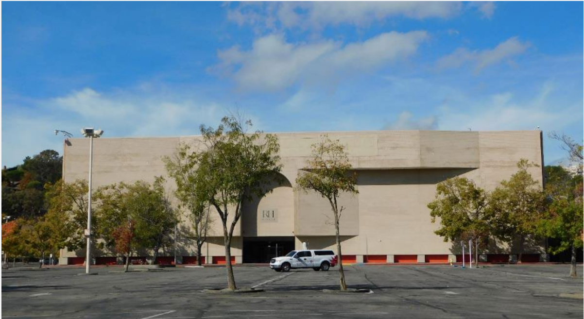
Photograph 12. Sears: East elevation, view to west (DSCN9502)
