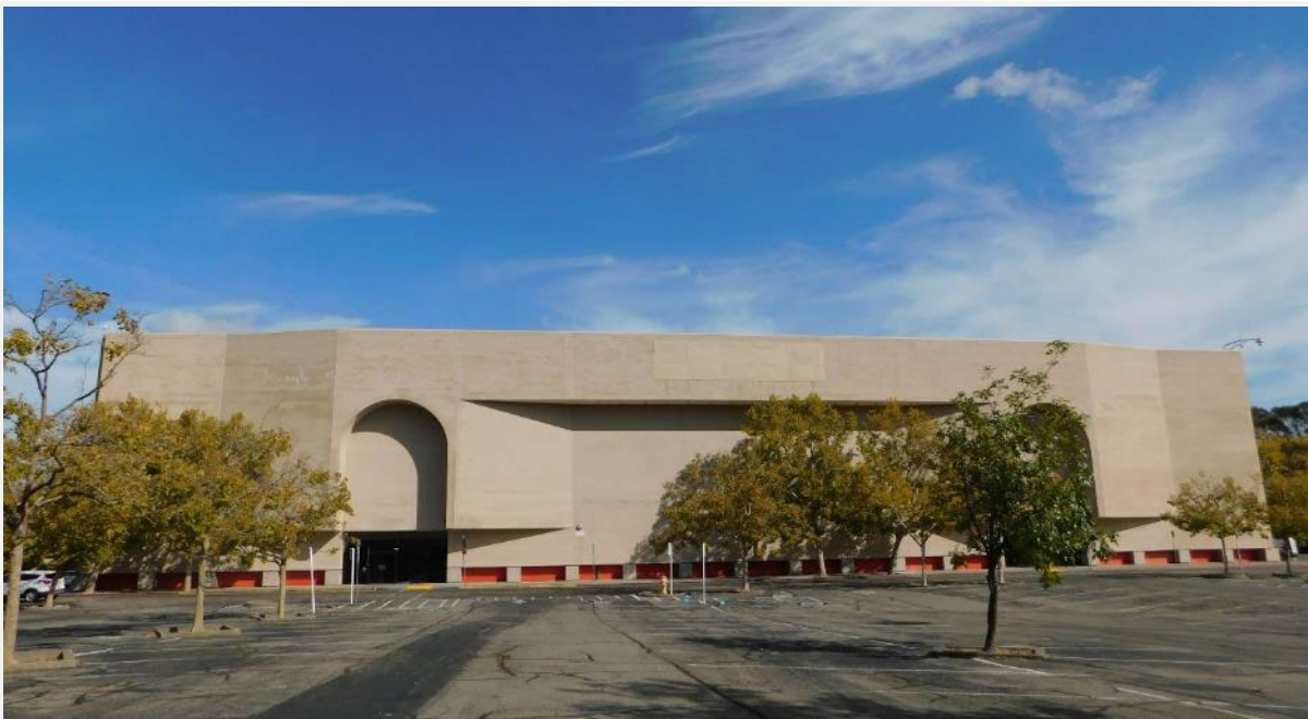
Photograph 11. Sears: South (main) elevation, view to north (DSCN9464)
