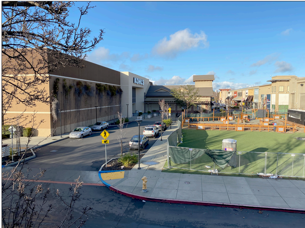
Photo 2: Photo of Kohl's building and Mall Shops West from the parking structure, looking north
