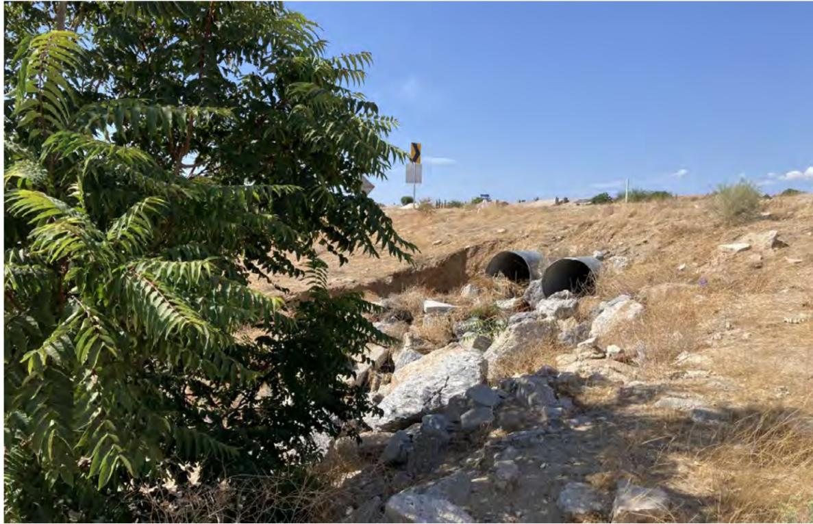
Photograph 1: Photo looking southwest (offsite) from western boundary of the Project site. Photo depicts piped culvert that conveys Drainage A beneath Hesperia Road.
