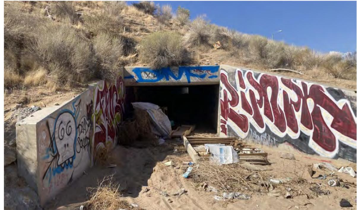
Photograph 4: Photo looking southwest within Drainage B near southern perimeter of the Project site. Photo depicts box culvert that conveys Drainage B beneath Ottawa Street.
