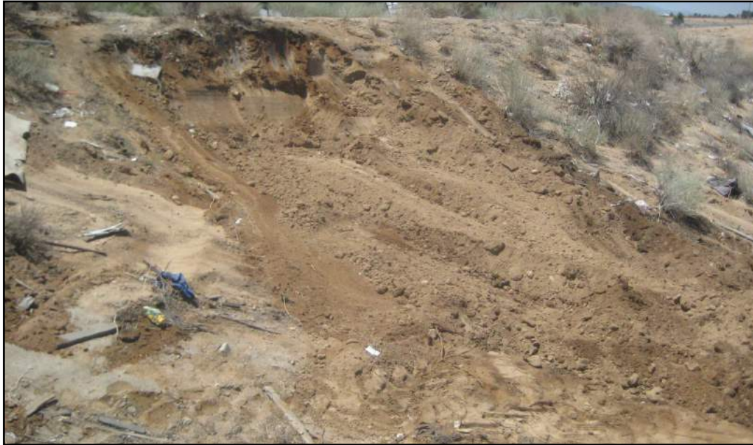
Photo 5—Excavated slope on parcel 551-07.
