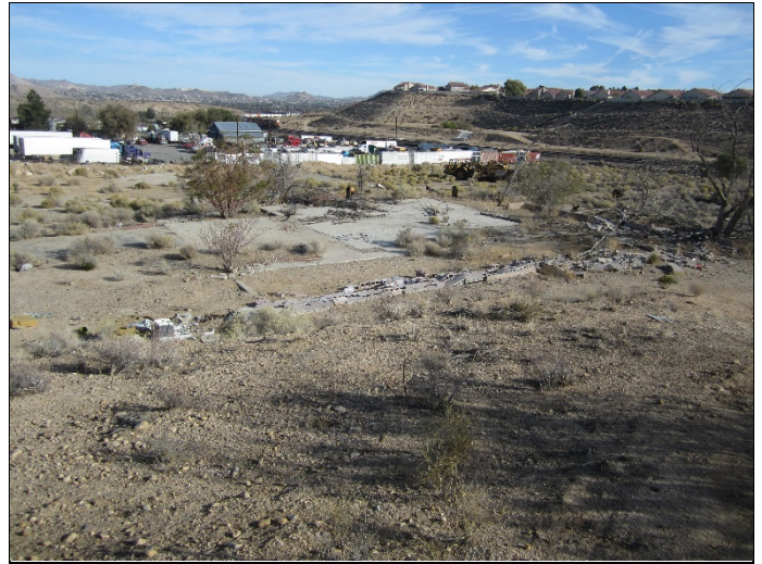
8. View of building foundations and debris on APNs 3090-531-03 and 3090-531-04.
