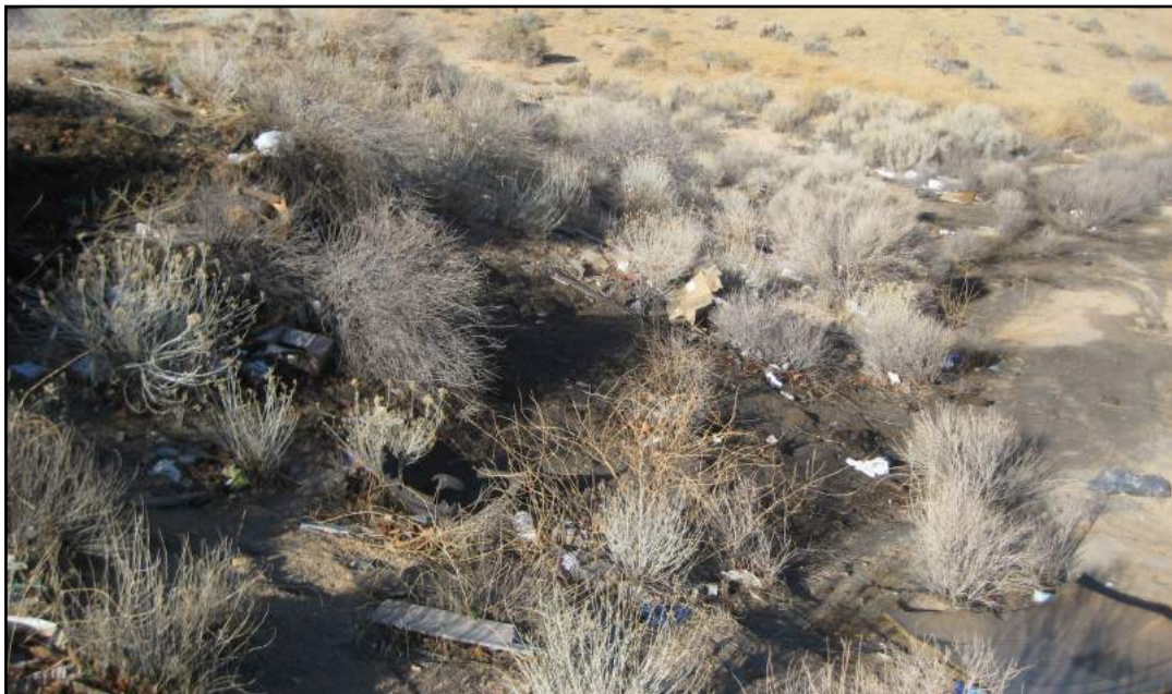
Photo 34—View toward northwest of debris and stained soil on slope adjacent to cul-de-sac on parcel 551-07.
