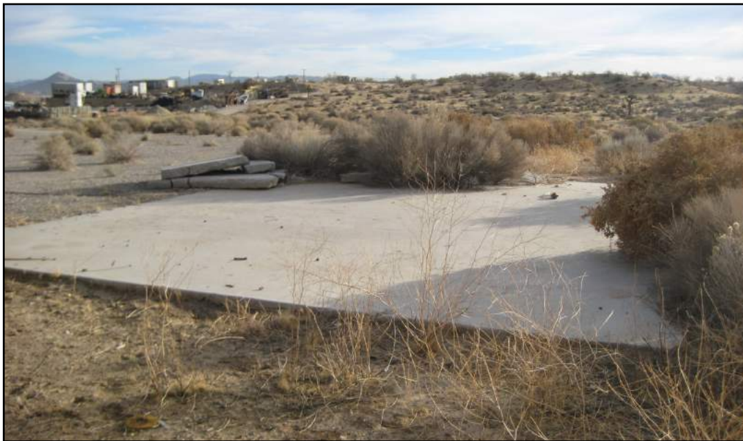
Photo 4—View toward northeast of concrete pad in southwestern portion of parcel 401-08.
