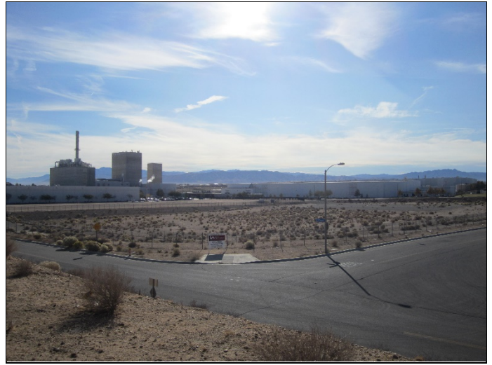
26. View of vacant land adjacent south.
