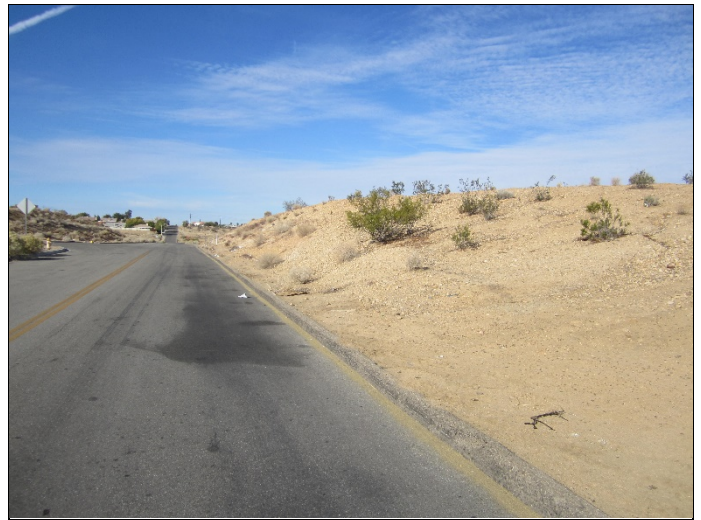
28. View west along Ottawa Street adjacent south of the subject property.
