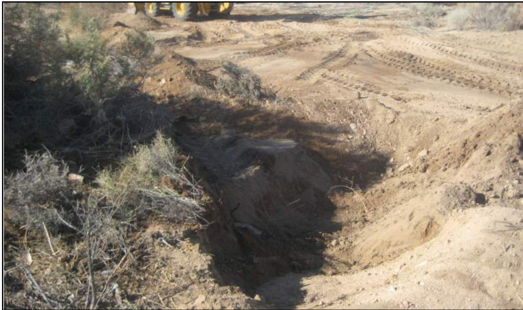
Photo 4—Excavation to 2 1/2 feet deep on parcel 551-07.
