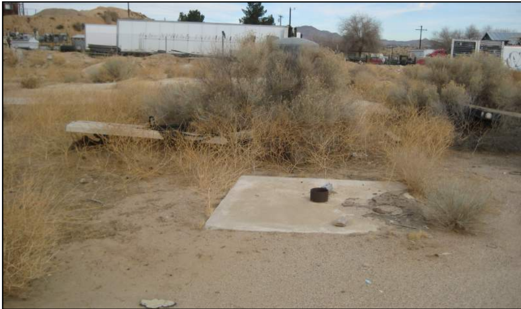
Photo 46—View toward north of former well and pressure tank in northwestern portion of parcel 531-04.
