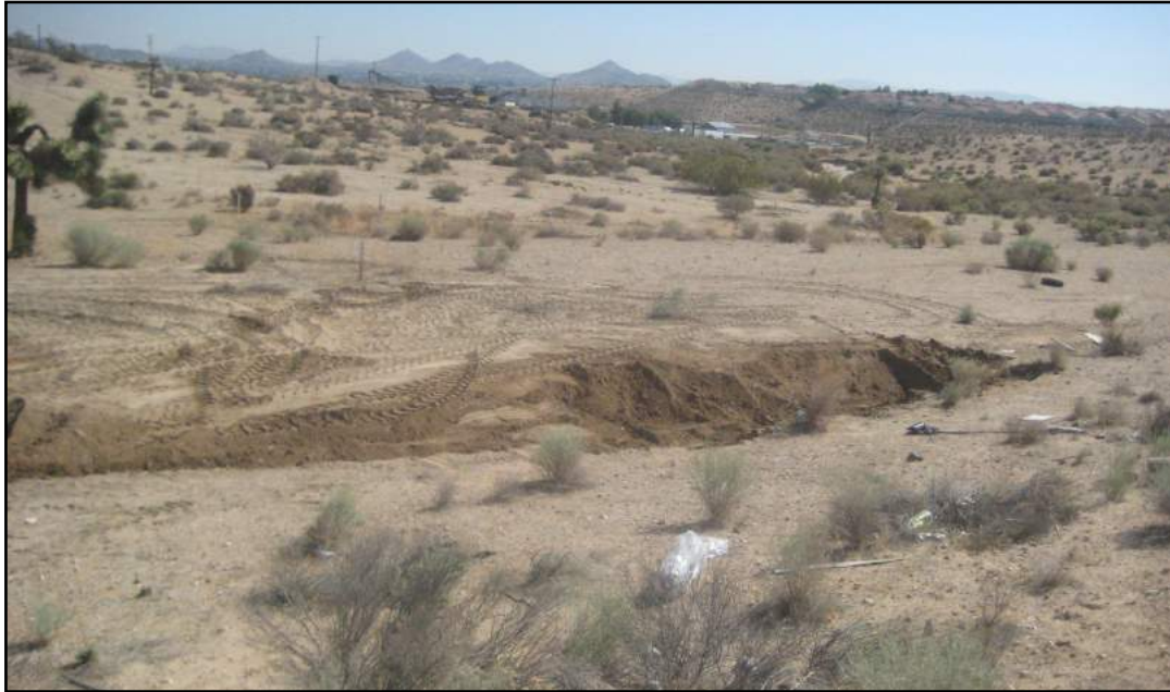
Photo 1—Excavation to 2 feet deep on parcel 441-04.
