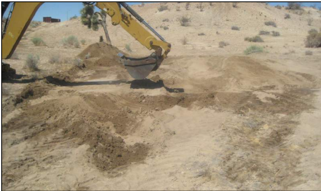
Photo 2—Excavation in progress in northeastern portion of excavation on parcel 441-04.
