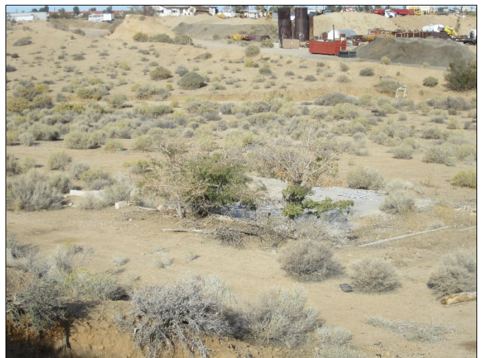
10. View of structure foundation on APNs 3090-531-03 and 3090-531-04.
