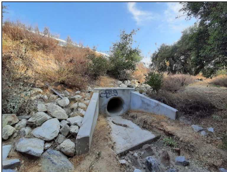
Photo 8. Culvert in northeast buffer, adjacent to Project site.
