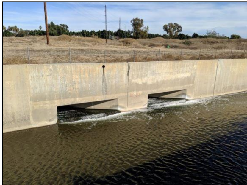
Figure 2.2-3. DCTWRP Outfall into the Los Angeles River below the Sepulveda Dam
