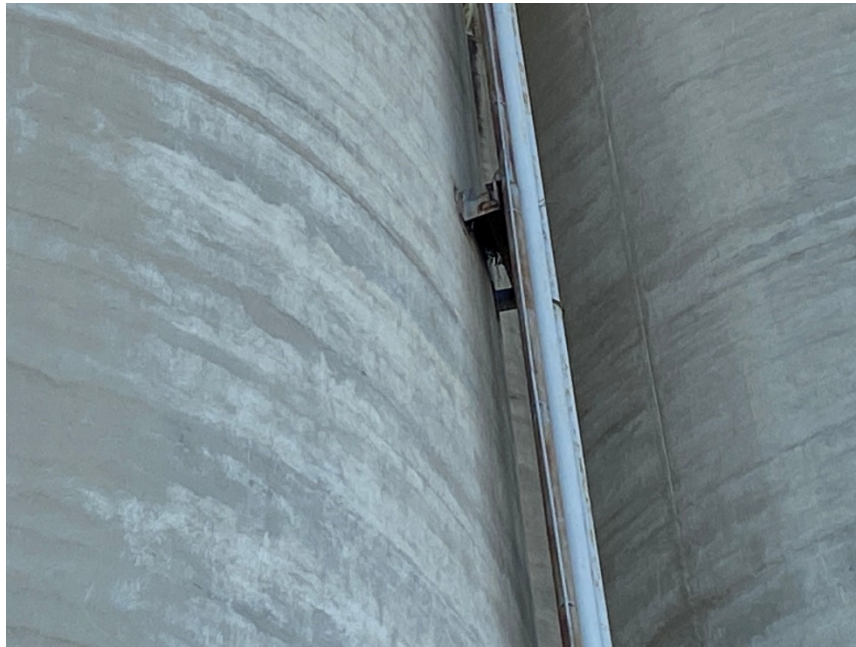
10. Photograph shows platform nest along storage silo.
