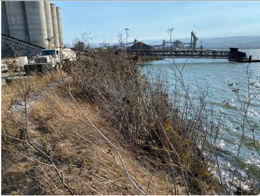
5. Photograph shows interface between western shoreline and Redwood Creek channel, facing south.
