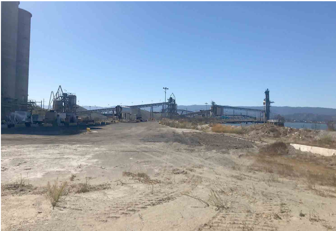
Photo No. 2 Existing Aggregate Processing Area South of Ready-mix concrete plant site. Aggregate Conveyors and Wharves in Background
