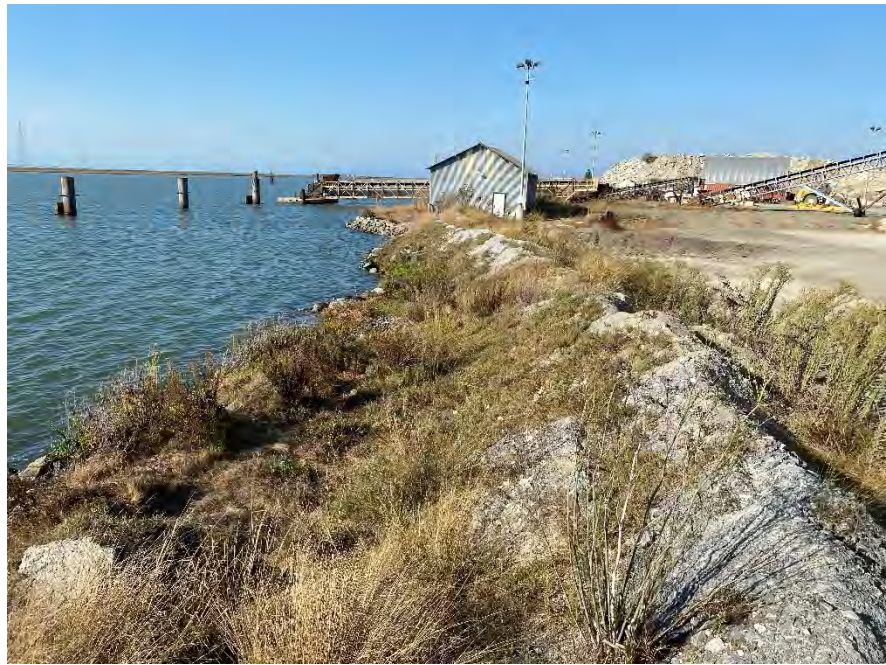
6. Photograph existing condition along western shoreline, facing north/northeast.
