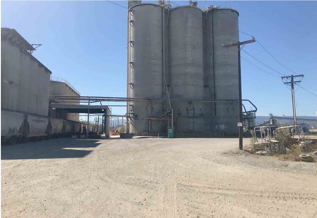
Photo No. 1 Proposed Ready-Mix Concrete Plant Location, Looking West
