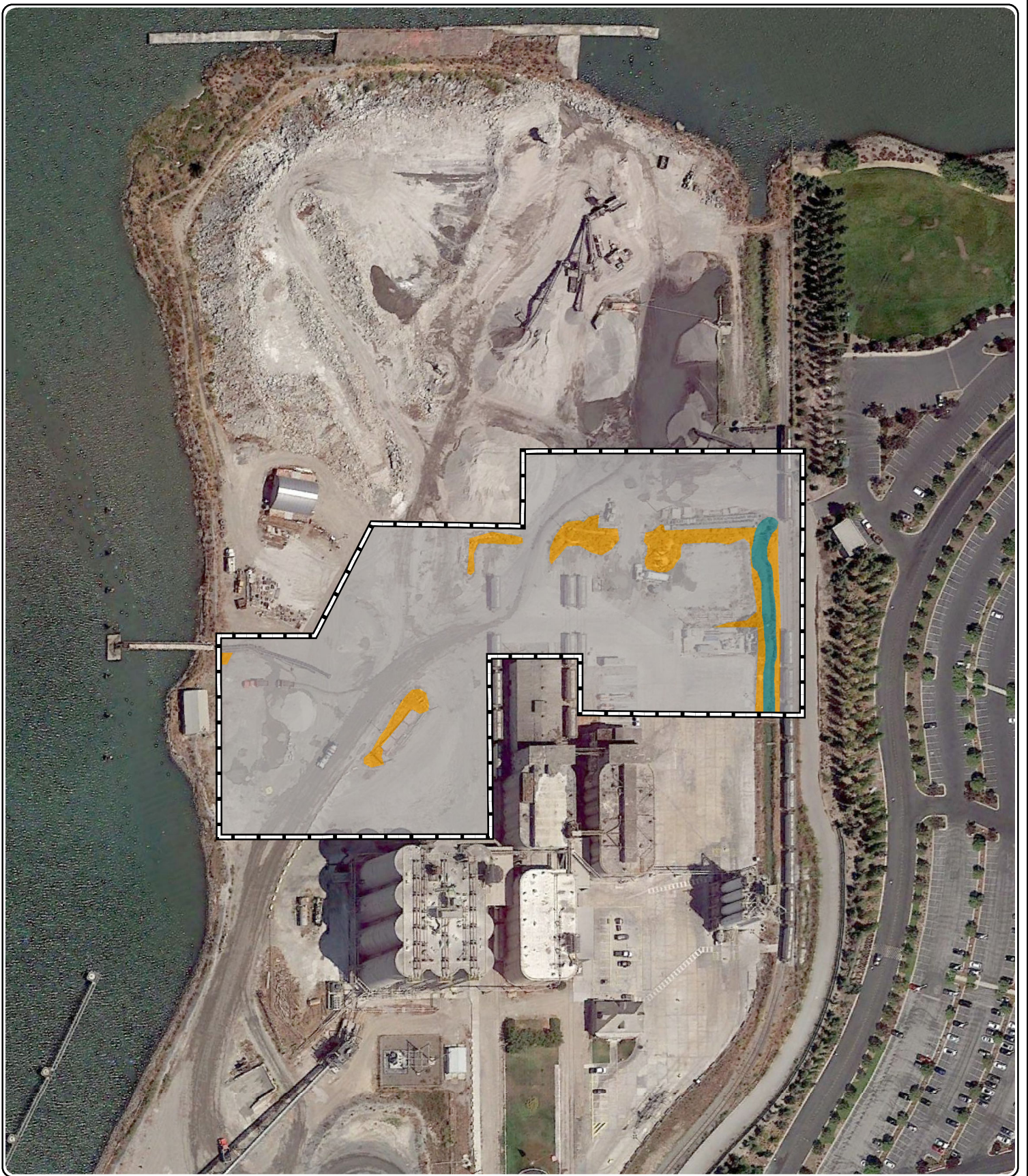
Aerial photo adapted from Google Earth Maps Imagery Date 8-9-2018.
