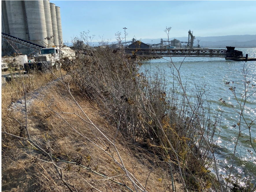
7. Photograph shows interface between western shoreline and Redwood Creek channel, facing south.
