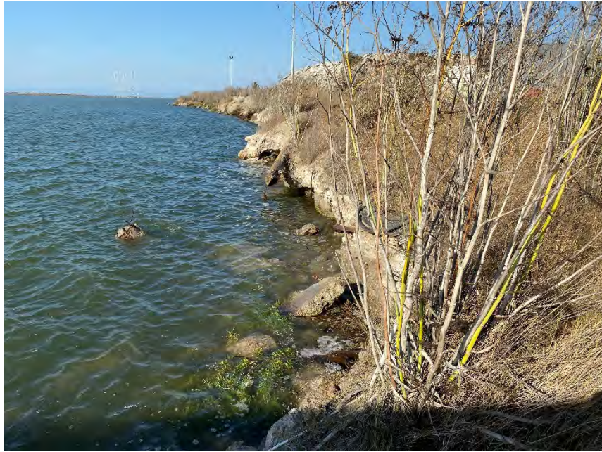
7. Photograph shows existing conditions along shoreline, facing northeast.
