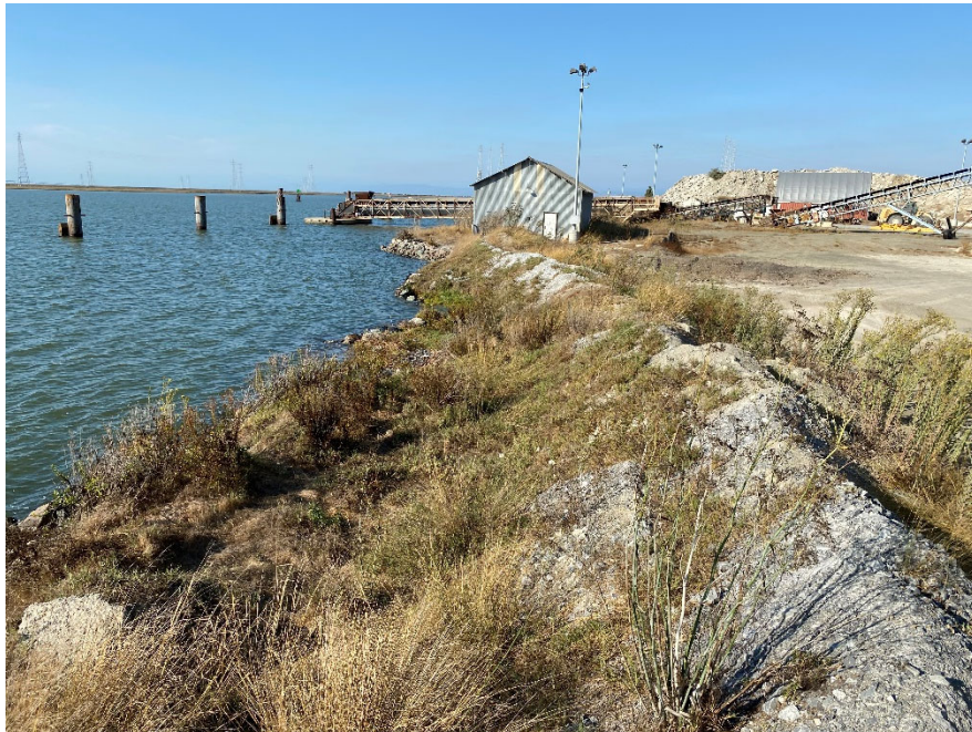
8. Photograph existing condition along western shoreline, facing north/northeast.
