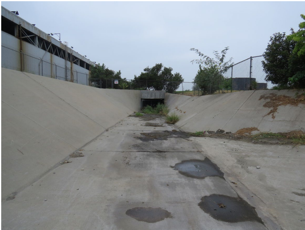
Photograph 14: From within the concrete-lined trapezoidal channel that parallels the southern boundary of the project site. Looking west towards the culvert that conveys flows from the western portion of the project site into San Sevaine Channel.
