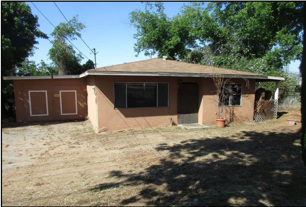
PHOTOGRAPH 1 Facade of House at 2355 Montiel Road, Looking Southwest
