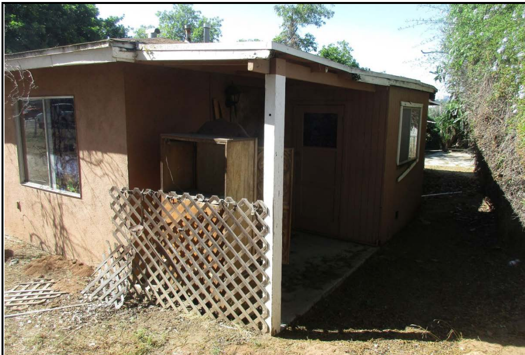
PHOTOGRAPH 6 Covered Porch at the Northwest House Corner
