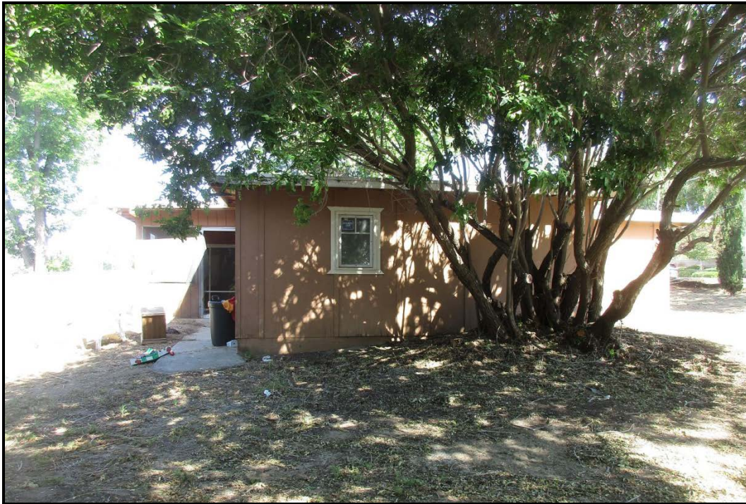
PHOTOGRAPH 3 Southeast Elevation, Showing Garage. Looking Northwest
