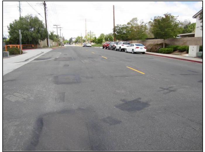
20. Street view to west on Montiel Road.
