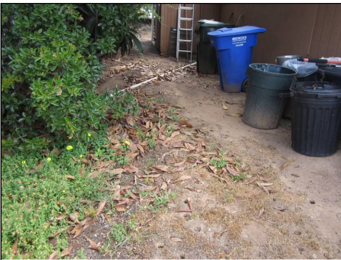
11. Septic tank area at 2355 Montiel Road.
