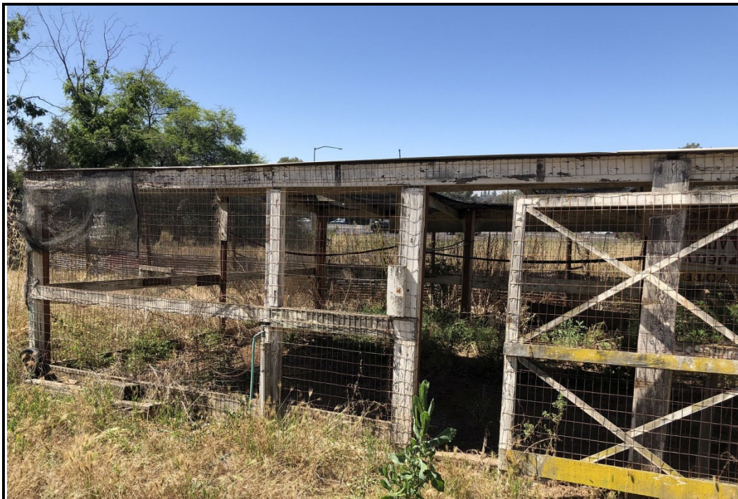
PHOTOGRAPH 6 Typical Pen-type Structure
