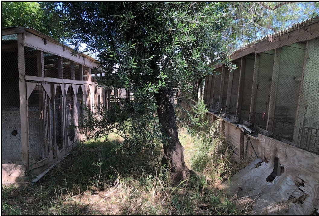
PHOTOGRAPH 5 Typical Wood Framed Structures
