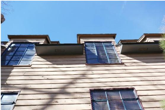
Figure 15: Detail of windows and boxed eaves at plan east façade.
