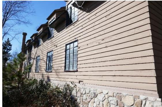
Figure 16: North end of plan east façade with peeling paint, looking southwest.
