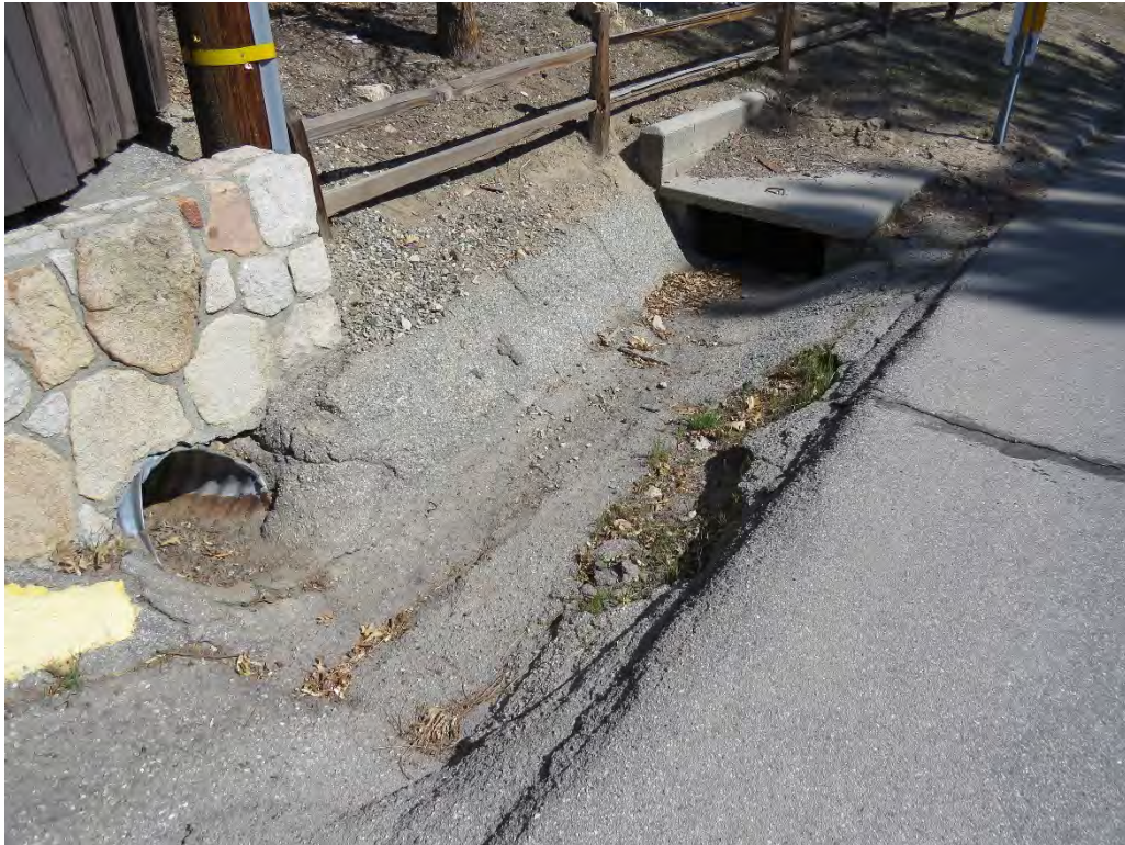
Photograph 10: Culvert outlet under the existing maintenance building.
