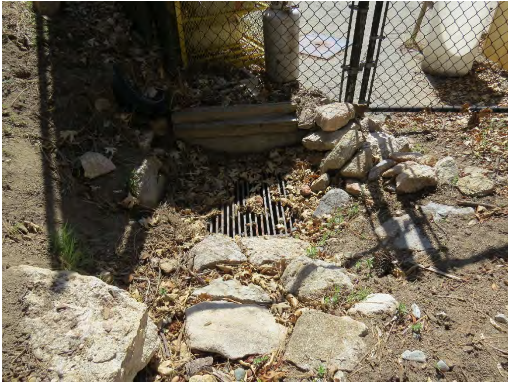
Photograph 9: Drainage inlet under that conveys flows under the existing maintenance building.
