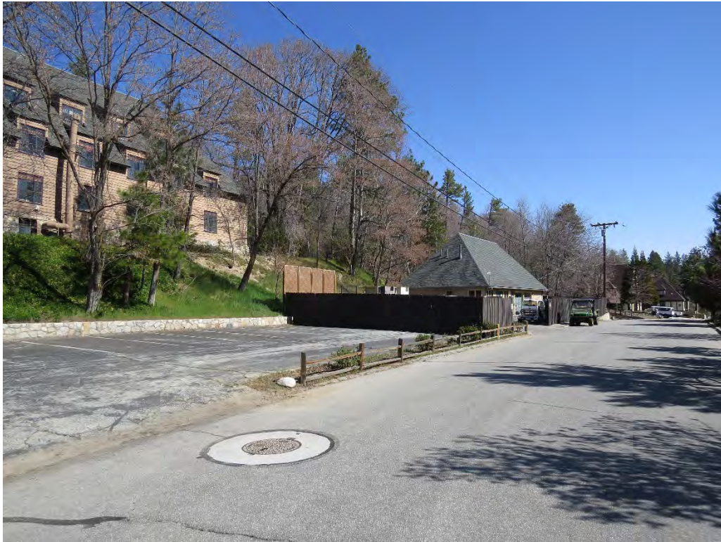
Photograph 1: From southeast corner of the project site looking north at the existing paved street, Cedar Building and maintenance building.
