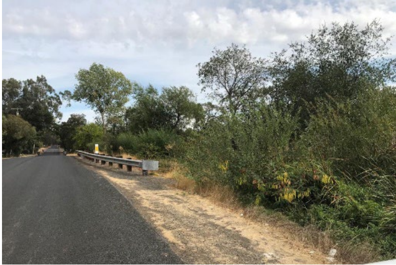
Photo 1. Bridge crossing over seasonal channel between Railroad Avenue and Melvina Avenue. All planned construction will take place within the roadway right-of-way.
