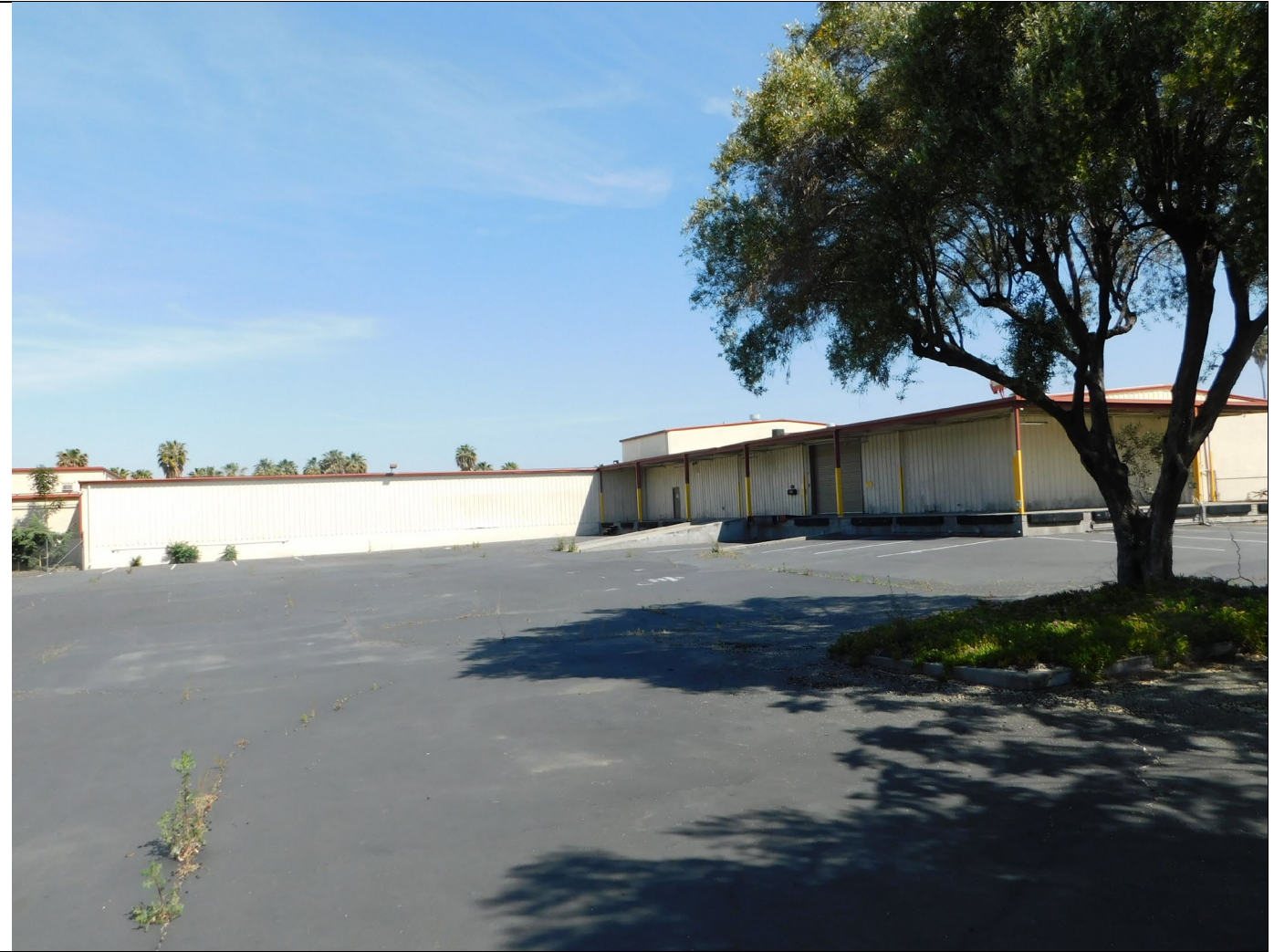
Photograph 4. Building A's : West (main) elevation, view looking east (IMG_9079)
