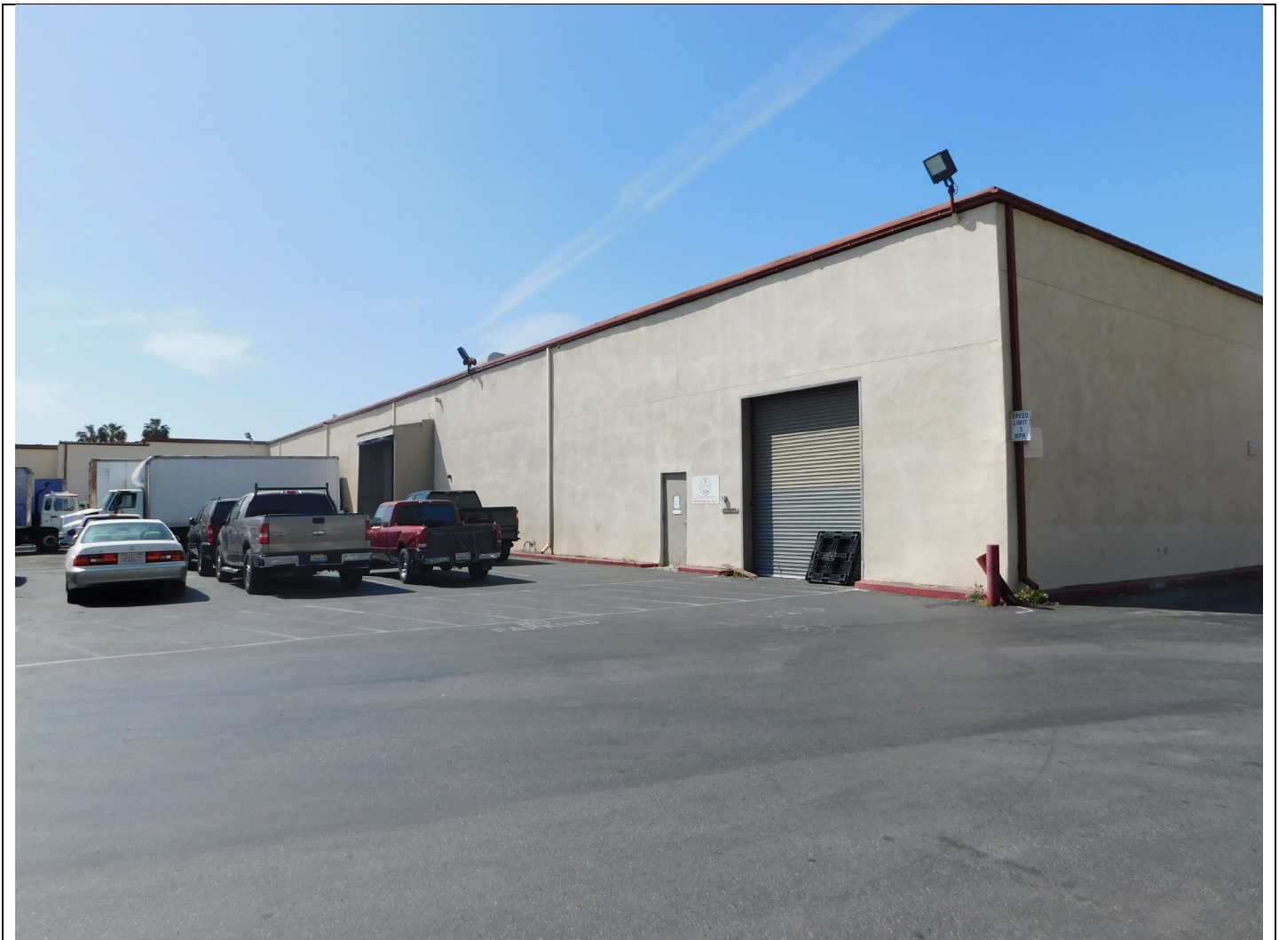
Photograph 3. Building A's east elevation, view looking south (IMG 9042)
