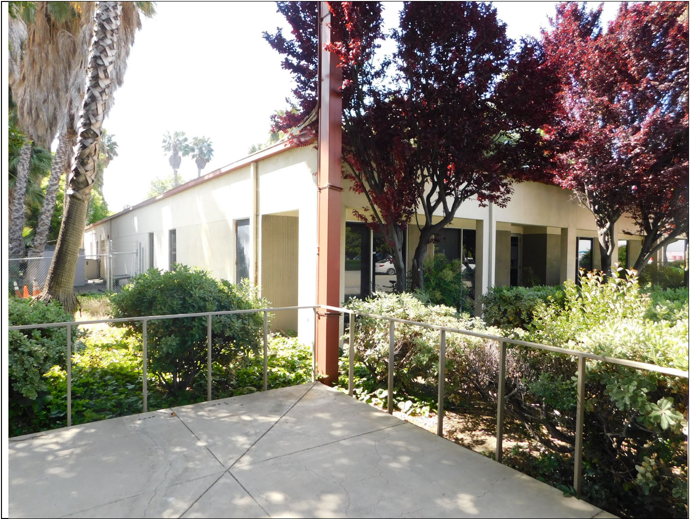
Photograph 6. Building B: South (main) elevation and view looking west (IMG_9000) looking south (IMG_9014)
