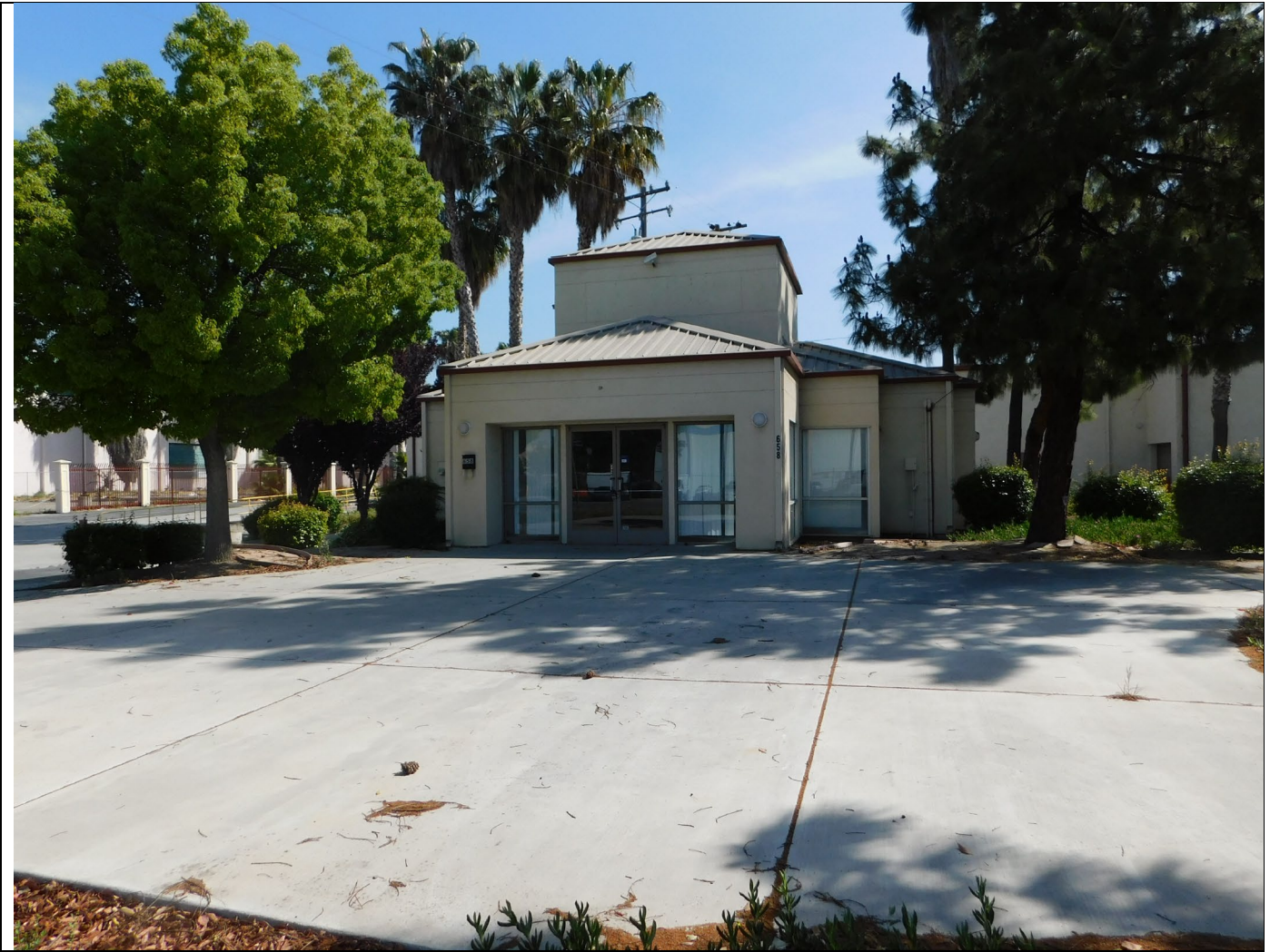
Photograph 8. Building C: West (main) elevation, view looking east (IMG 8985)
