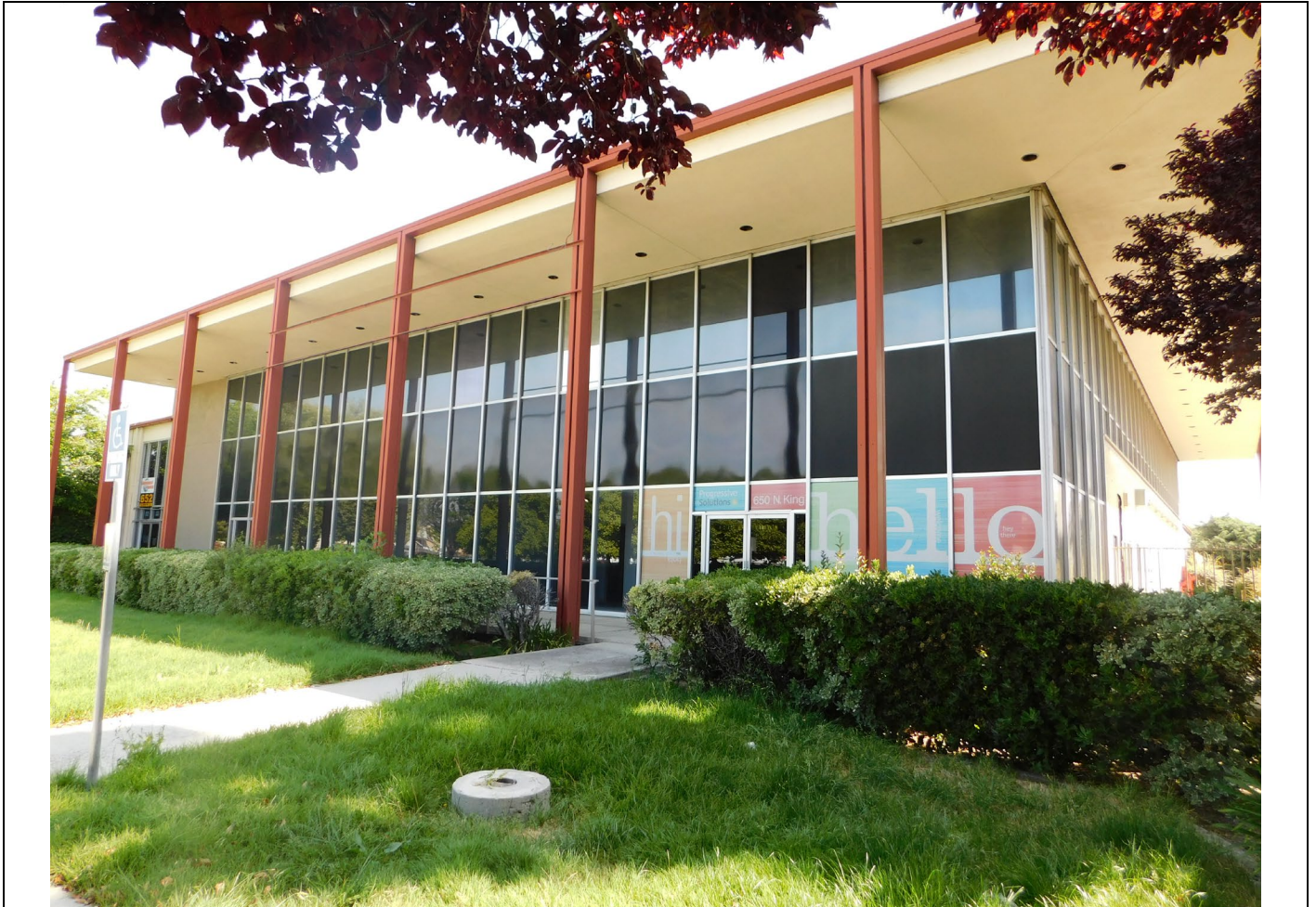
Photograph 2. Building A's west (main) and partial south elevations, view looking east (IMG 8971)
