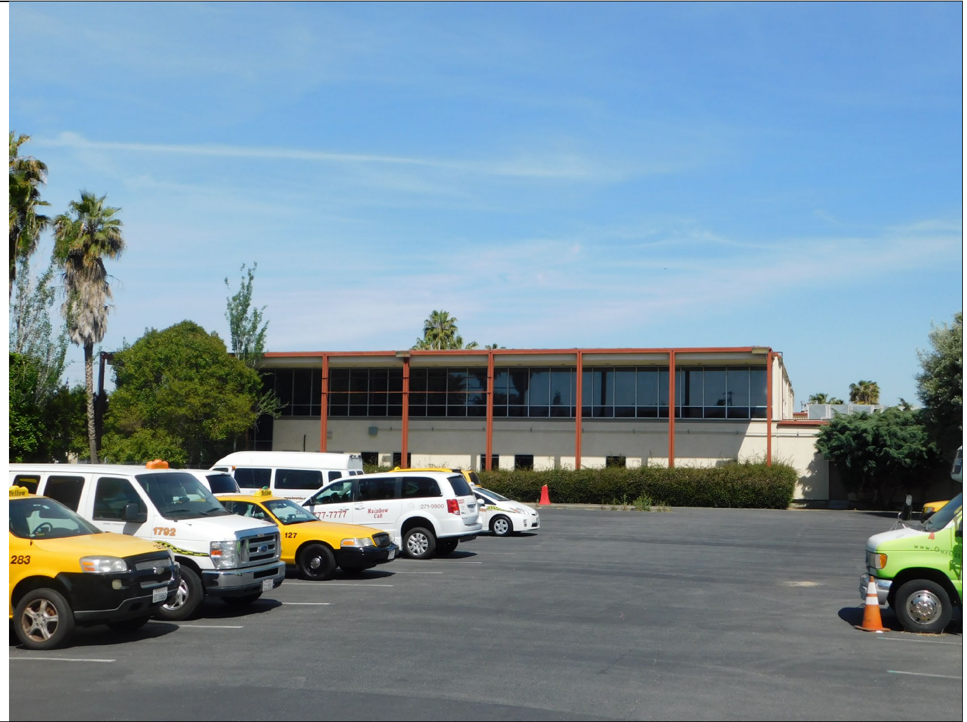
Photograph 5. Building A's south elevation, view looking northwest (IMG 9082)
