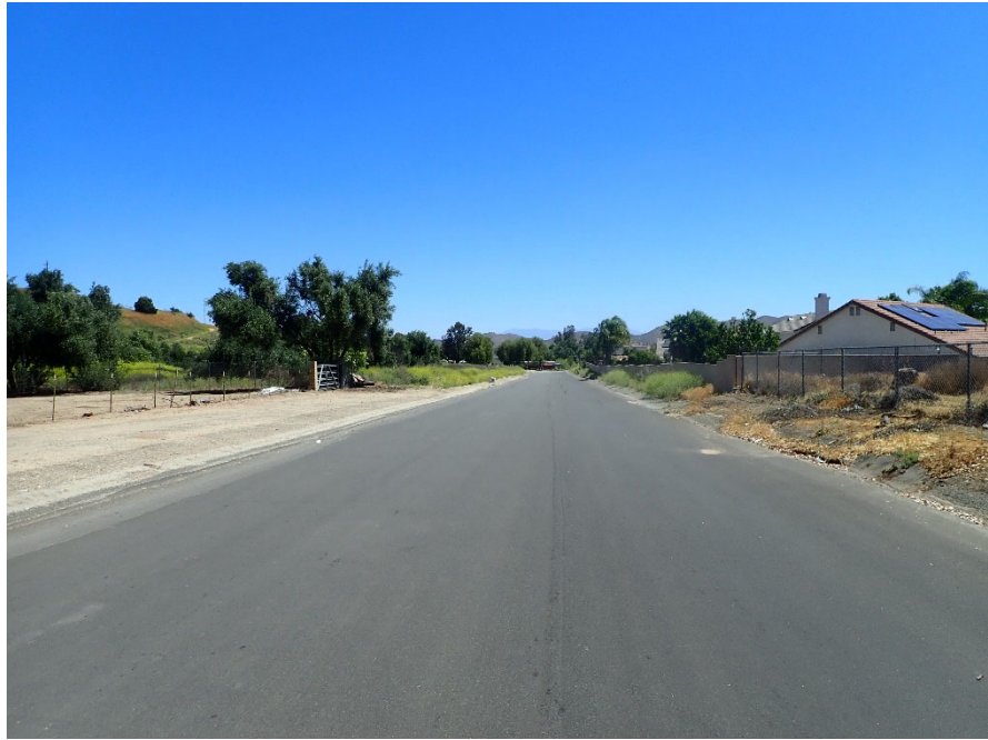
Photograph 11: View northeast along Stoneman Street at the central portion of the site.
