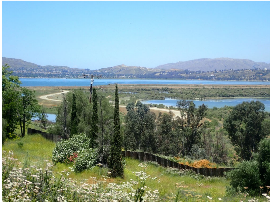
Photograph 25: View north from the top of Rome Hill. Lake Elsinore is viewed in the distance and the Lake Elsinore Levee is centered in the photo. Left of center in the photo is a power pole with a transformer.
