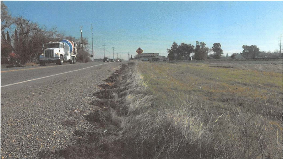
Photo 15: The roadside drainage swale present along the north border of the project area, part of AOI-3. Photo taken along Riego Rd in the northwest corner of the project area, looking east.
