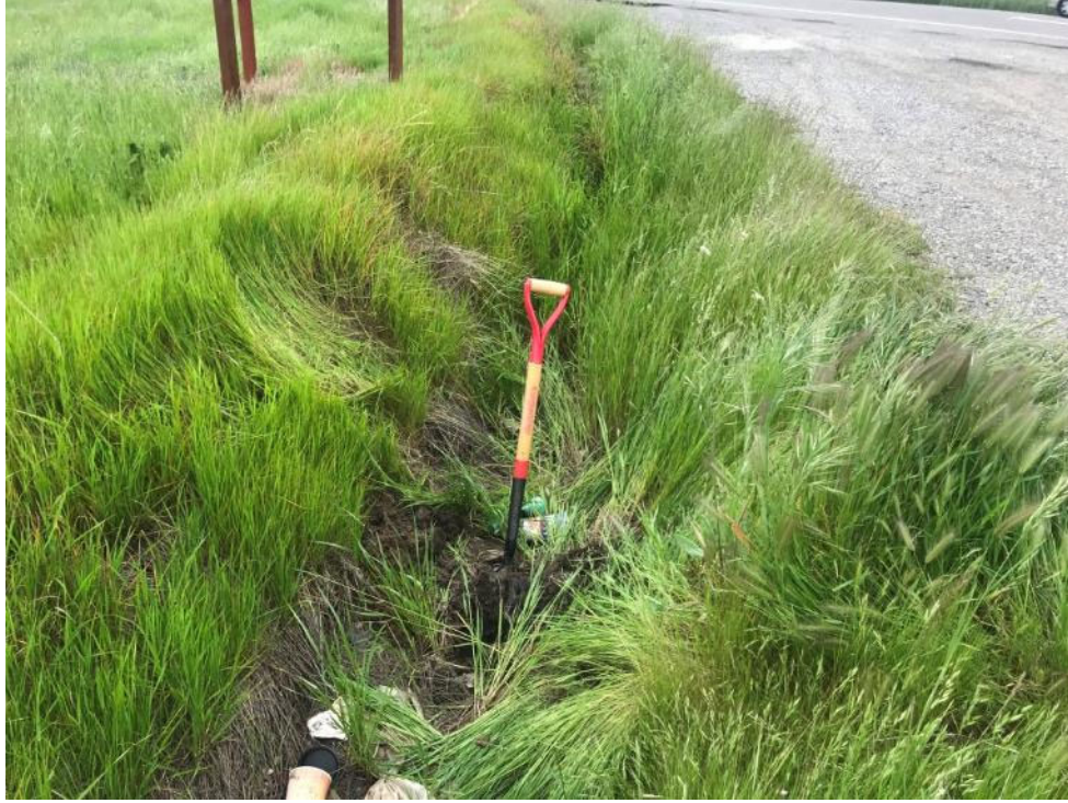
Photo 11: DP-4 taken within a topographic ditch excavated to drain stormwater runoff from the road where the three requisite wetland criteria were observed to be present, taken along the ditch and looking northwest. The portion of the ditch containing the three wetland criteria was mapped as R4EM2-1.
