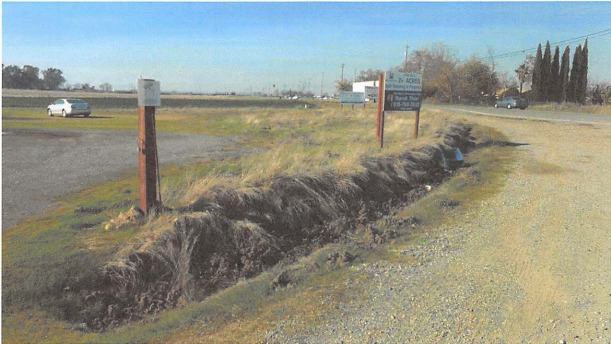
Photo 14: The roadside drainage swale in the northeast corner of the project area, part of AOI-3. Photo taken in the gravel parking area, looking northwest.
