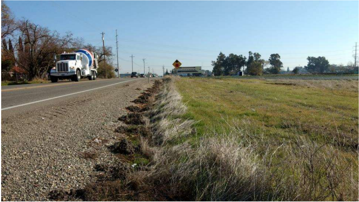
Photo 15: The roadside drainage swale present along the north border of the project area, part of AOI-3. Photo taken along Riego Rd in the northwest corner of the project area, looking east.
