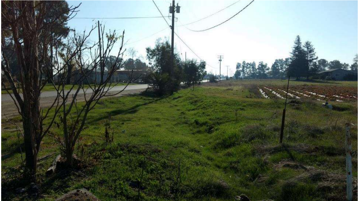
Photo 13: The roadside drainage swale along Pleasant Grove Rd, part of AOI-3. Photo taken from just south of the gravel parking area looking south.
