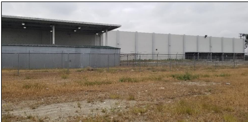
Figure 6. Overview of southern portion of Project Area, view northeast
