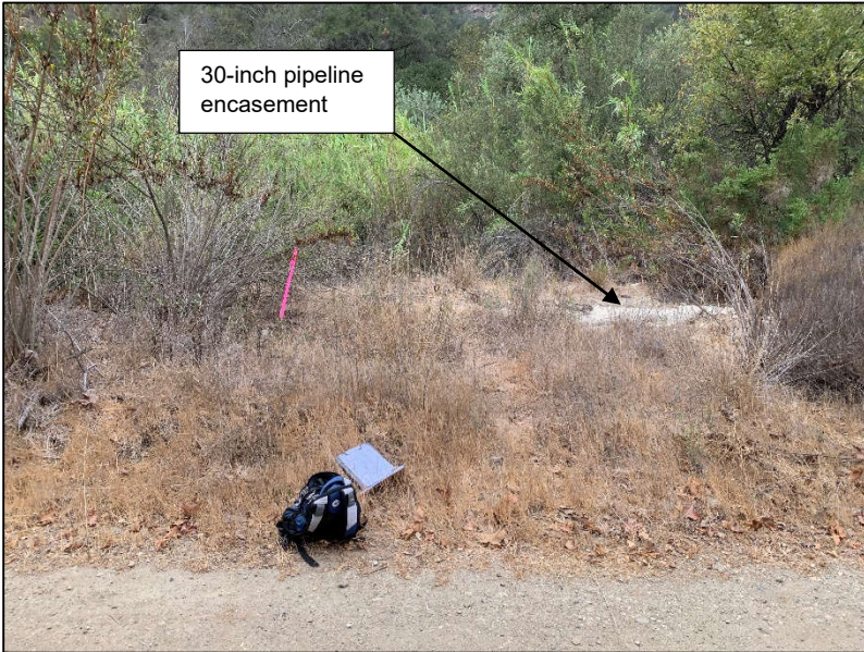
c. Pipe access tee installation area 3 (near pipeline Station 28+00)
