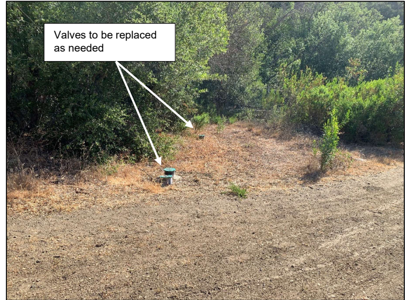
d. Shapell lateral valve replacement work area
