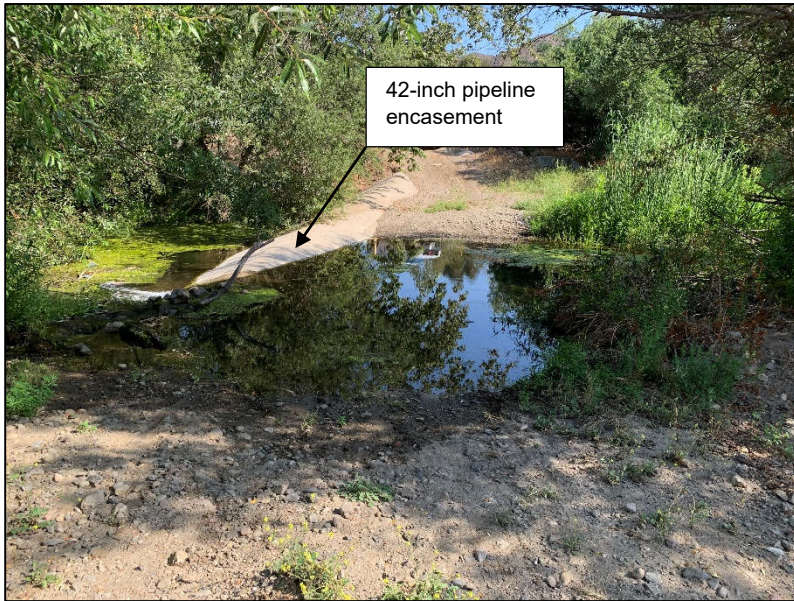
a. Maintenance road creek crossing 1, near Structure W-A, facing north
