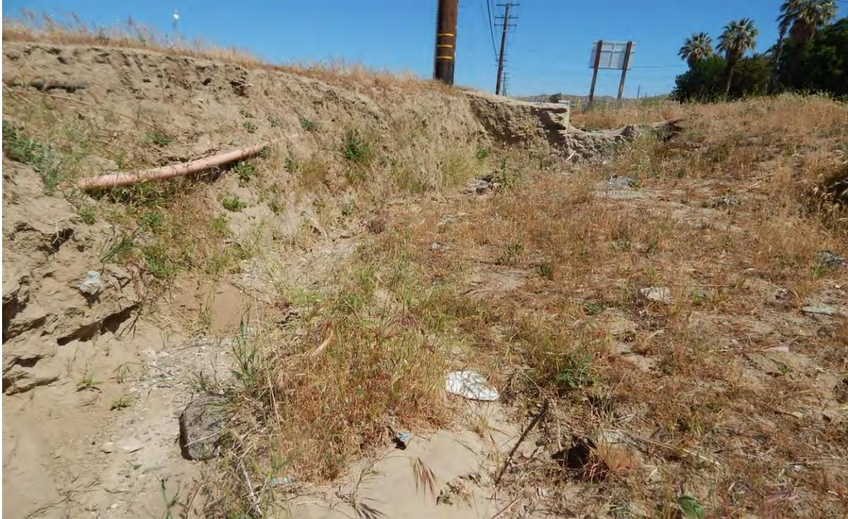
**Photograph 3.** View north and upstream of the roadside drainage channel showing the low-flow channel to the left of a terrace, steep banks, and a drop weir structure in the channel bed in the background.
