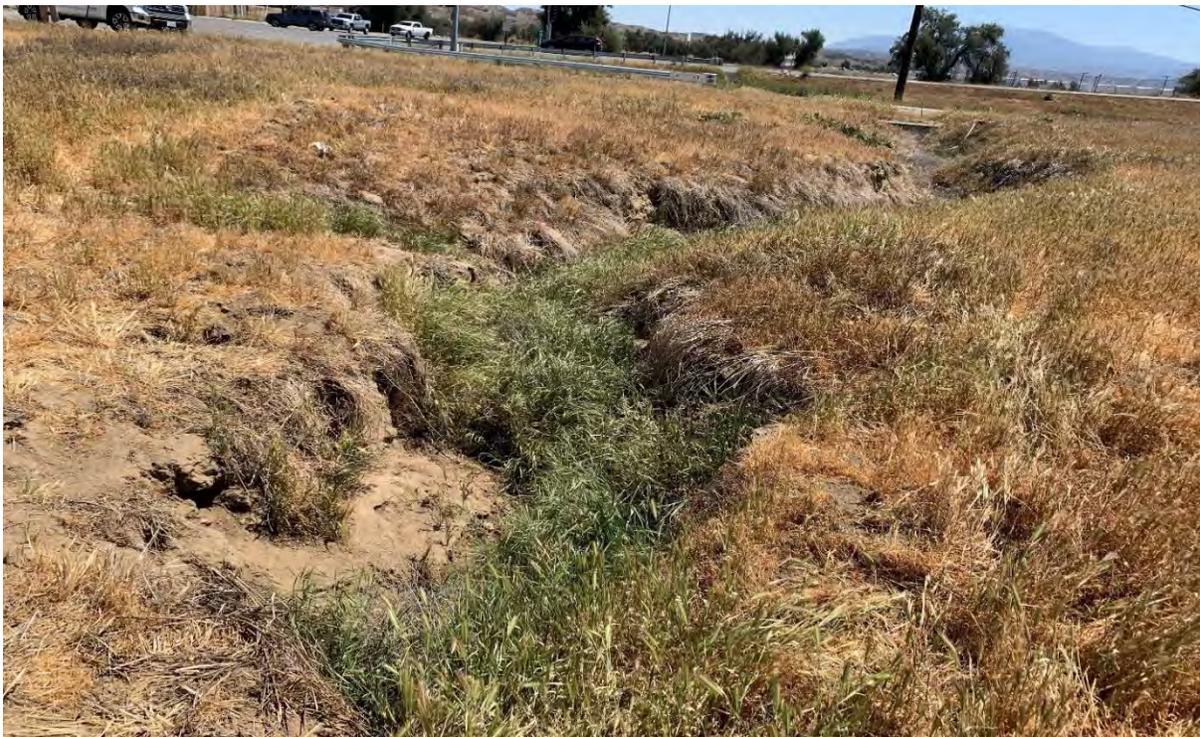
**Photograph 6.** East-facing view toward Spruce Avenue and Redlands Boulevard intersection showing weak water flow evidence and dense annual grasses in the erosional drainage ditch.
