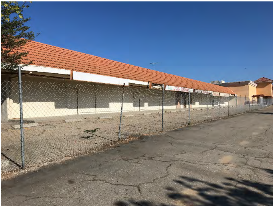
Photo #2 Exterior view of 325 Hampshire Road, Unit B-F.
