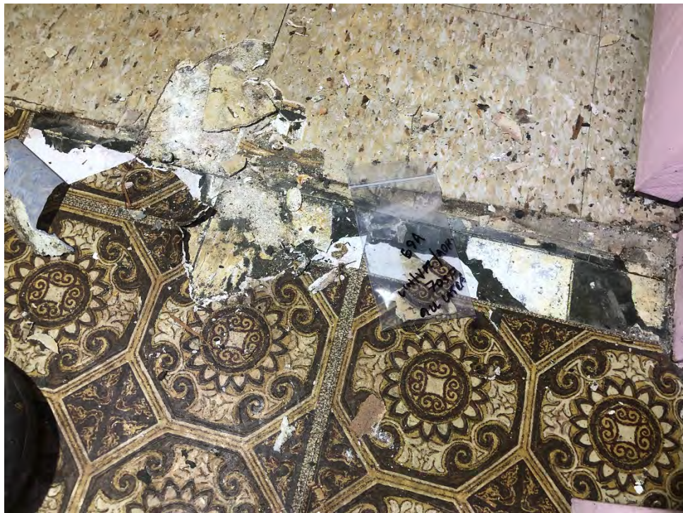
Photo #20 View of multi-layer brown/yellow VFT (HA #69) within 325 Hampshire Road, Unit D. This material is an ACM.
