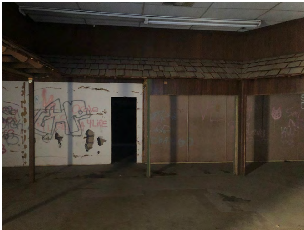
Photo #26 View within 325 Hampshire Road, Unit B.
