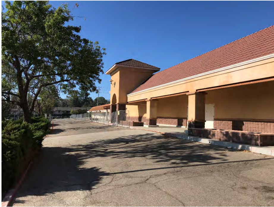
Photo #1 Exterior view of 325 Hampshire Road, Unit A.
