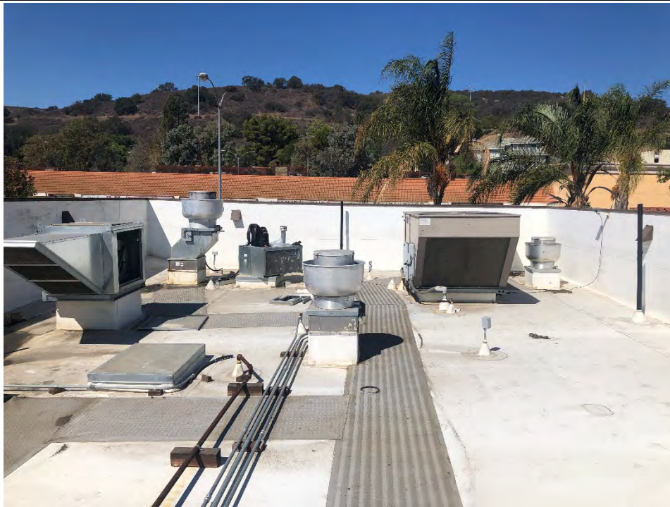
Photo #37 View of across the roof of 391 Hampshire Road, looking west.
