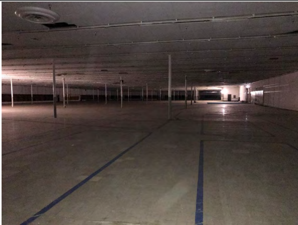
Photo #29 View within the former sales area of 325 Hampshire Road, Unit A.
