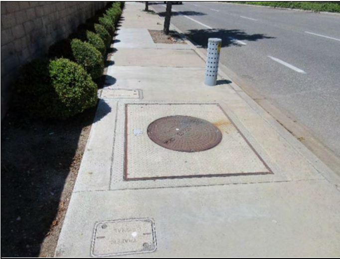
19. View of offsite transformer
