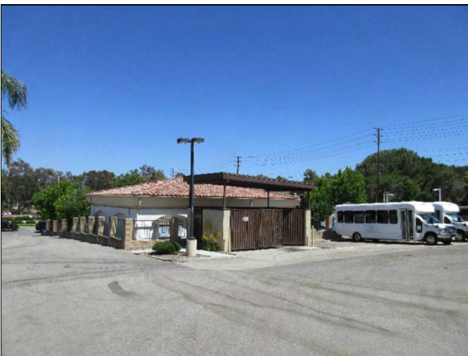
17. View of trash enclosure
