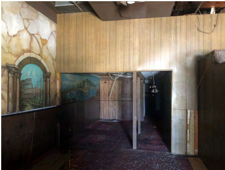
Photo #16 View within 325 Hampshire Road, Unit D.
