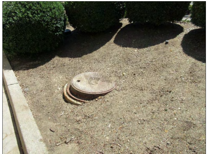
16. View of grease interceptor
