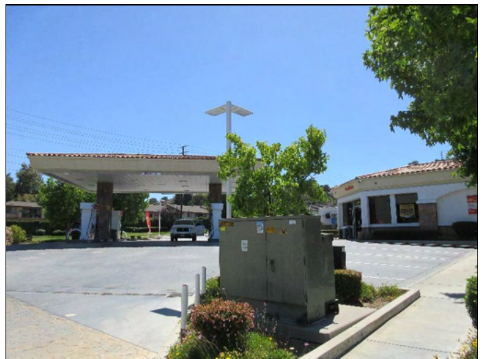
24. View of Shell Station to the southeast
