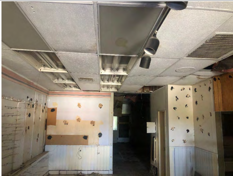
Photo #21 View within 325 Hampshire Road, Unit C.
