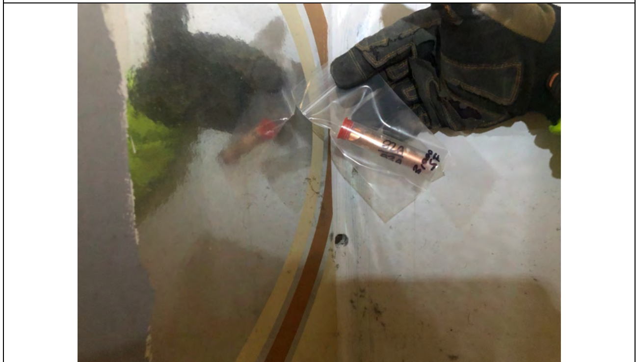
Photo #24 View of wall system within 325 Hampshire Road, Unit C. The joint compound (HA #83) is an ACM.
