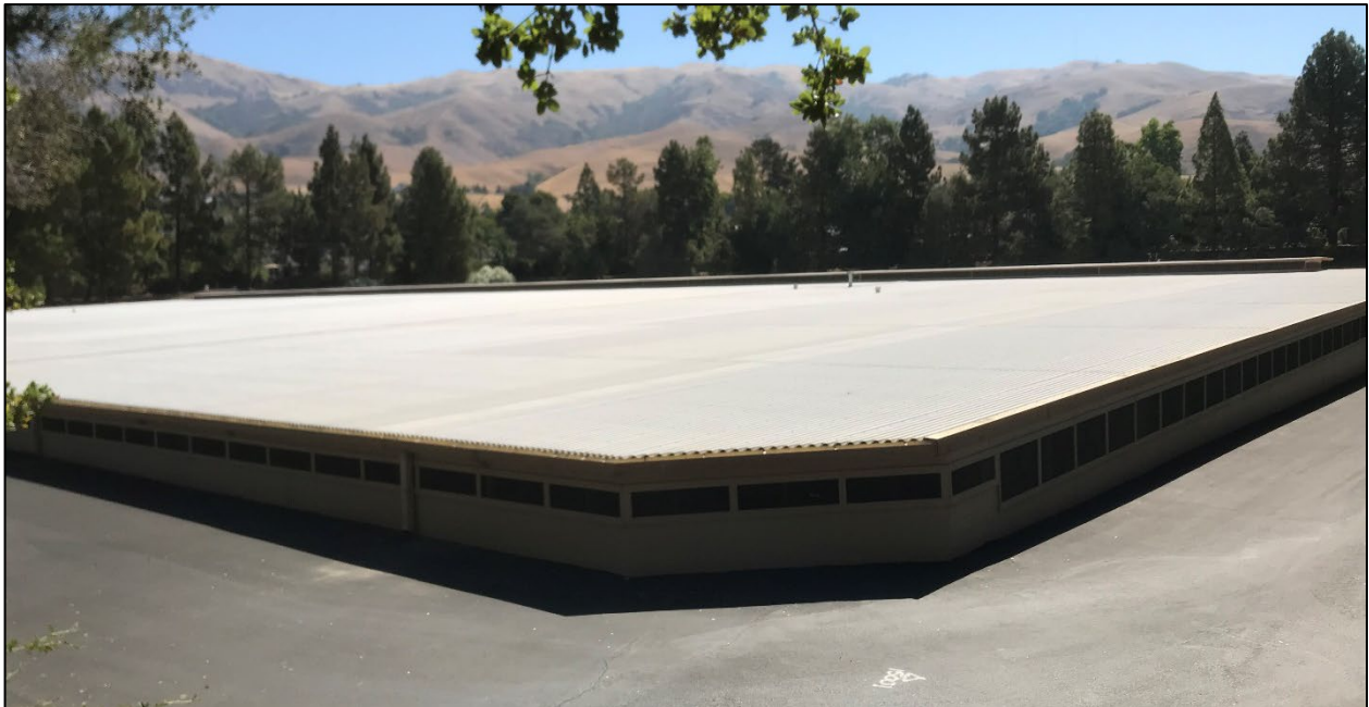
Photograph 2. Photograph depicting Alameda Reservoir, within the developed area of the Study Area.
