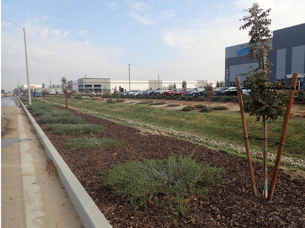
Figure 13 – New sections of irrigated landscaping and paved curb on south side of Riggin Avenue near Kelsey Street (View East)
