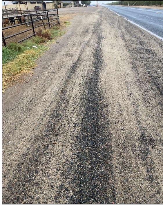
Figure 4-1 Road aggregate on south side of West Riggin Ave, facing west.
