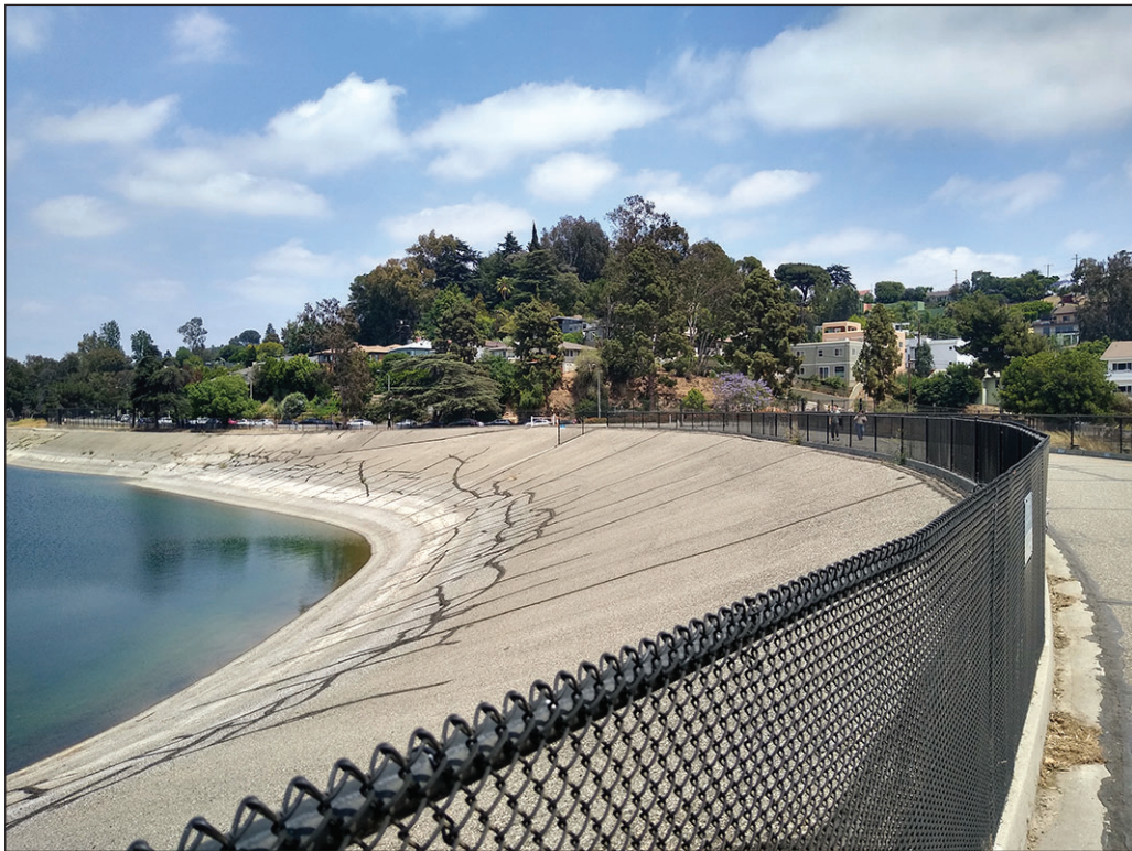
Looking northeast on Silver Lake Dam Pedestrian Path
