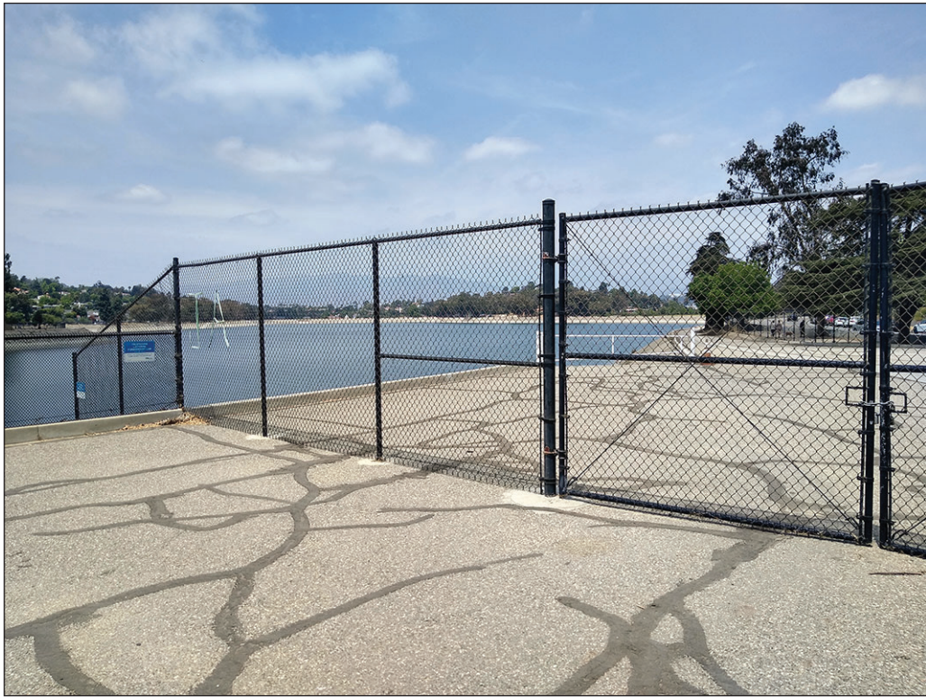
Looking north at southeast corner of Silver Lake Reservoir
