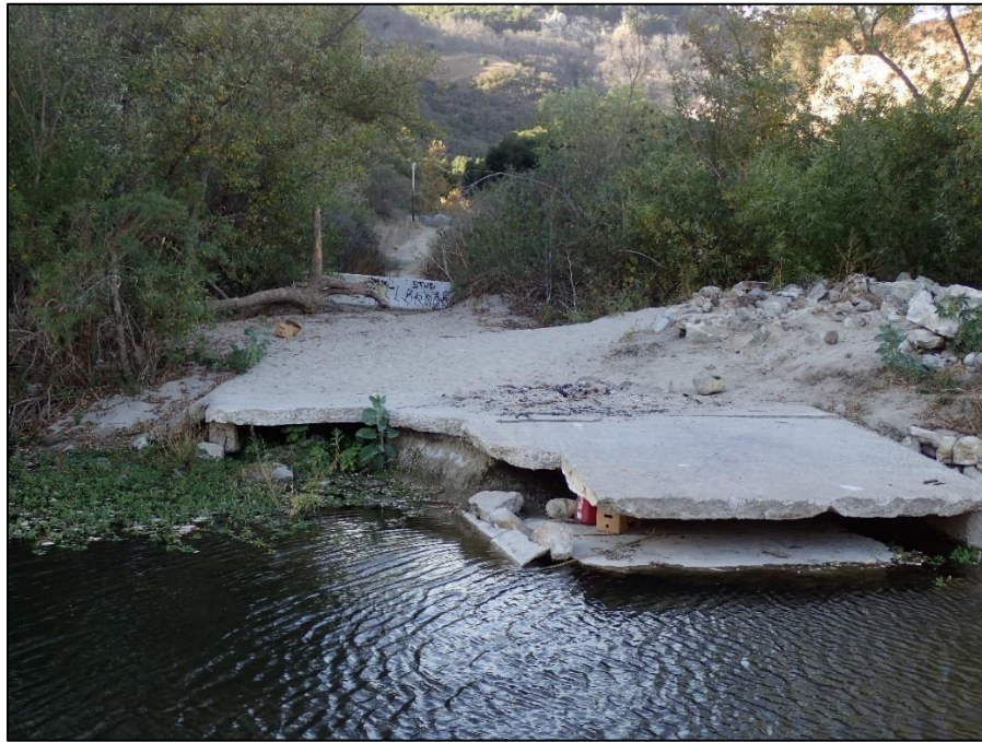
Figure 1-10. Old Concrete Ford Crossing (North Side, Partially Removed)
