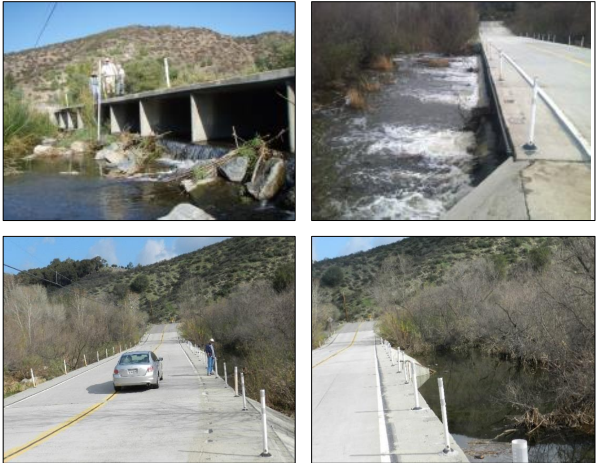
Figure 1-2. Existing Sandia Creek Drive Bridge
