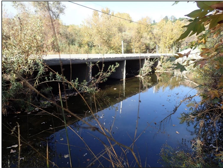
Figure 1-6. Sandia Creek Drive Bridge (Upstream Face)
