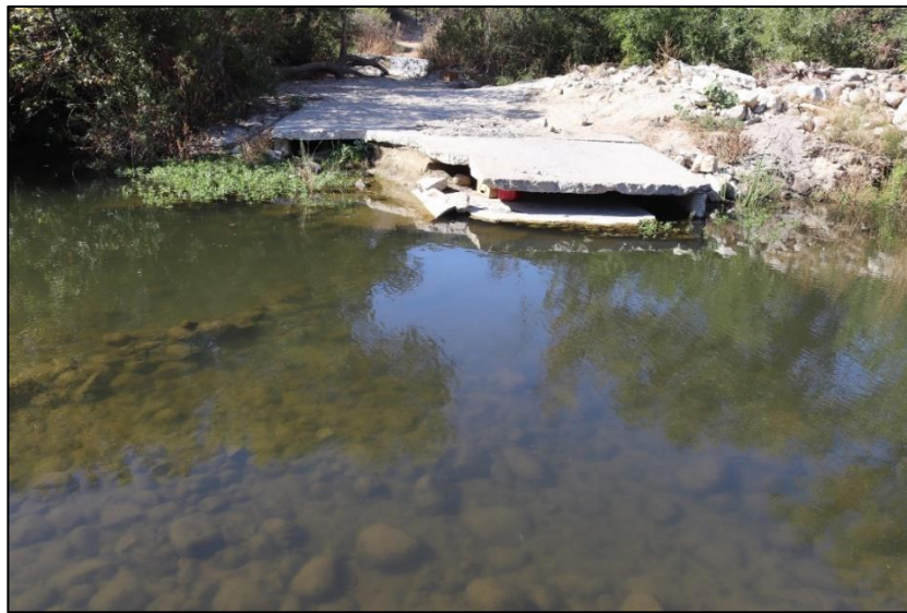
Figure 2-5. Partially Removed Ford Crossing
