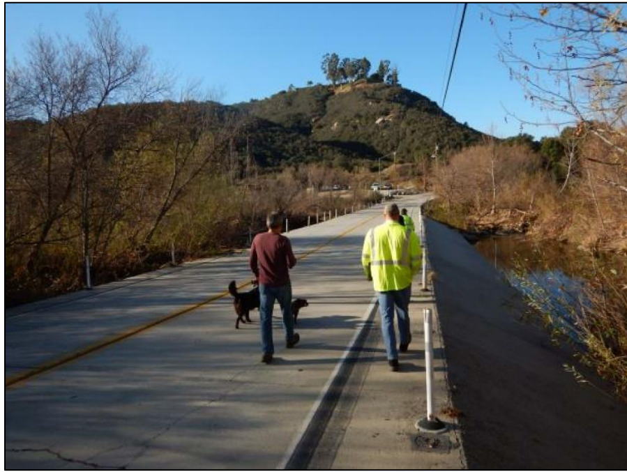
Figure 1-8. Sandia Creek Drive, Facing South toward Parking Lot
