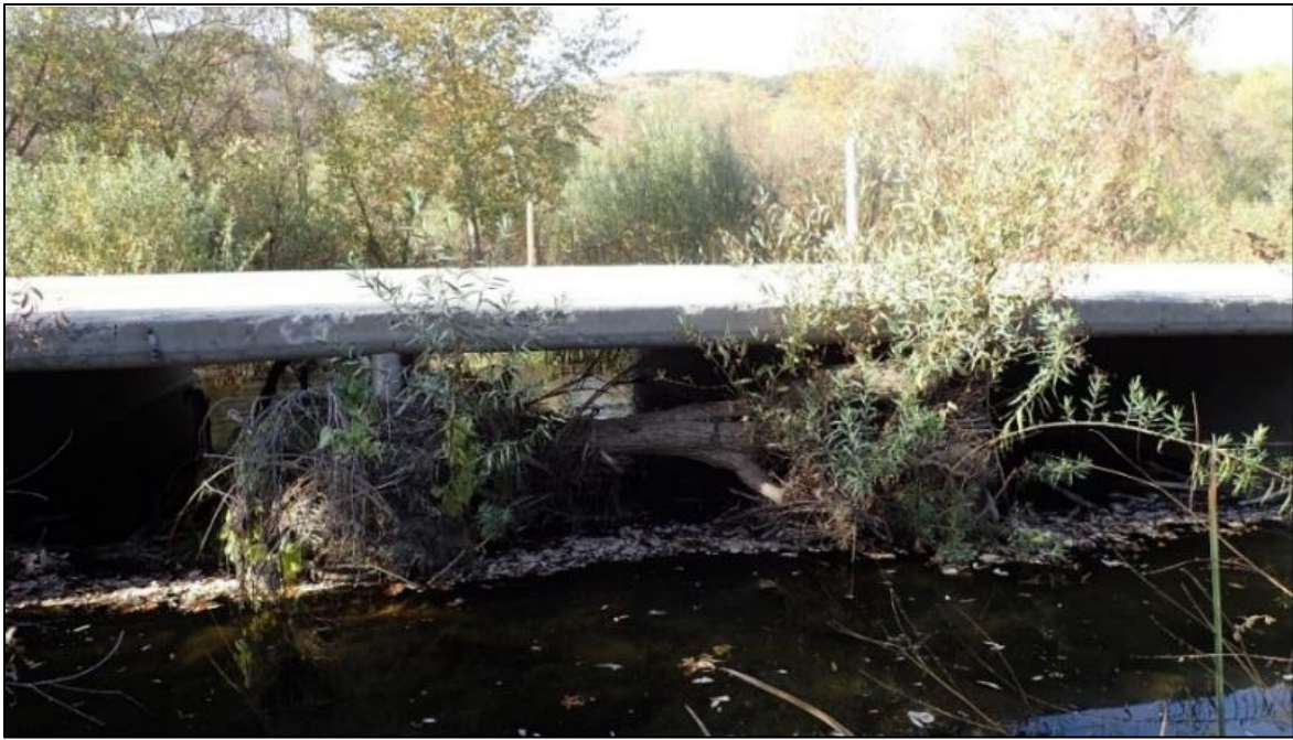
Figure 2-1. Sandia Creek Drive Bridge (Upstream Face)
