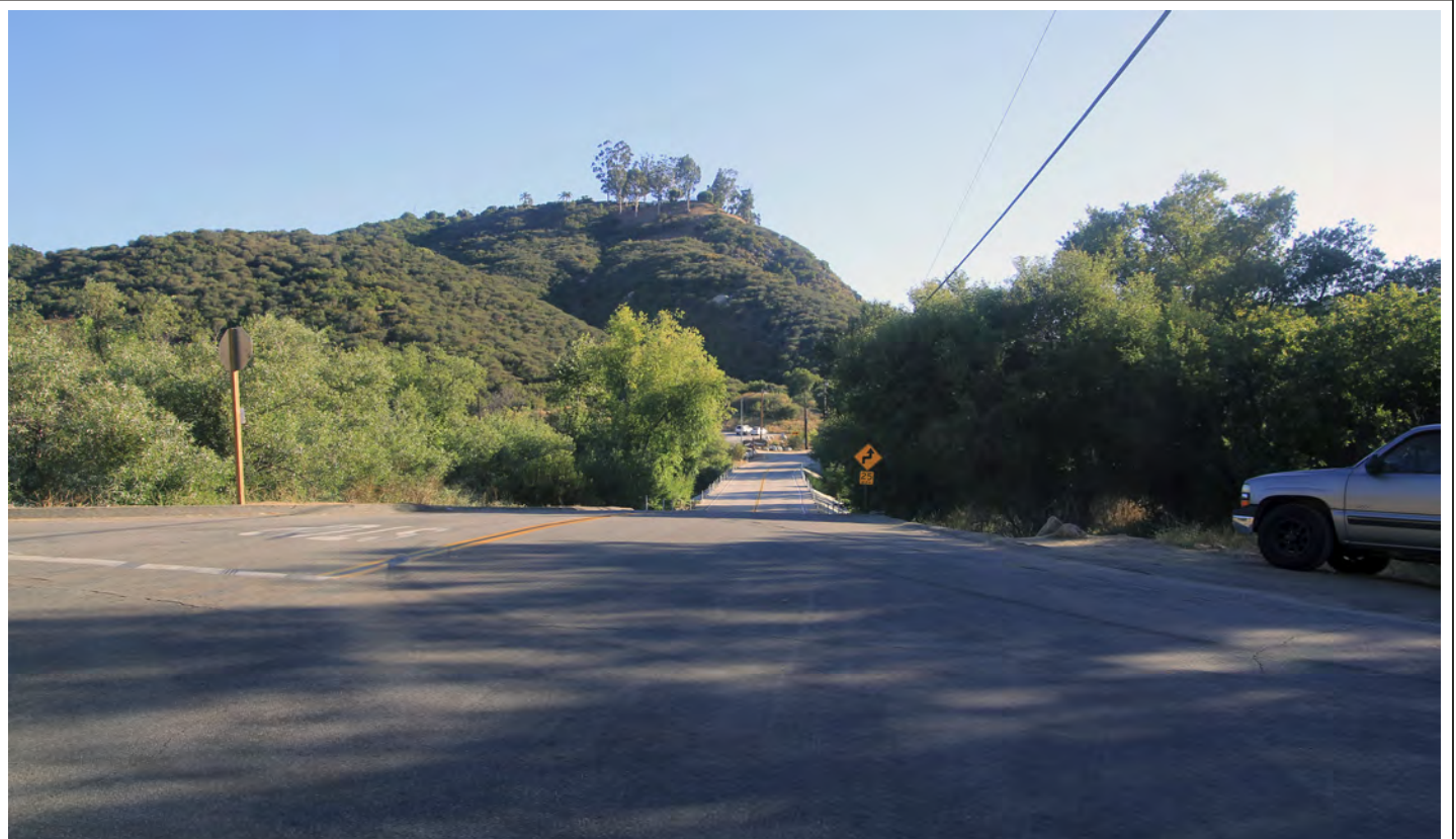
Existing View from Rock Mountain Drive/Sandia Creek Drive intersection towards existing bridge
