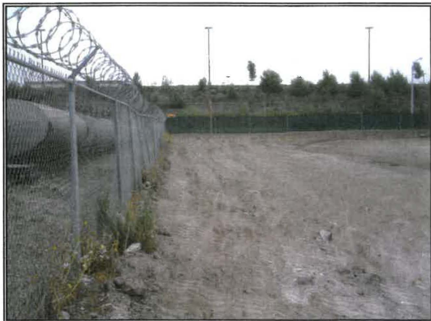
Plate 2. Facing the southwest corner of the proposed project site.
