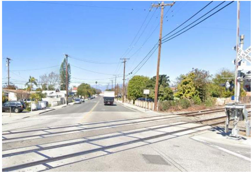
Railroad crossing at Orr and Day Road
