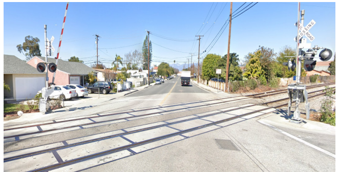
Railroad crossing at Orr and Day Road
