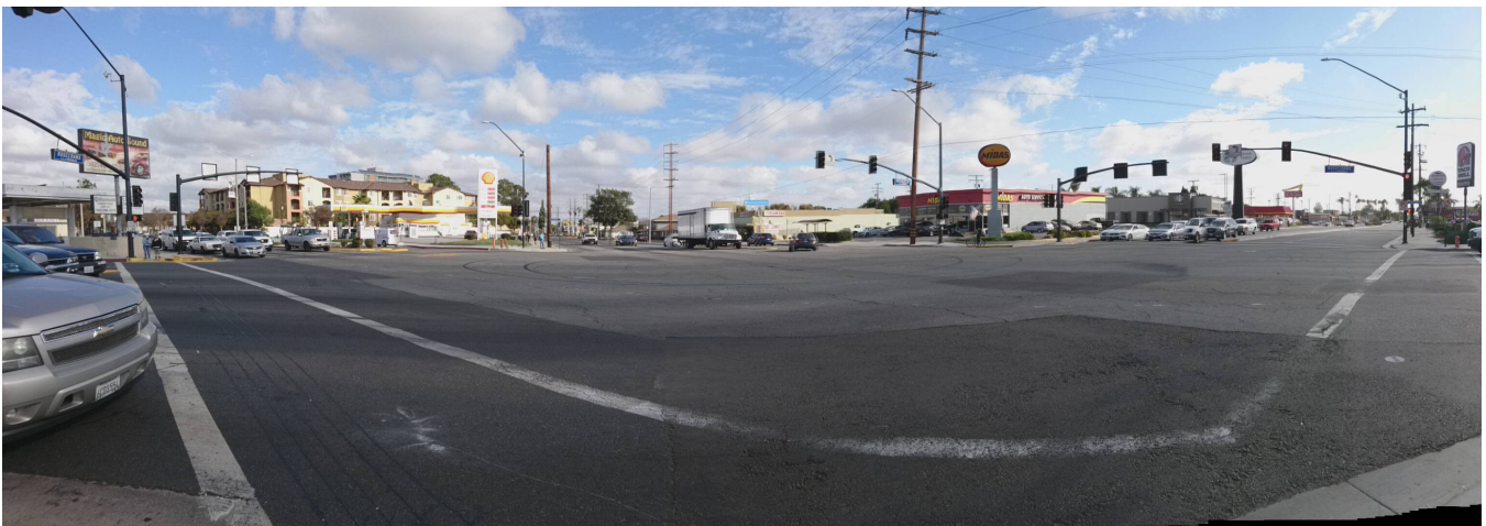
Intersection of Pioneer Boulevard, Rosecrans Avenue, and San Antonio Drive
