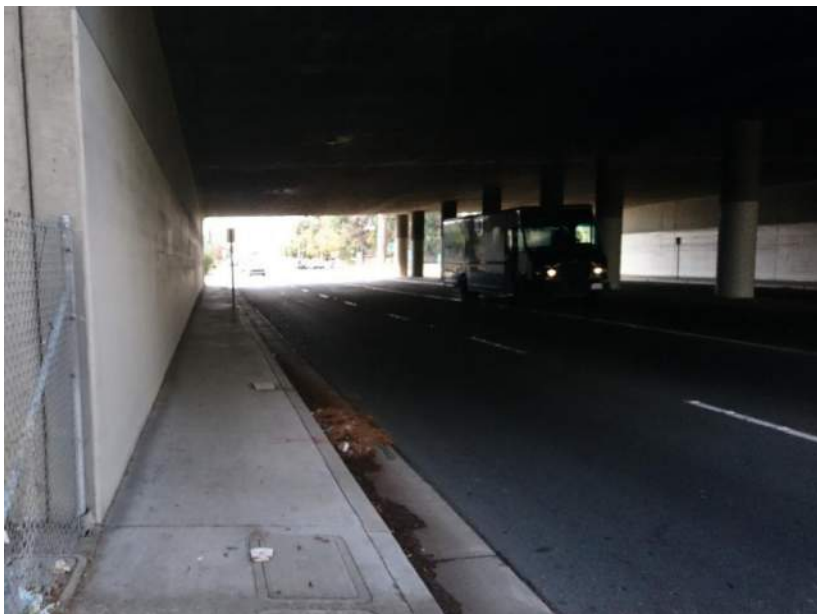
I-605 overpass at Rosecrans Avenue
