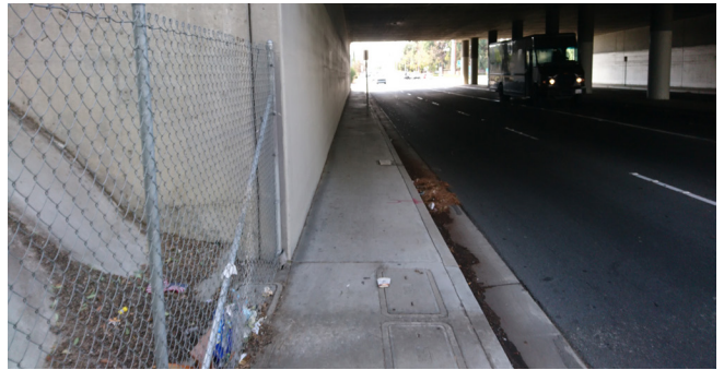
I-605 overpass at Rosecrans Avenue
