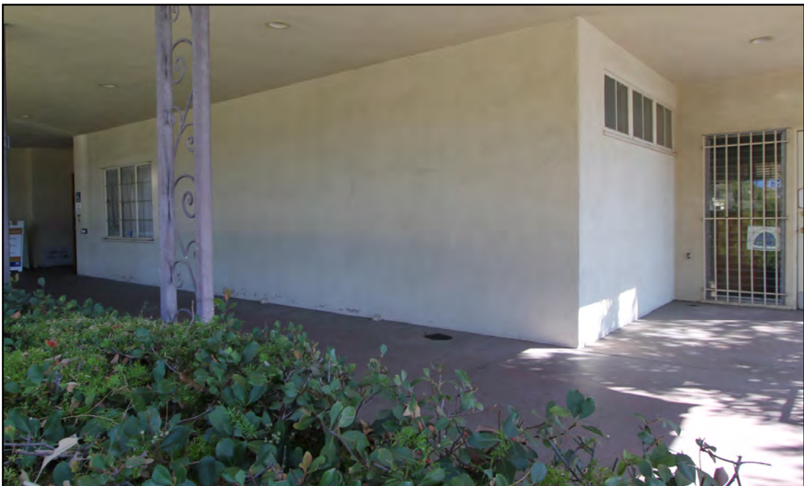
Image 21: San Marino Center, north elevation, view southeast, note entry porch (Chattel, 2021)
