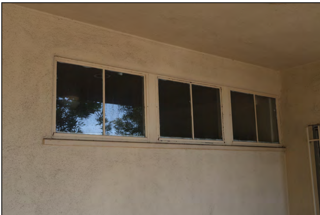
Image 23: Detail of steel sash windows on west elevation, view southeast (Chattel, 2021)
