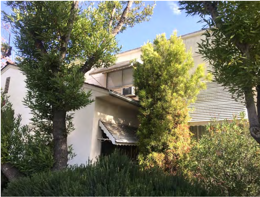
Photograph 5: 1800 Huntington Drive, west elevation, camera facing northeast, January 19, 2021.
