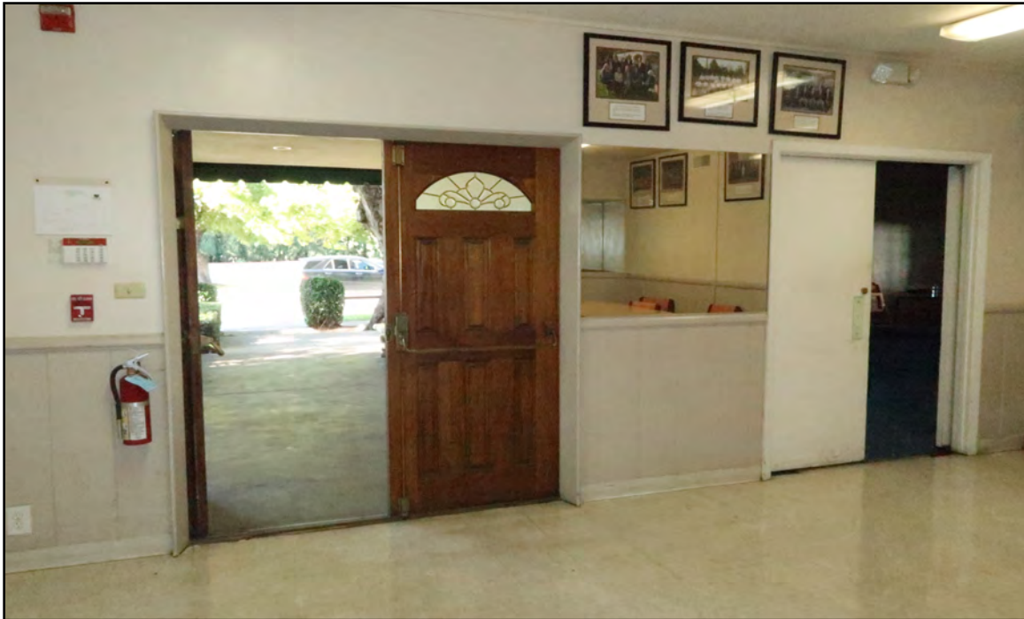
Image 26: View of entry double doors from interior, view northeast (Chattel, 2021)
