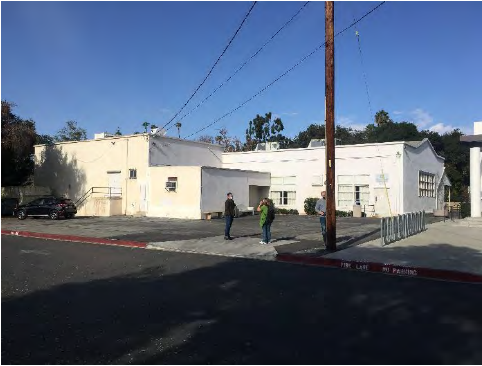
Photograph 3: 1800 Huntington Drive, south and east elevations, camera facing northwest, January 19, 2021.
