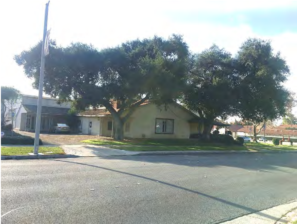
Photograph 2: 1800 Huntington Drive, north and east elevations, 1958 addition center frame, camera facing southwest, January 19, 2021.
