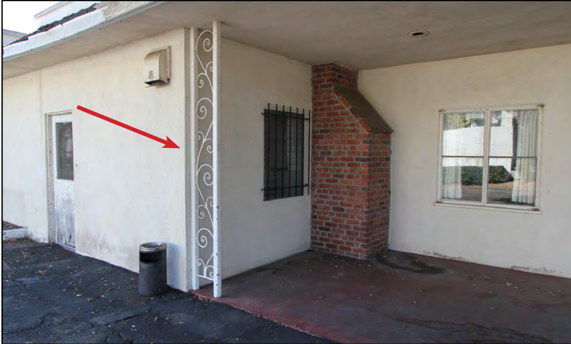
Image 7: San Marino Center, east elevation (far left) and north elevation (center), note brick chimney bisected by east storage addition and ornamental ironwork (Chattel, 2021)
