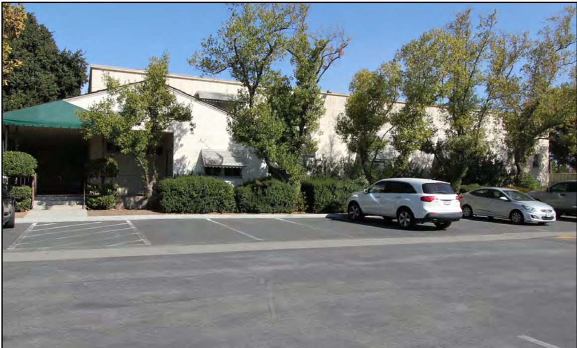
Image 19: San Marino Center, west elevation, view east (Chattel, 2021)
