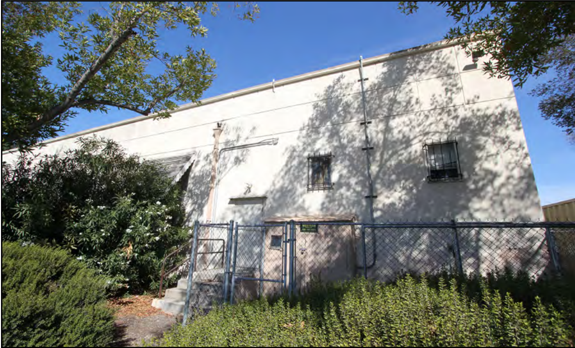
Image 18: San Marino Center, west elevation, view east (Chattel, 2021)
