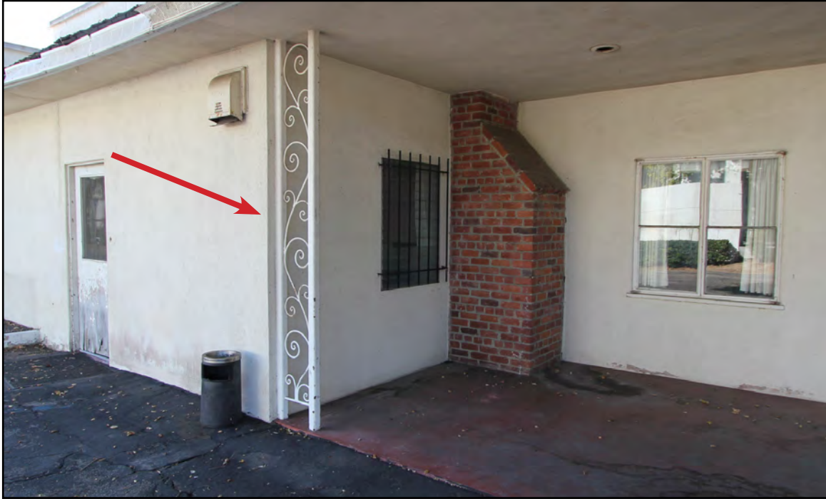
Image 7: San Marino Center, east elevation (far left) and north elevation (center), note brick chimney bisected by east storage addition and ornamental ironwork (Chattel, 2021)
