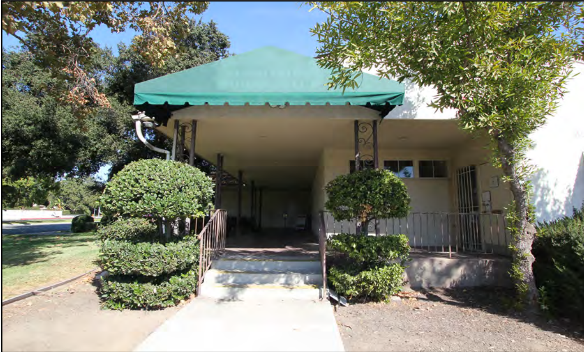
Image 20: San Marino Center, west elevation, view east (Chattel, 2021)
