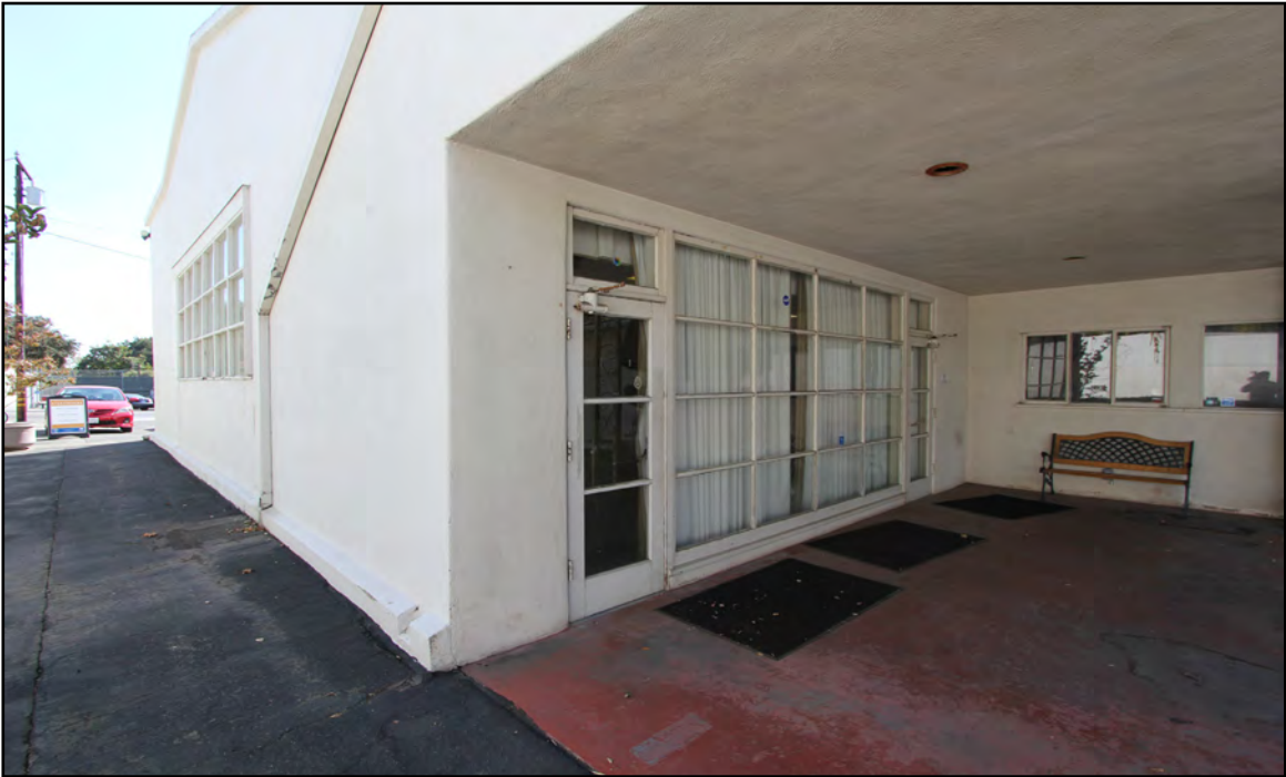
Image 10: San Marino Center, east elevation, view southwest (Chattel, 2021)
