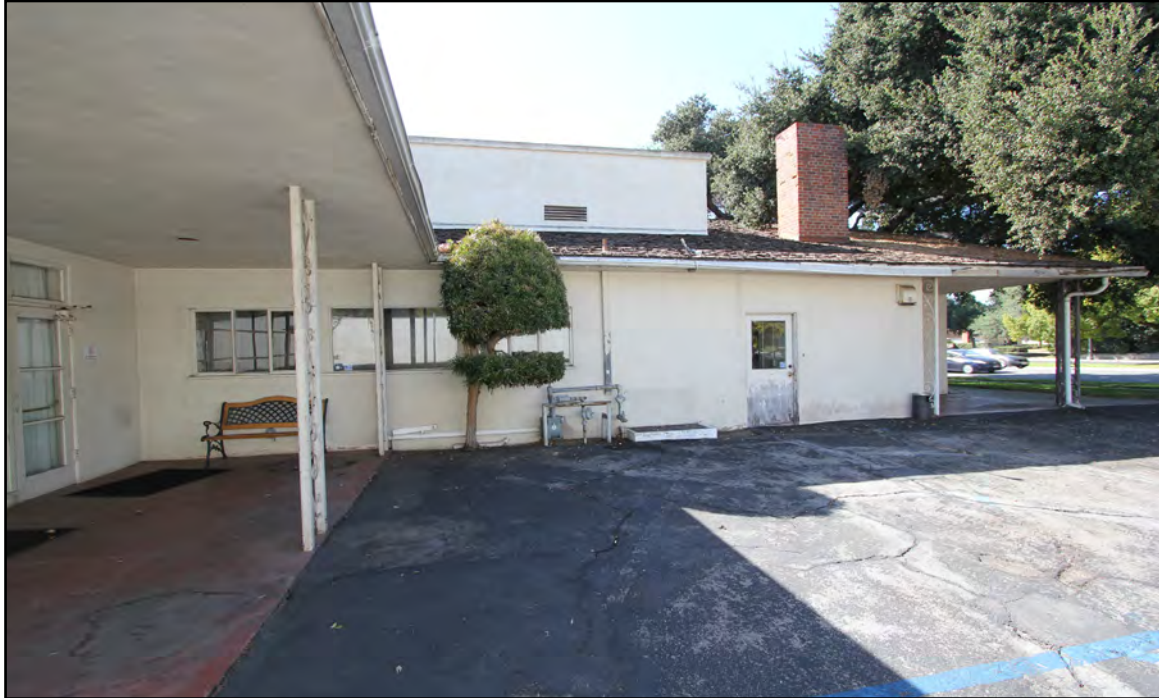
Image 8: San Marino Center, north elevation (left) and east elevation (right), note recessed porch with original paving painted red, view west (Chattel, 2021)
