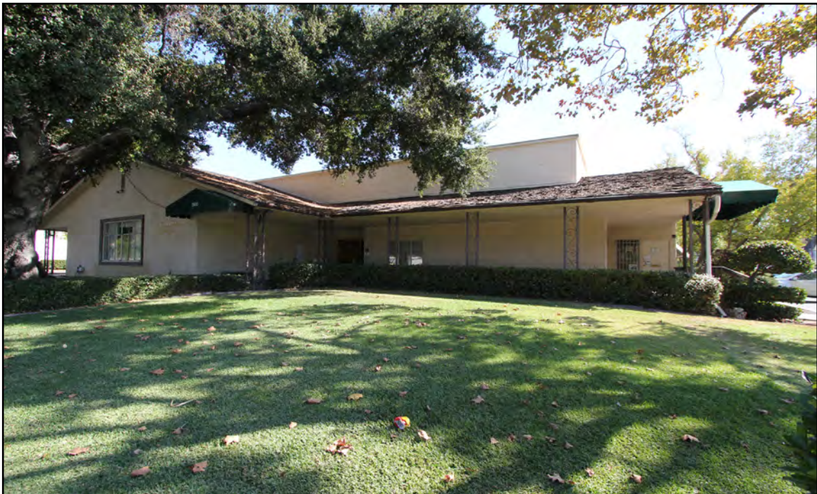
Image 2: San Marino Center, north elevation, view southeast (Chattel, 2021)
