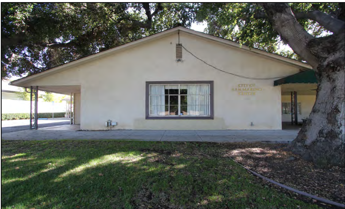
Image 4: San Marino Center, north elevation, view south (Chattel, 2021)
