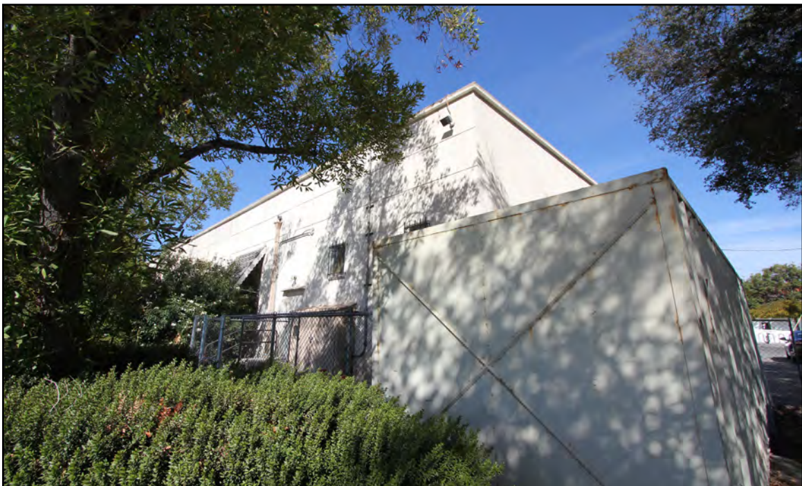
Image 17: San Marino Center, west elevation, view northeast (Chattel, 2021)
