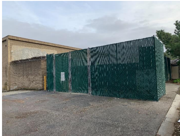
Figure 14: North façade, looking southeast.
