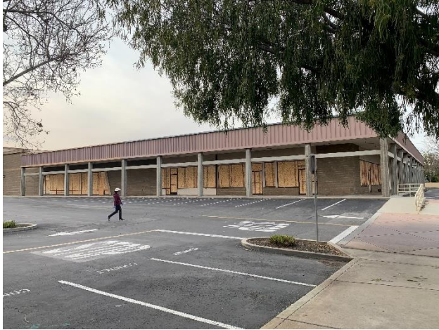
Figure 4: East segment of south façade, looking northeast.
