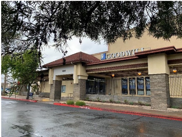
Figure 6: South facade, view northwest.
