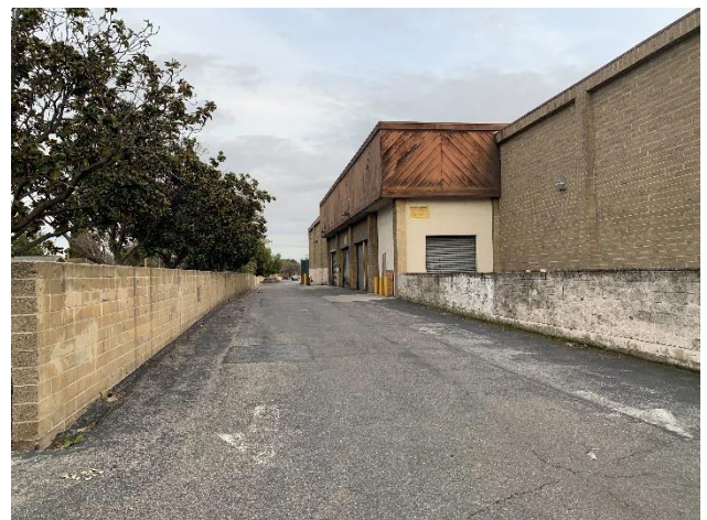
Figure 13: North façade, looking southeast.
