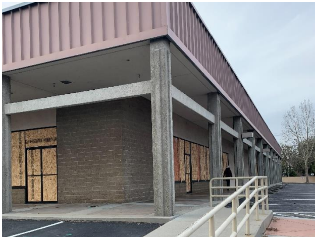
Figure 6: Southeast corner of building, looking north.
