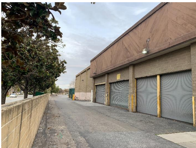
Figure 12: North façade, looking southeast.
