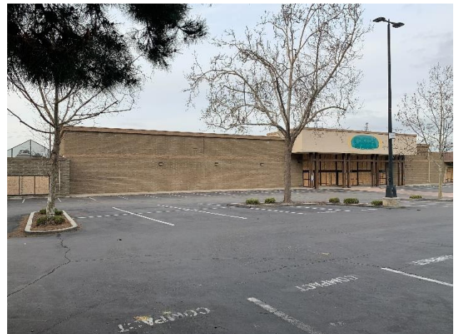
Figure 3: Central segment of south façade, looking northeast.
