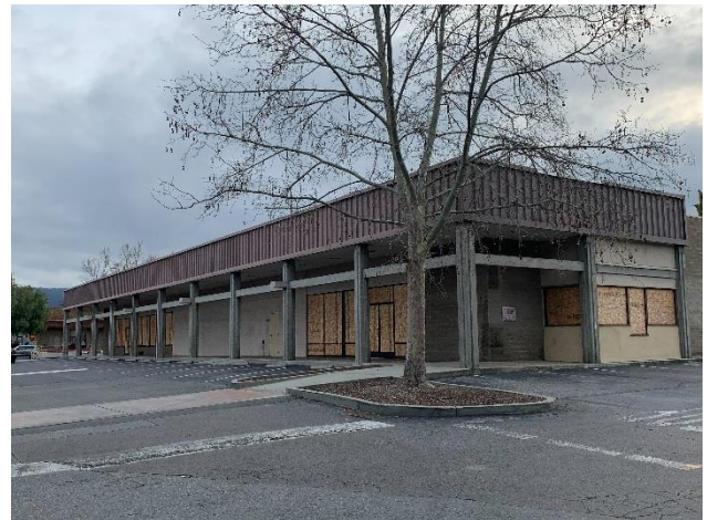
Figure 7: East façade, looking southwest.
