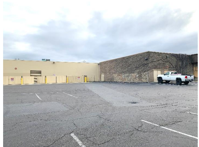
Figure 15: West portion of north façade, view southwest.
