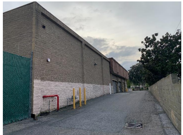
Figure 11: North façade, looking southwest.
