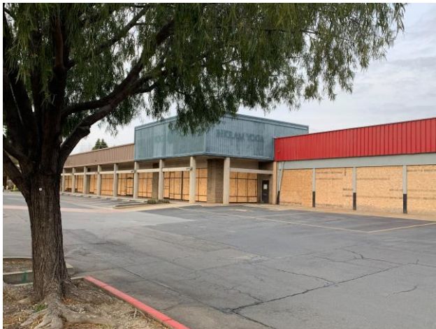
Figure 10: View northeast toward central portion of west façade.
