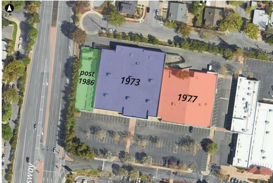
Figure 19. Construction sequence of 5365 Prospect Road. Source: Google Earth, 2022, edited by Page & Turnbull.
