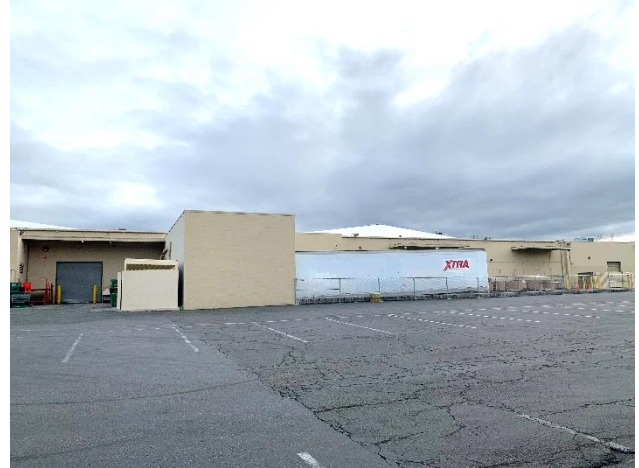
Figure 13: Central portion of north façade, view southwest.
