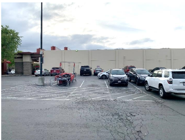
Figure 16: East façade, looking west.
