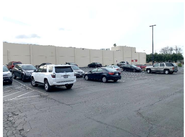
Figure 17: East façade, looking northeast.
