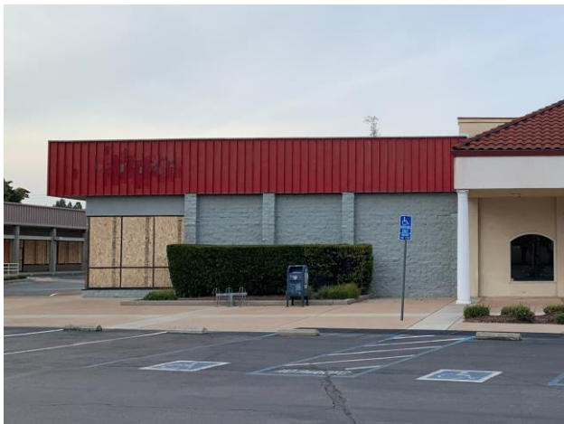
Figure 2: South façade west corner, looking north.
