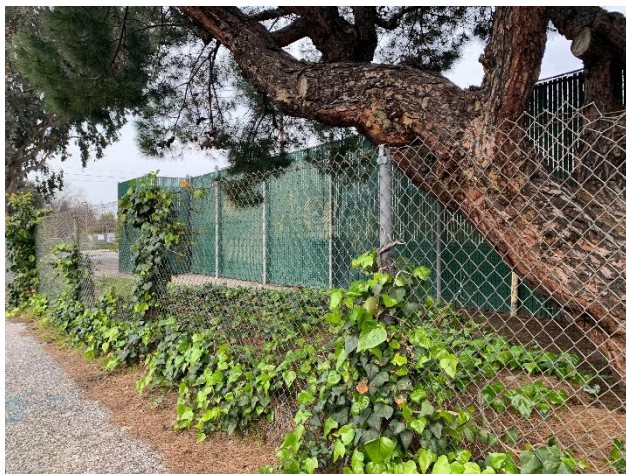
Figure 15: West façade, looking northeast.
