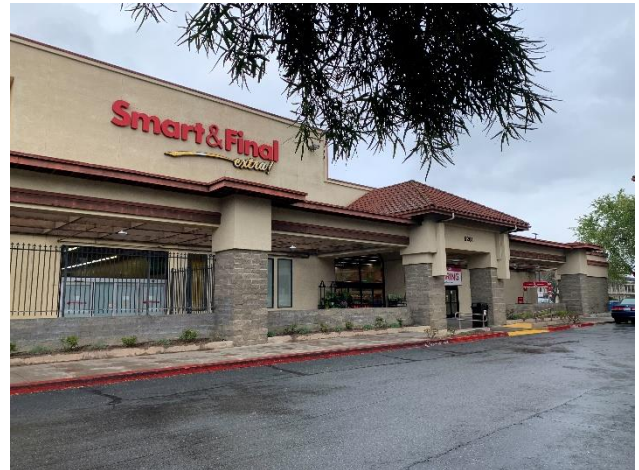
Figure 7: South facade, view northeast.
