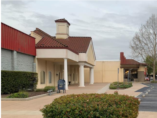
Figure 4. South facade, view east.
