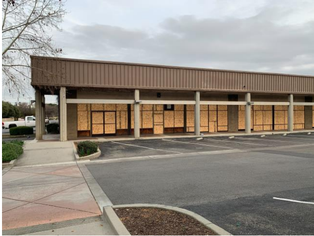
Figure 8: North end of west façade, view east.
