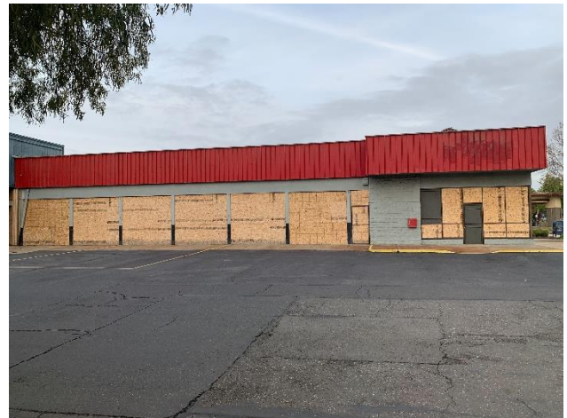
Figure 11: South end of west façade, view east.
