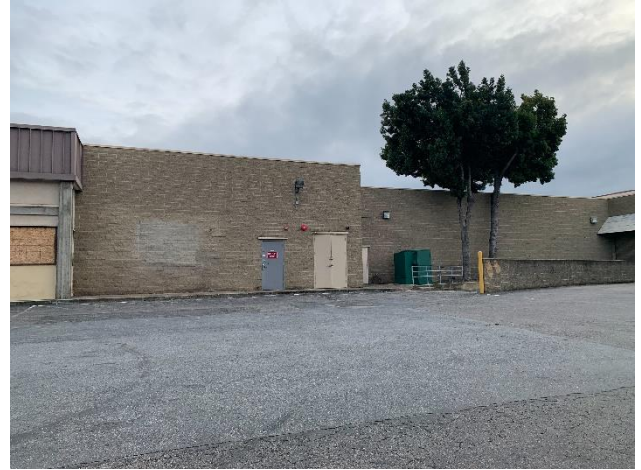
Figure 9: North façade, looking south.
