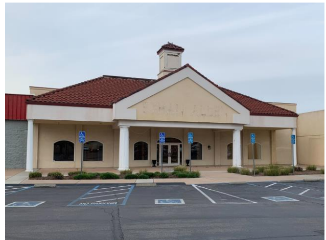
Figure 3: South façade, looking northeast.
