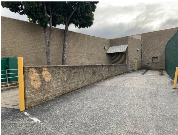
Figure 10: North façade, looking southwest.
