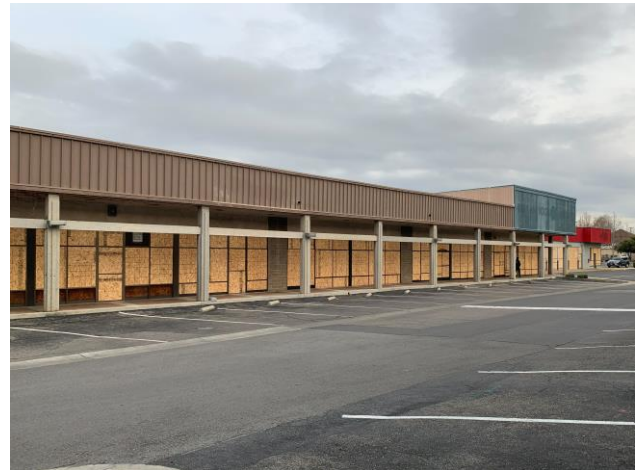
Figure 9: View southeast along west façade.
