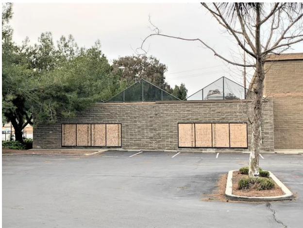
Figure 2: West segment of south façade, looking north.
