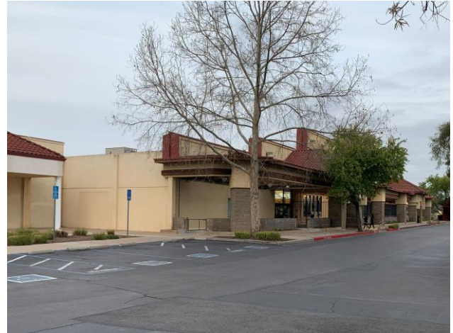
Figure 5. South facade, view northeast.
