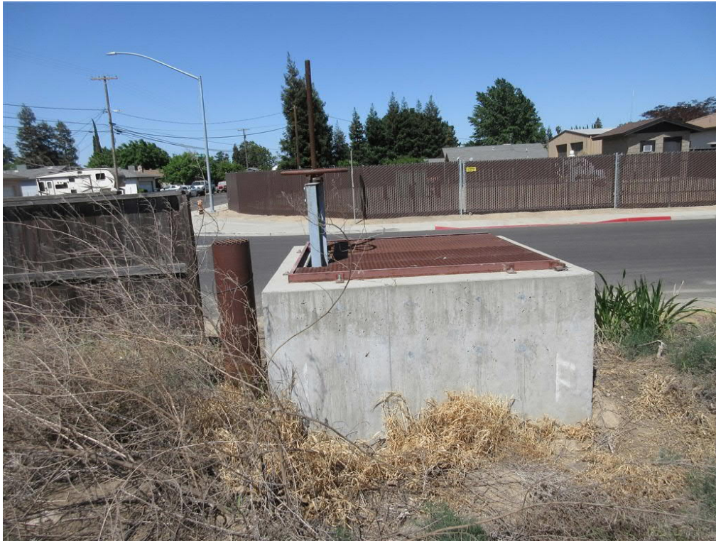
Photo 9: View of irrigation system access/valve/vent features located in the southwestern portion of the subject site.
