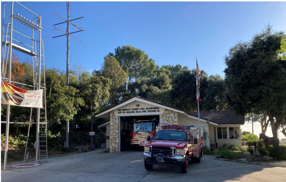
Los Angeles County Fire Station No. 56
