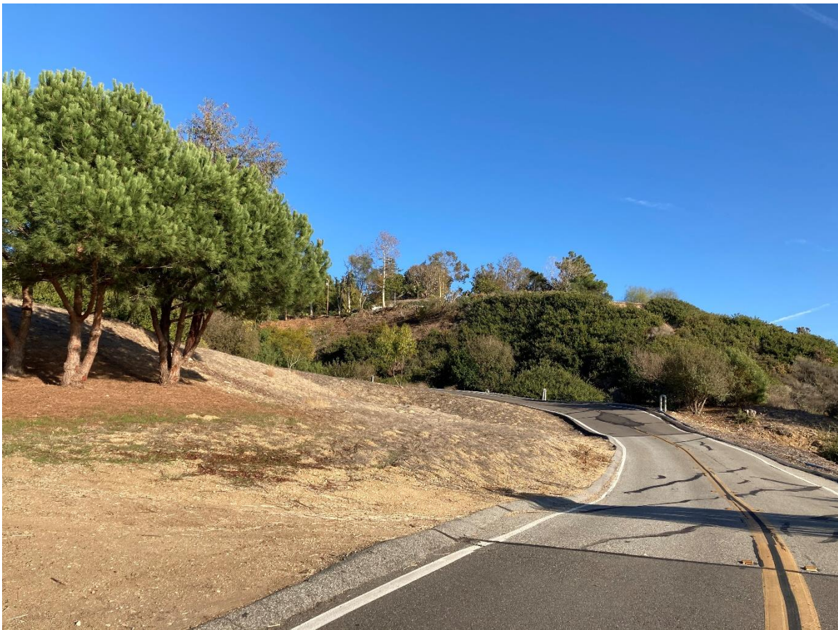
Portuguese Bend Road, south of Crest Road
