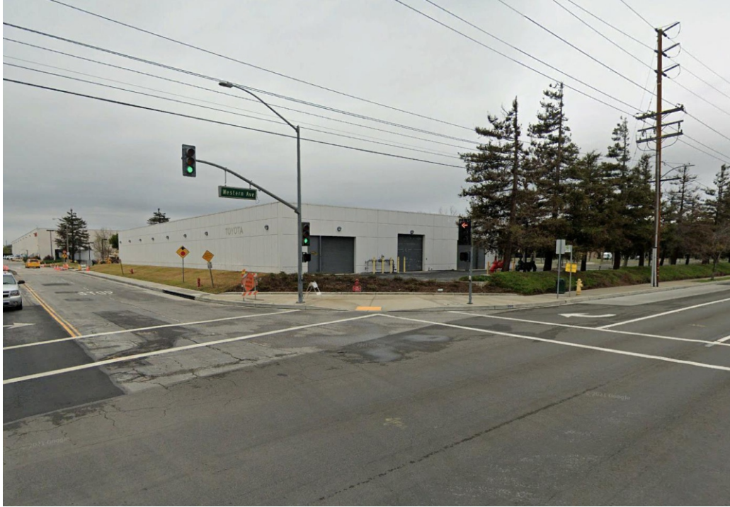
Photo 3: View from the intersection of Western Avenue/195th Street.
