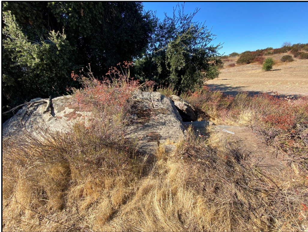
Plate 4.5–1: Overview of BMF A at Site Temp-3, facing northwest.
