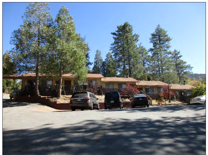
6. Eastern motel building on the subject property
