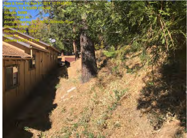
Looking north along the back (east side) of existing units on Parcel 028 (11.01.2019).
