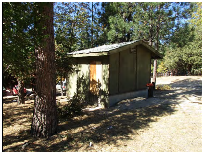
18. Existing inactive water pump house and active water well
