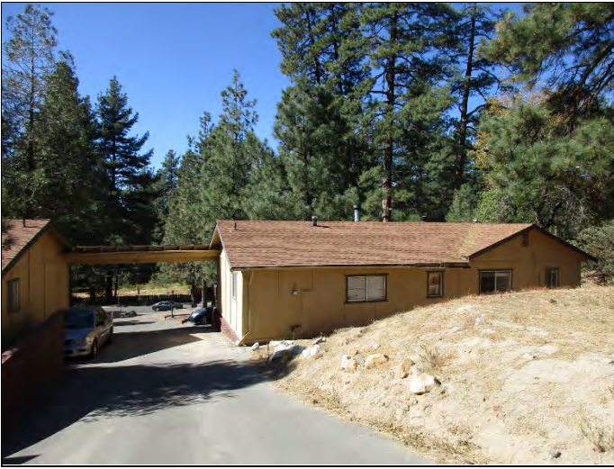
13. Driveway commencing from CA Highway 243 through the subject property
