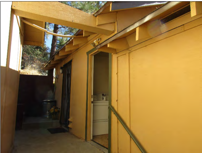
9. Entrance to the laundry room
