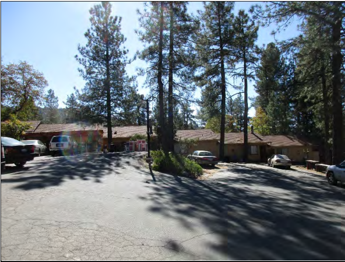
7. Southern motel building on the subject property
