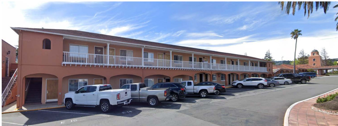
Photo 4. View of Building 100 facing southeast. The replacement railing was likely added ca. 1950 when Buildings 200 and 300 were built. Compare to Figures 4 through 6. Source: Google Earth 2019.
