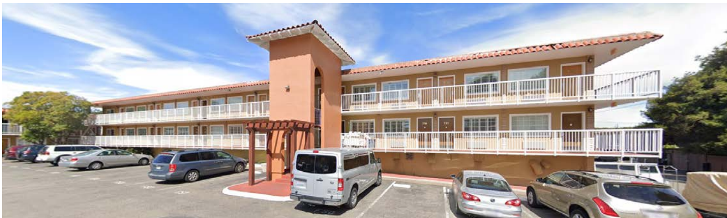
Photo 9. View of Building 700 facing west. Source: Google Earth 2019.
