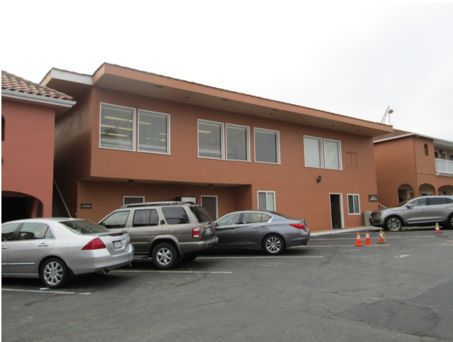
3. View of Building 3 from the northeast
