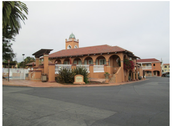
4. View of Building 4 from the south
