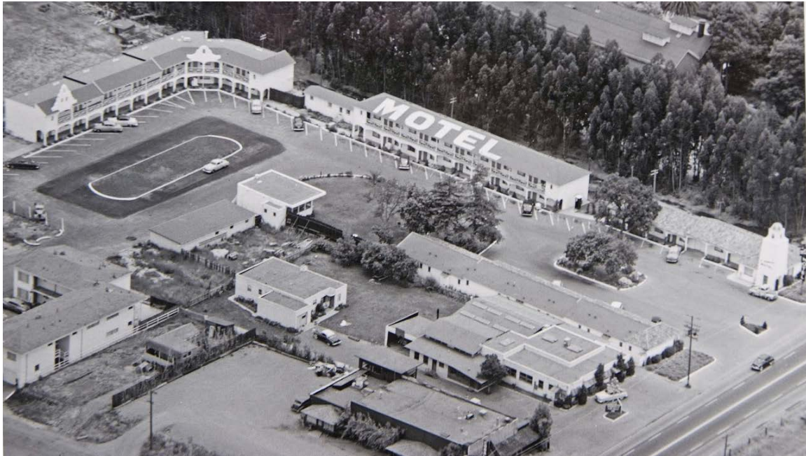
Figure 6. Photo of the El Rancho Motel ca. 1954. By this time, Building 200 was partially extant and the now-demolished “15 Units” building was present at the western edge of the site. Source: Dawdy 2020.
