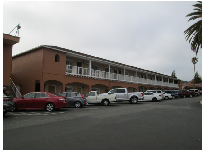
2. View of Building 2 from the northeast
