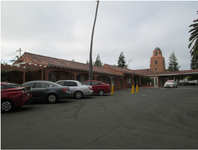
1. View of Building 1 from the northeast
