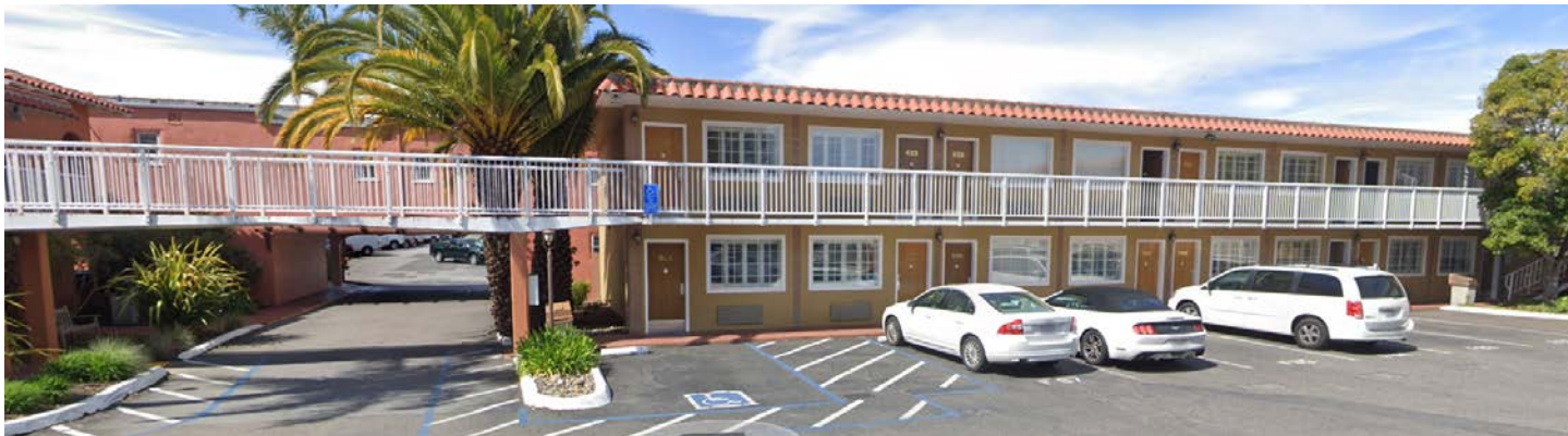
Photo 8. View of Building 600 facing southwest. Note the cut-through of Building 200 that provides vehicular access to the northern end of the complex. Source: Google Earth 2019.
