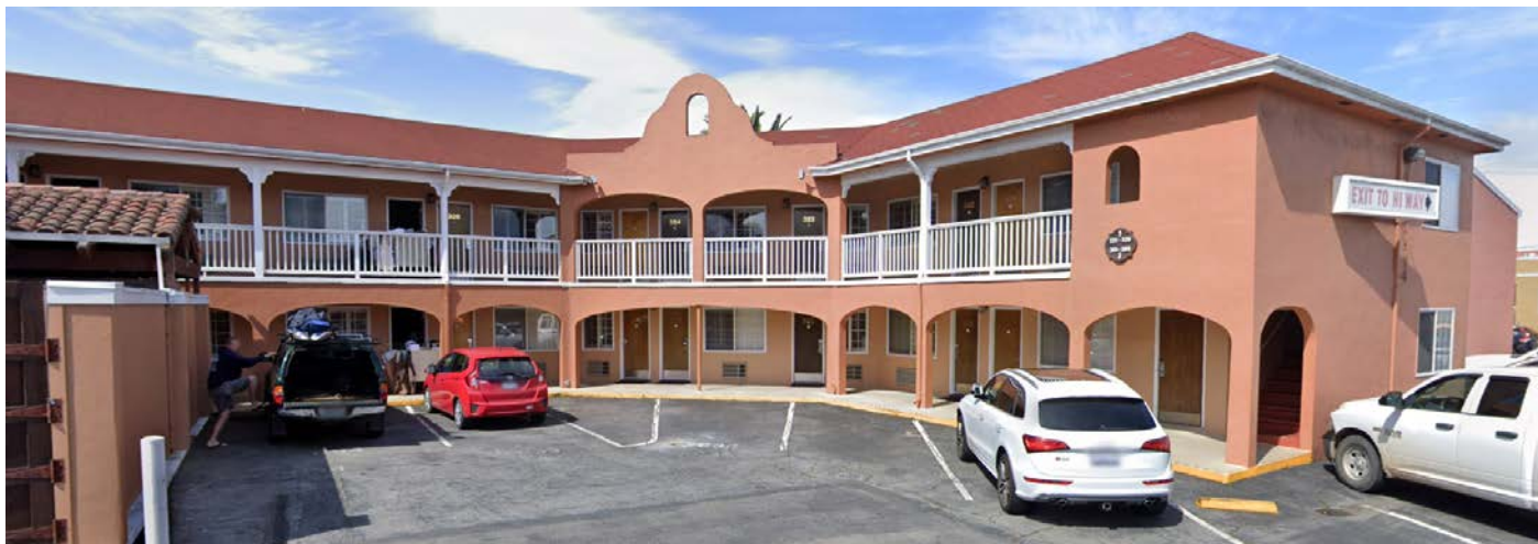
Photo 6. View of Building 300 facing southwest. Source: Google Earth 2019.
