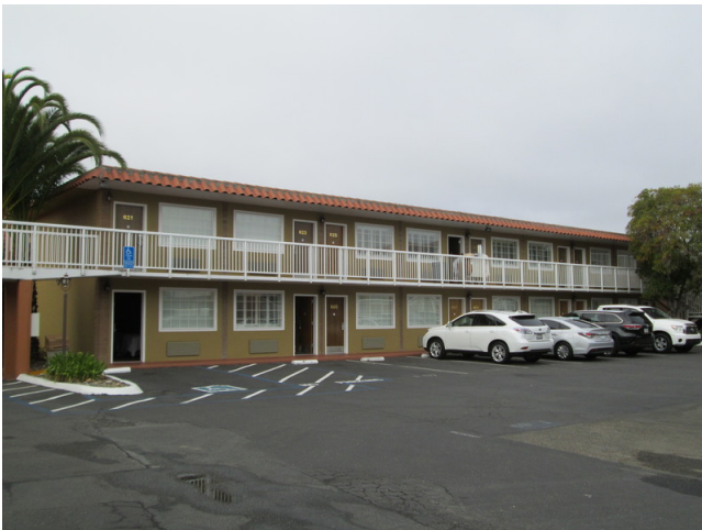
7. View of Building 7 from the east
