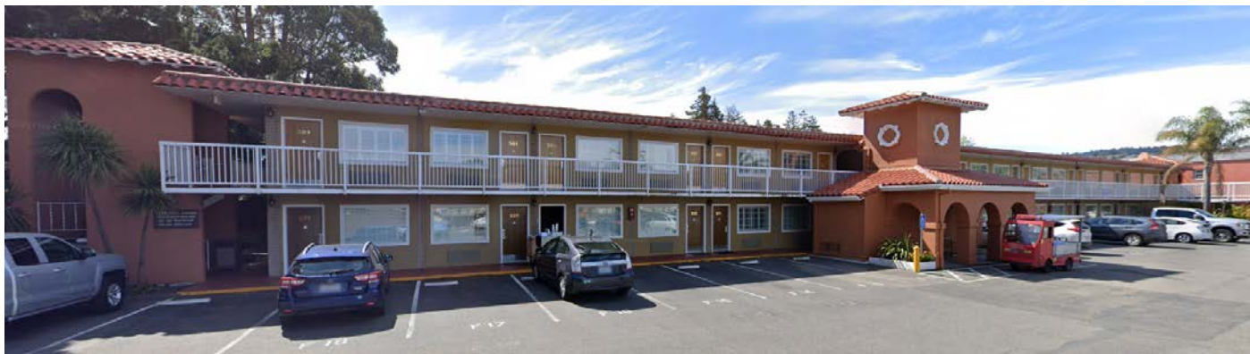
Photo 7. View of Building 500 facing south. Source: Google Earth 2019.
