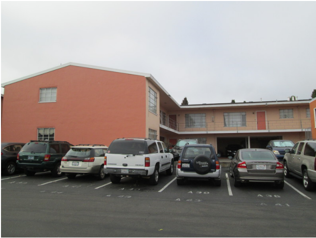
9. View of Building 9 from the east
