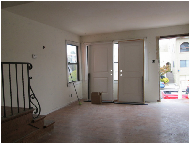
25. View of the interior of Building 10
