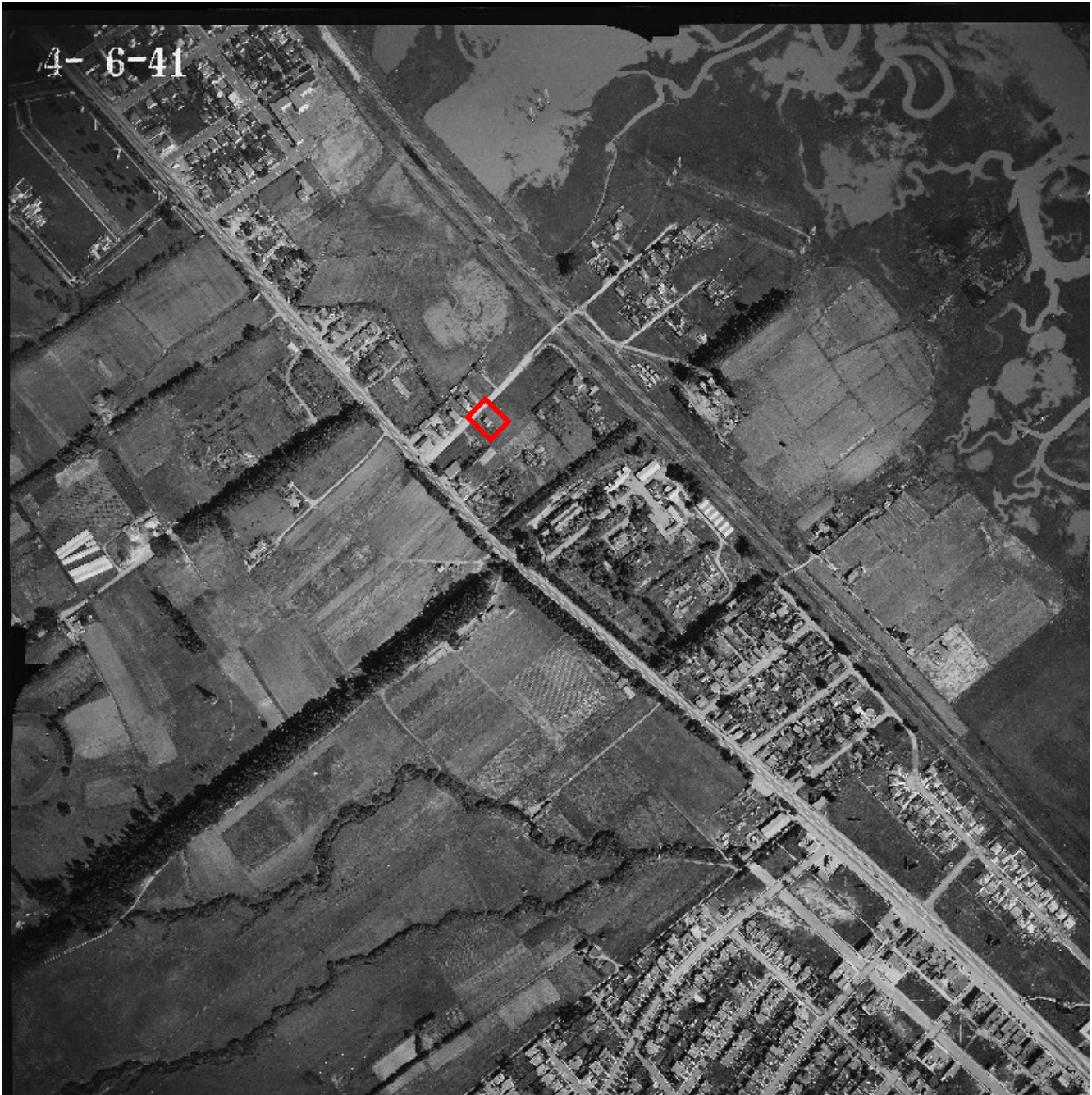
Figure 1. 1941 Historic aerial photograph of the 33 and 35 Center Street parcel as the surrounding area is scattered residential development. 35 Center Street is constructed, but 33 Center Street is not yet built. Source: UCSB and ESRI 2021.
