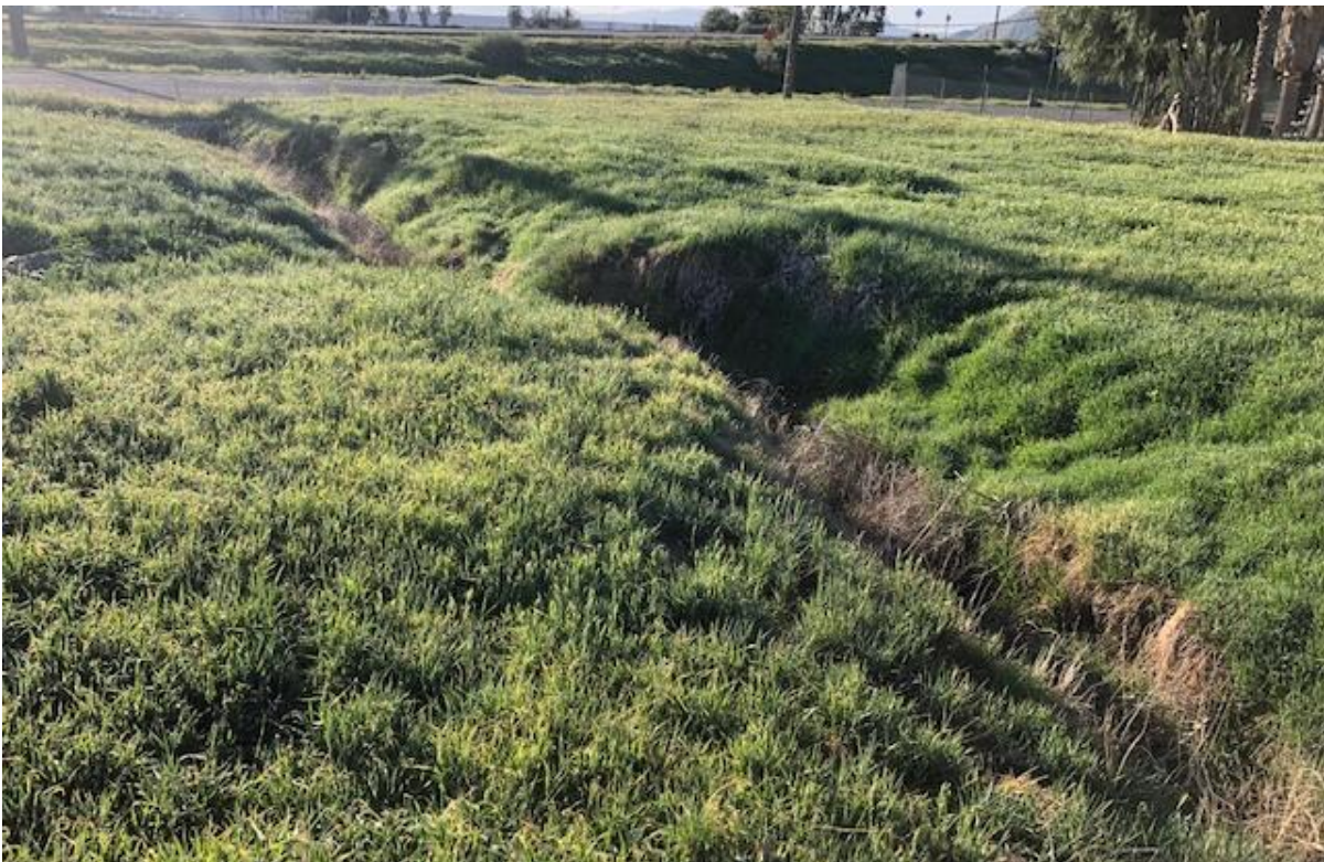
Photograph 6. Downstream, southeast-facing view of erosional feature toward Spruce Ave.
