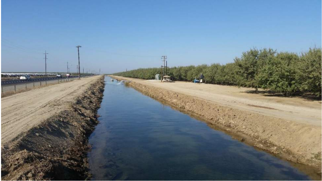
Photo 5. Well 88-25-010, on right in background (facing west).
