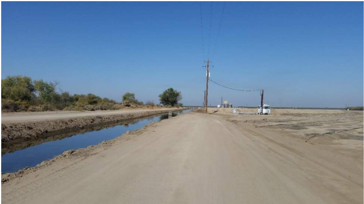
Photo 2. Proposed pipeline route to well 88-29-035 (facing northwest with 8-29 Canal on the left and well 88-29-035 on the right in background).
