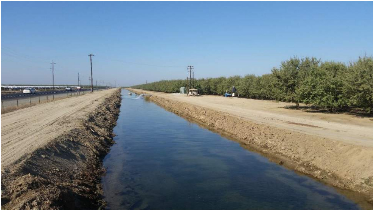
Photo 7: Well 88-25-010, on right in background (facing west).
