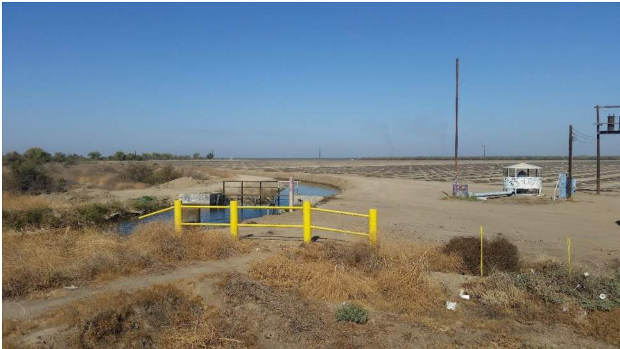
Photo 3: Proposed pipeline route to well 88-29-035 (facing northwest from Friant-Kern Canal tie-in location, with 8-29 Canal on the left).
