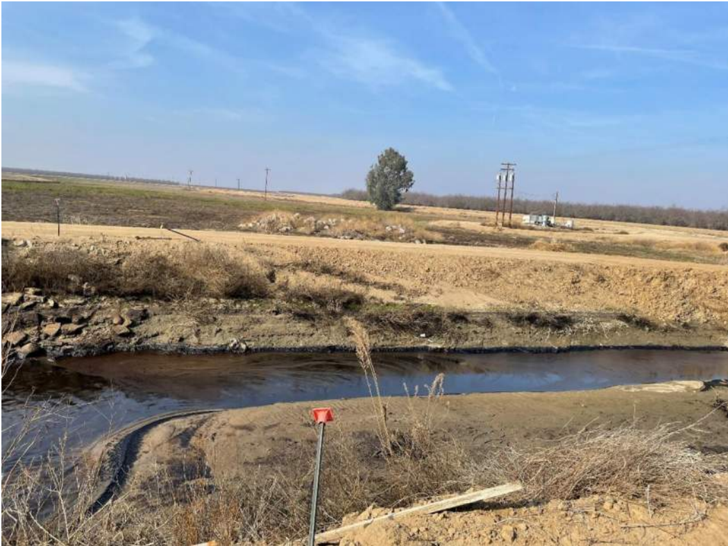
Photo 2: Calloway Canal adjacent to Rosedale spreading basin, east facing west (April 2021).
