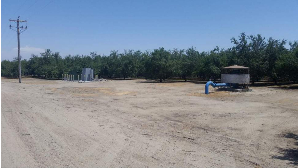
Photo 7. Well 88-17-036 (facing southwest).
