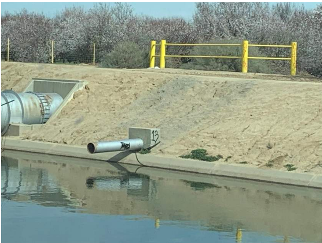
Photo 12. An example of a standard turn-in and small delivery gate (center) at Friant-Kern Canal.
