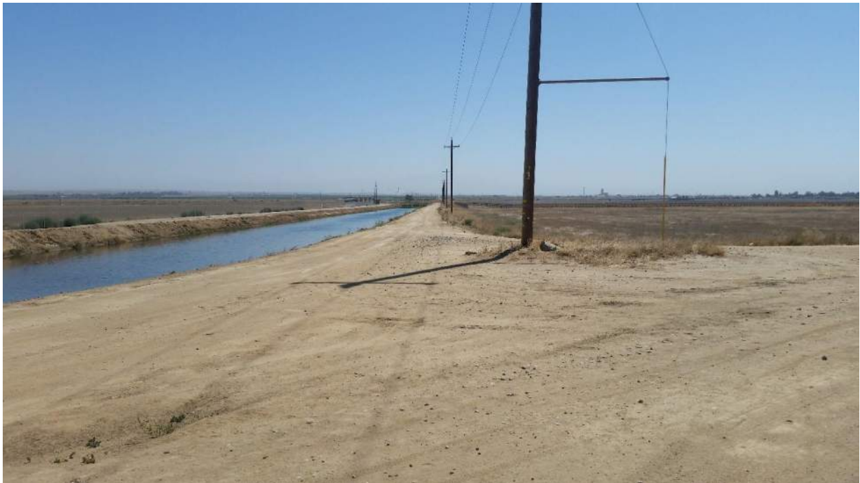
Photo 10. Proposed pipeline route between Calloway Canal and Friant-Kern Canal (facing east).
