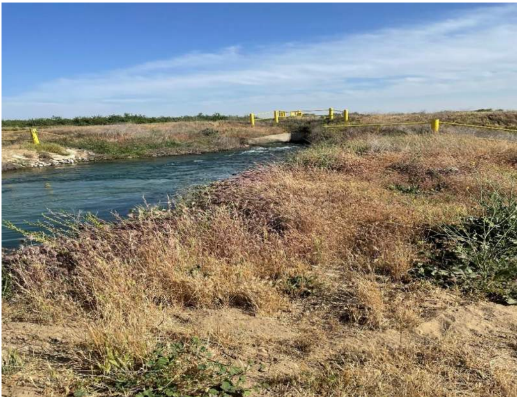
Photo 12: Canal adjacent to well 88-05-003 (April 2021).
