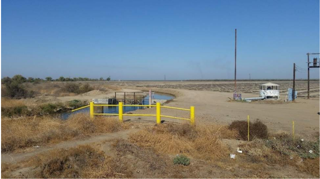
Photo 1. Proposed pipeline route to well 88-29-035 (facing northwest from Friant-Kern Canal tie-in location, with 8-29 Canal on the left).
