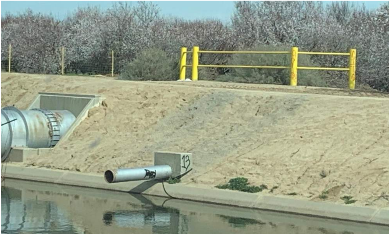
Photo 10: An example of a standard turn-in and small delivery gate (center) at Friant-Kern Canal.
