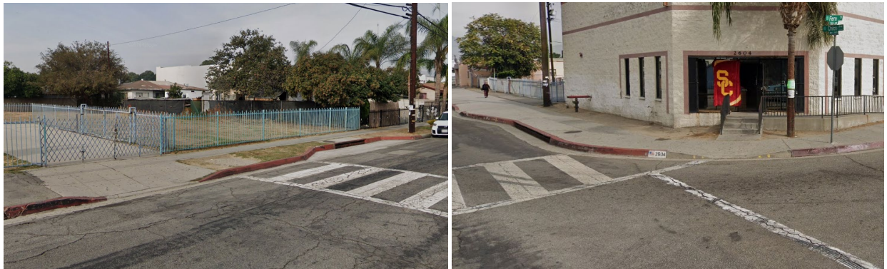
Current misaligned curb ramp configurations for crosswalk at Chico Avenue/Fern Street intersection.
