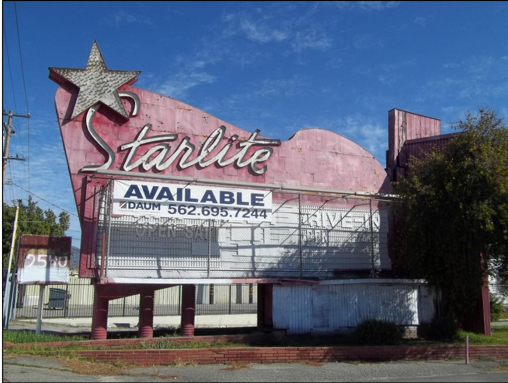
E-1. Starlite Drive-In theater sign, facing north
