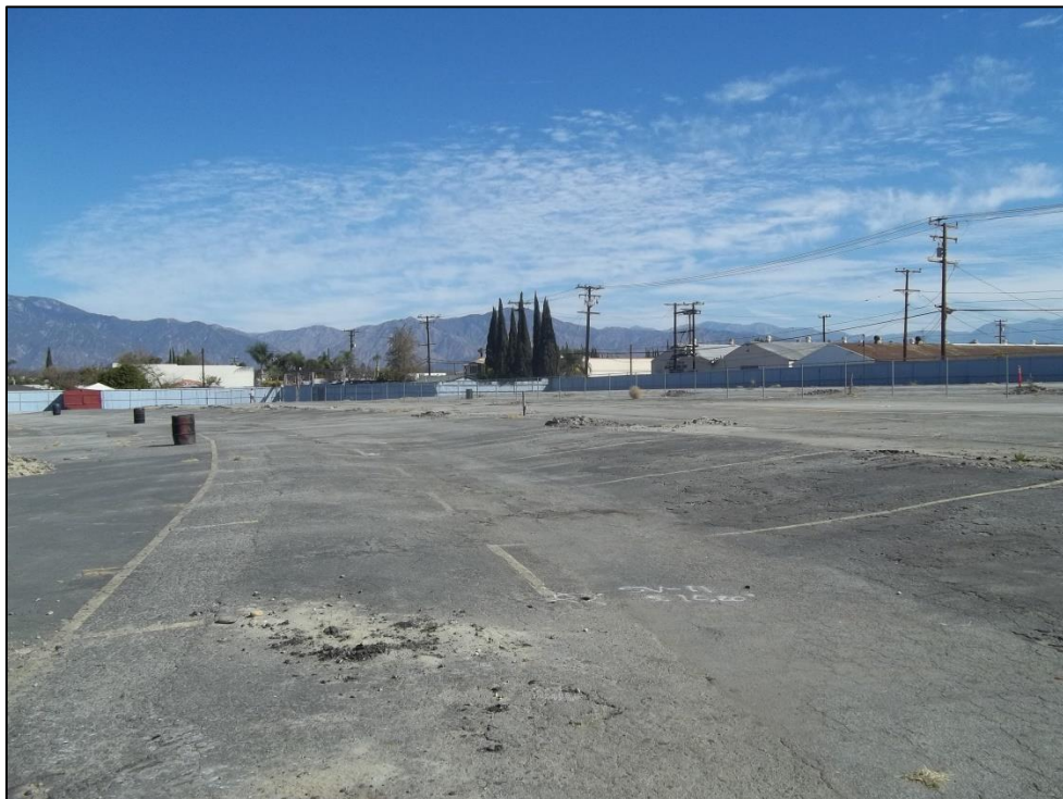
9. Overview of eastern section of parking area, facing north
