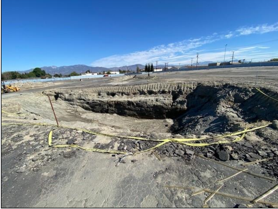
Figure 15. Excavated trench, facing north
