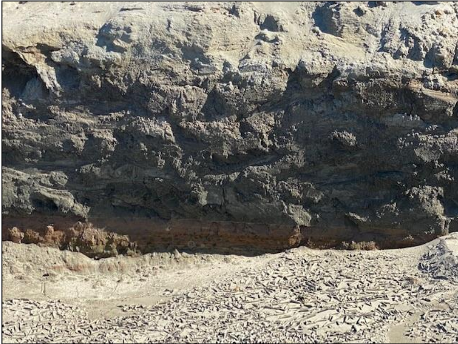
Figure 16. Stratigraphy of north wall, facing north
