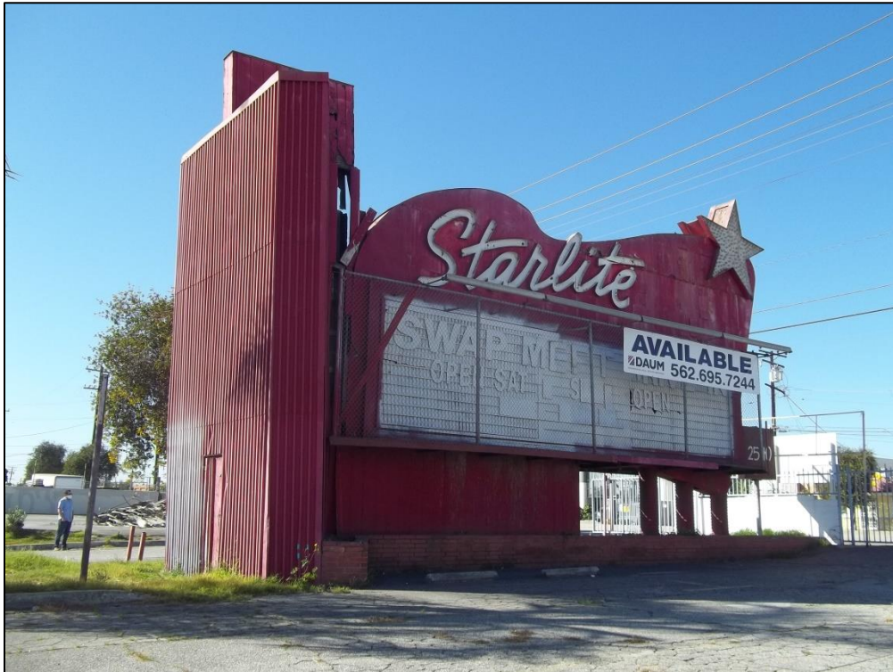
E-2. Starlite Drive-In theater sign, facing southwest
