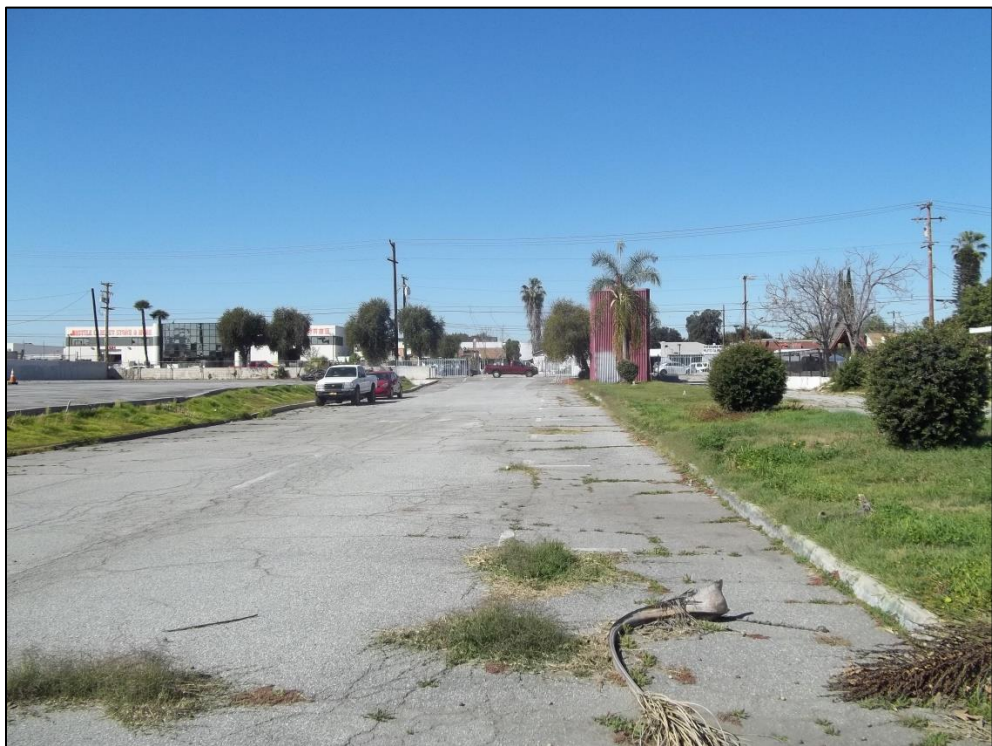
4. Main entrance driveway, facing west towards Rosemead Blvd.
