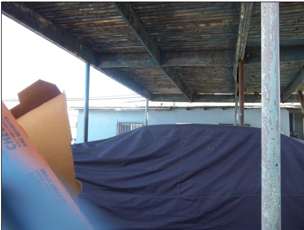
Wood framed shelter and west elevation of residence.
