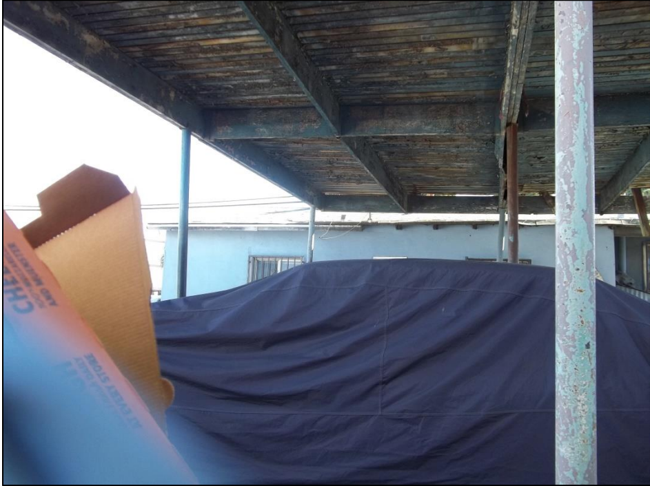
E-14. Partial west elevation and wooden carport
