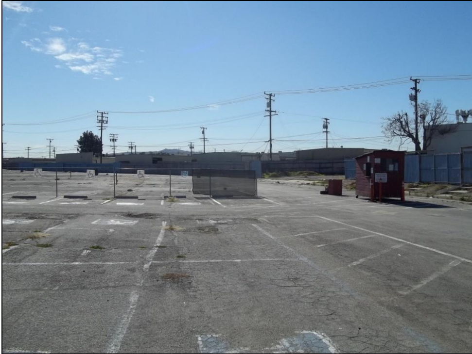
E-8. Overview of southwest segment of parking area
