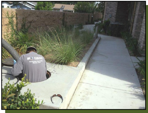
Vacuuming out of media filters.
