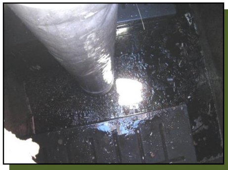
Removal of trash, sediment and debris.
