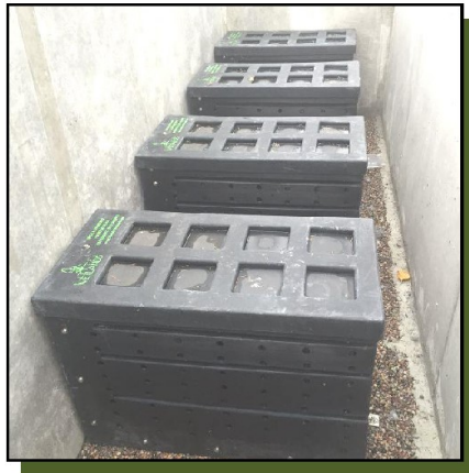
Pre-filter cartridges with tops on.
