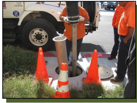
Insertion of vacuum hose into separation chamber.
