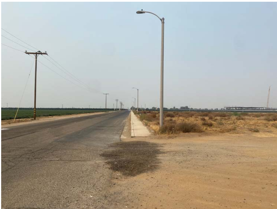
Photo B-8: Photograph of proposed stormwater drain pipe route along West Street facing north (August 19, 2021)
