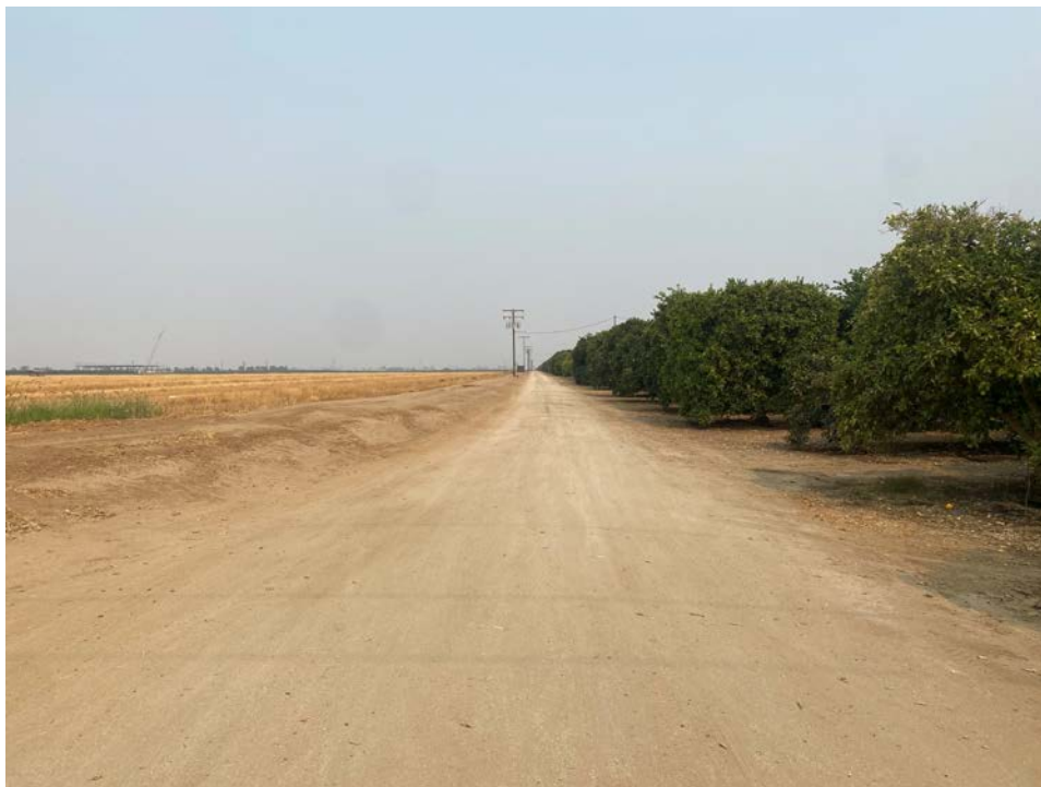
Photo B-6: Photograph of proposed stormwater drain pipe route from Road 216 facing east (August 19, 2021)
